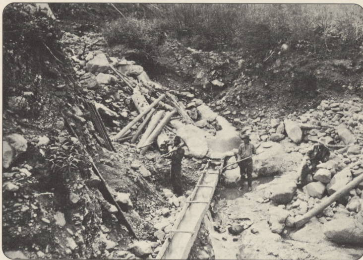
Long, wooden troughs or sluices used in large-scale placer operations diverted stream flow to wash sand free of gold particles.
