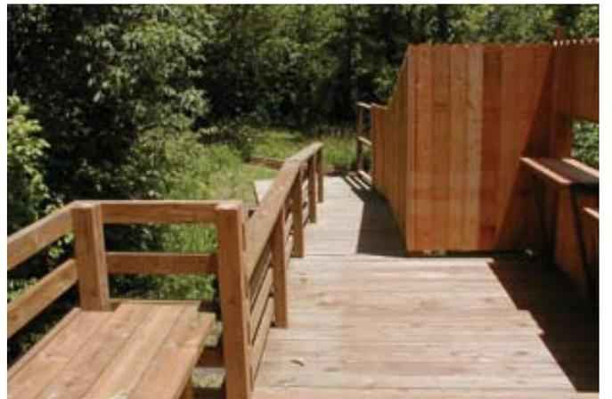
**June 15** The fence along the upper portion of the ramp slopes upward from under five feet to the full height of the fence on the decks.
