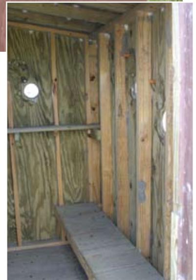
**Materials:** Treated 2x4's and plywood, with painted exterior.
