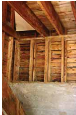
Figure 32: Floor Joist Support at Back
