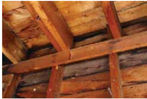
Figure 31: Floor Joist Support at Front
