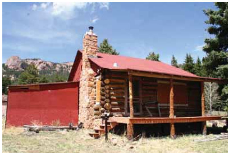
Figure 24: Exterior View of Large Cabin
