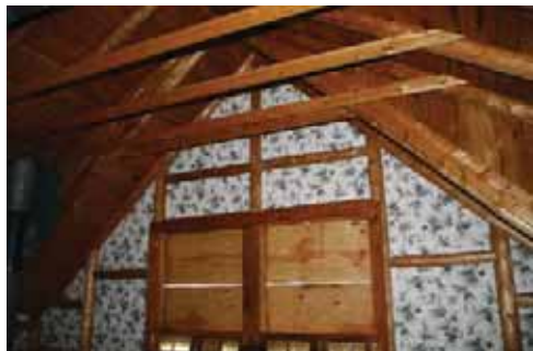
Figure 20: Roof and Gable End Wall Framing
