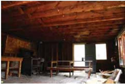
Figure 30: First Level with Upper Floor Framing
