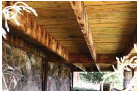
Figure 25: Porch Floor Framing
