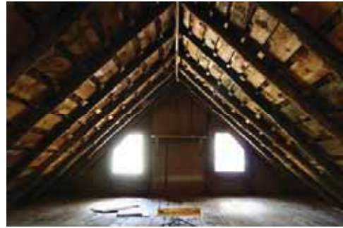
Figure 16: Roof Framing at Ridge
