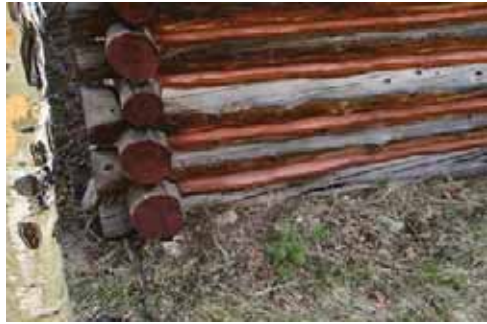
Figure 10: Corner Joint
