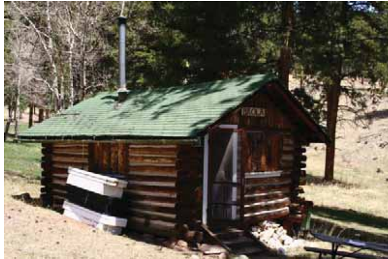
Figure 17: Exterior View of Brola Cabin
