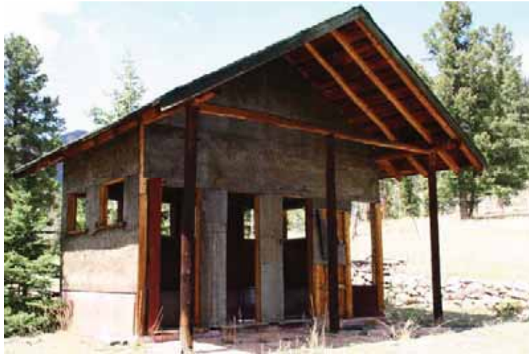
Figure 22: Exterior View of Bath House
