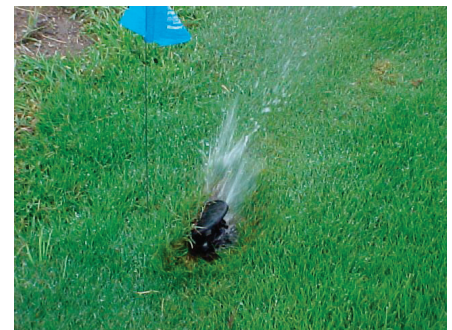
Figure 8: This sprinkler head is not parallel to the slope.
