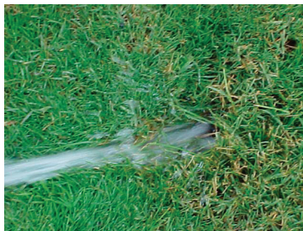
Figure 6: Water deflected due to the sprinkler head being too deep.
