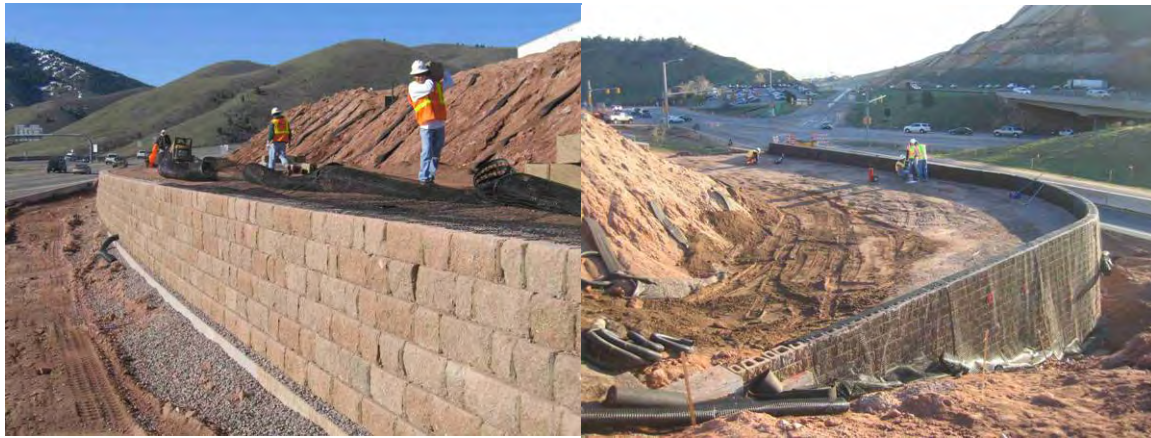
Figure 3-1. SH40 – I70 Hogback MSE Wall
