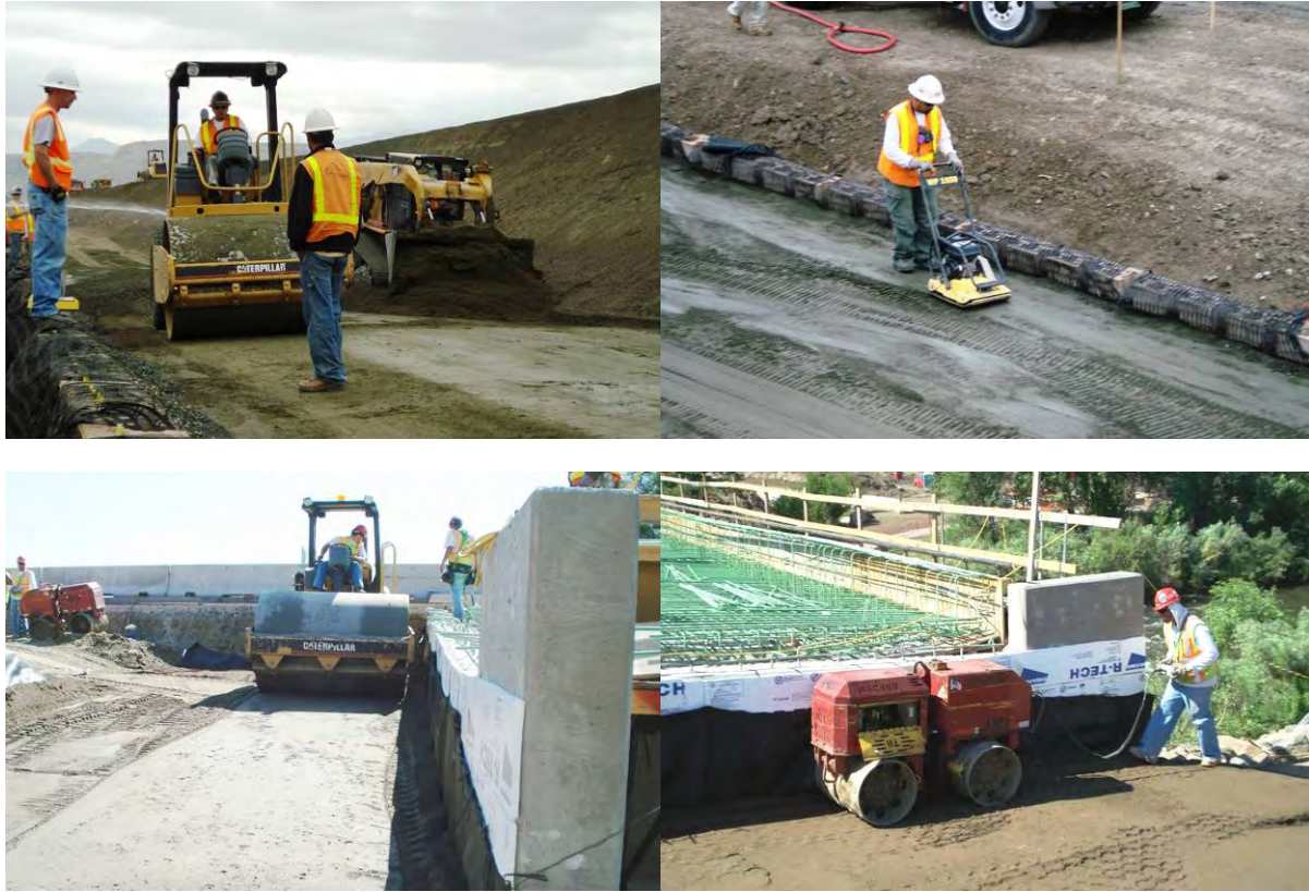
Figure 4-6. Near Wall Compaction Techniques
