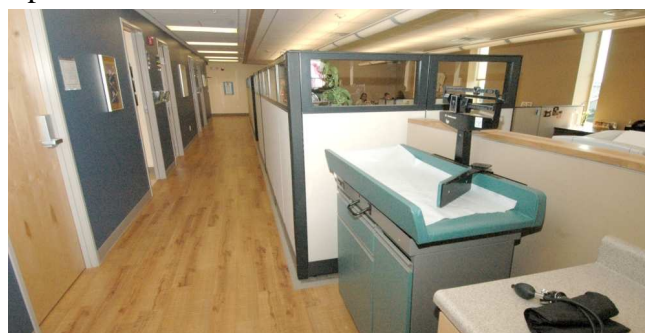
Clinica Campesina completed the renovation of the second floor of its Pecos Street clinic.
