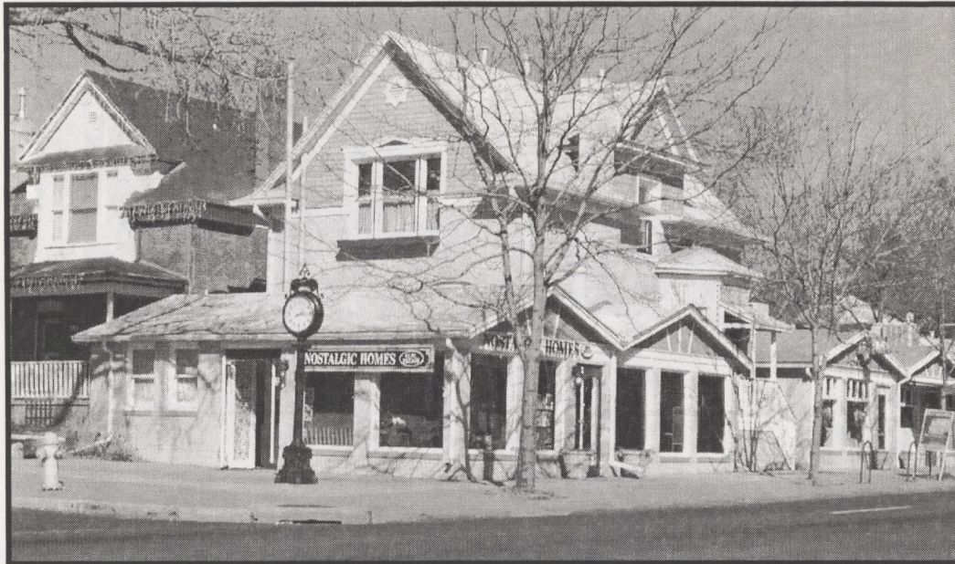
A corner commercial addition wraps around a Victorian-era house on East 6 th Avenue in Denver
