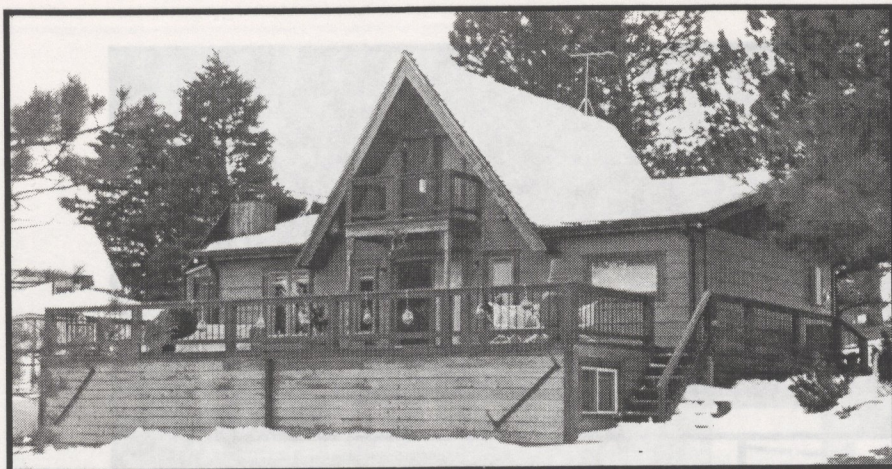
Though not a true A-Frame, this house in Louviers combines the basic form with gable-roofed side wings.
