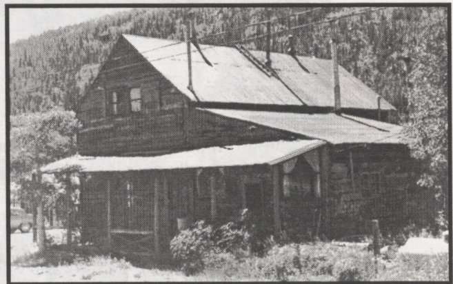
Mill waste, slab walls, front gable cabin in the Eldora Historic District, Boulder County
