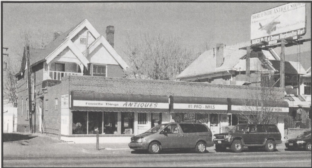
A triple-storefront addition of mid-twentieth century vintage fills multiple lots in front of a Queen Anne style house
