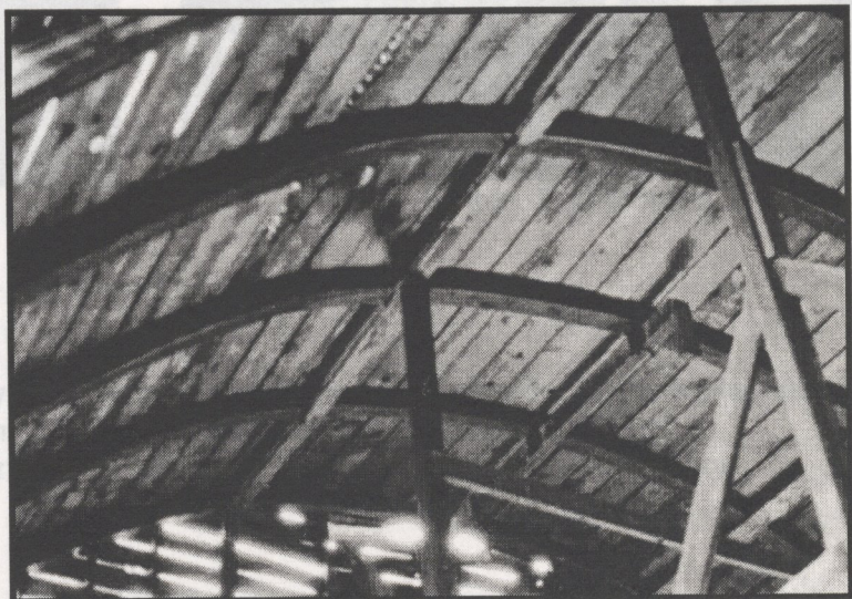
Interior Rafters of a Round-Roof Barn
