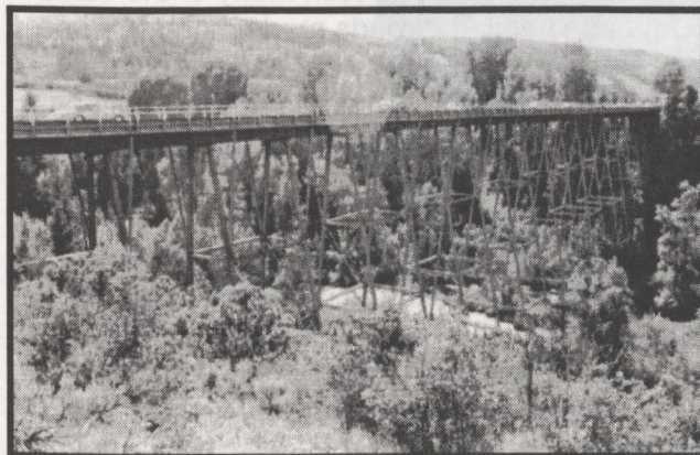
Steel Stringer, Aspen
