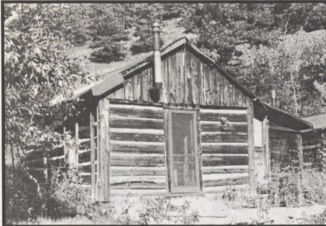
Hewn logs, boxed corners, front gable, and board and batten gable in Boulder County
