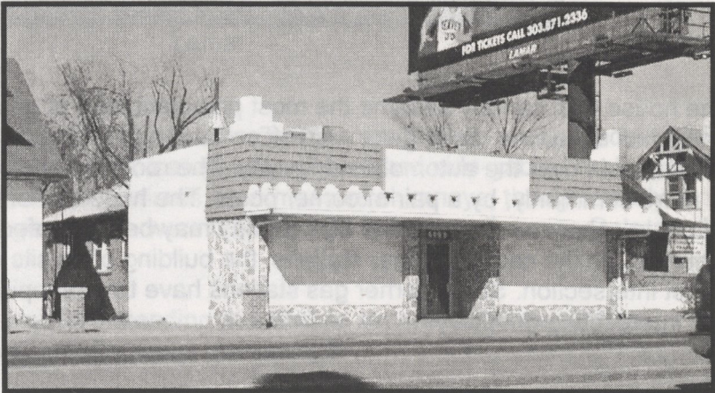
An E. Colfax restaurant addition in Denver almost completely hides the original house
