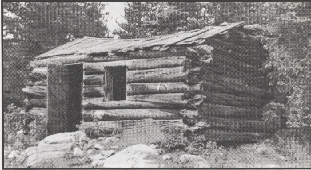
Round log, saddle-notched, side-gabled cabin in Boulder County
