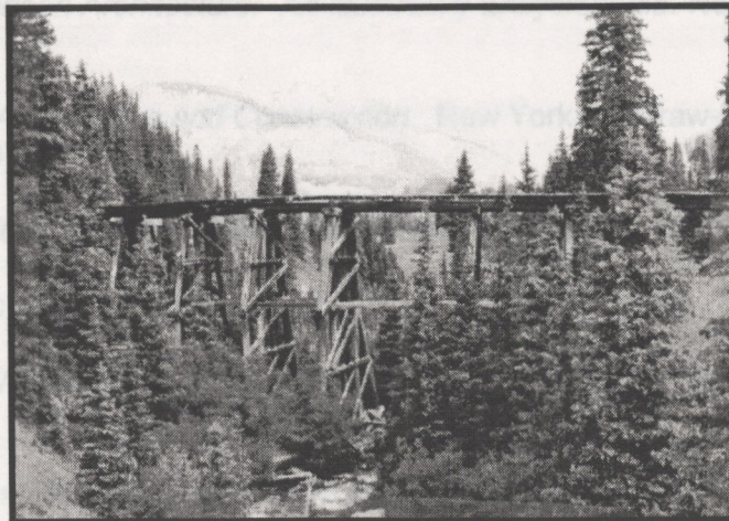
Railroad Timber Stringer Trestle in San Miguel County
