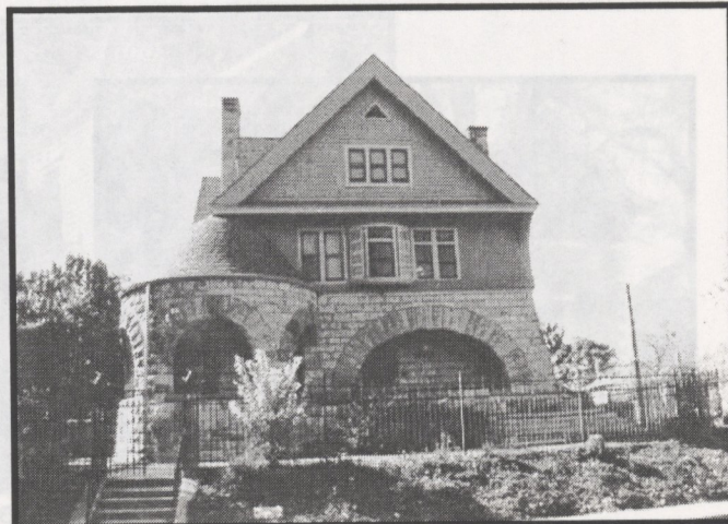
The Gates Mansion in Denver combines the Shingle style with Richardsonian Romanesque.
