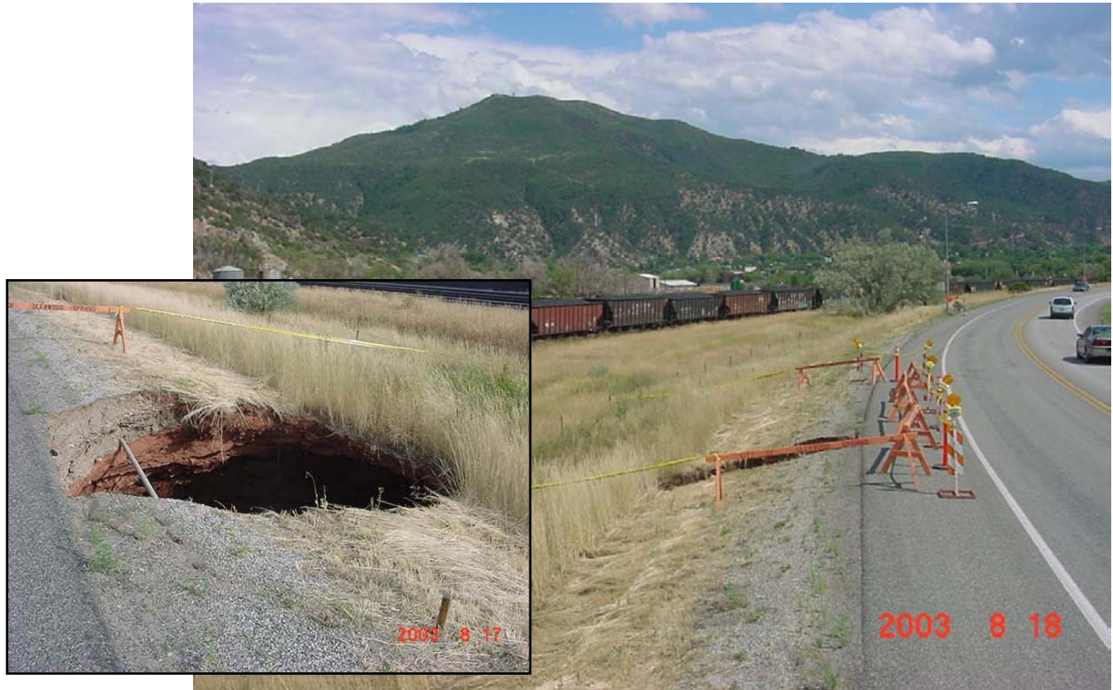
Figure 9. Sinkhole opening in 2003 along new bypass of Midland Avenue in West Glenwood Springs. View is to the east towards downtown Glenwood Springs and Lookout Mountain. Chalky white slopes exposed along valley wall is the Eagle Valley Evaporite. Photo courtesy of Larry Thompson, City of Glenwood Springs.
