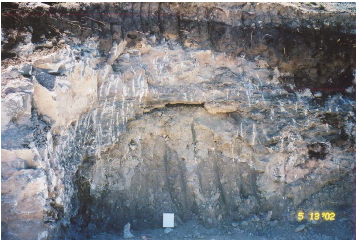
Figure 11. Residential foundation excavation in Eagle County has exposed a near-surface cavern in gypsum that is almost completely infilled with fine-grained sediment. Topsoil is at top of photo and original ground surface shown in upper right corner. Field notebook is shown for scale. Photo courtesy of Steve Pawlak (HP Geotech).
