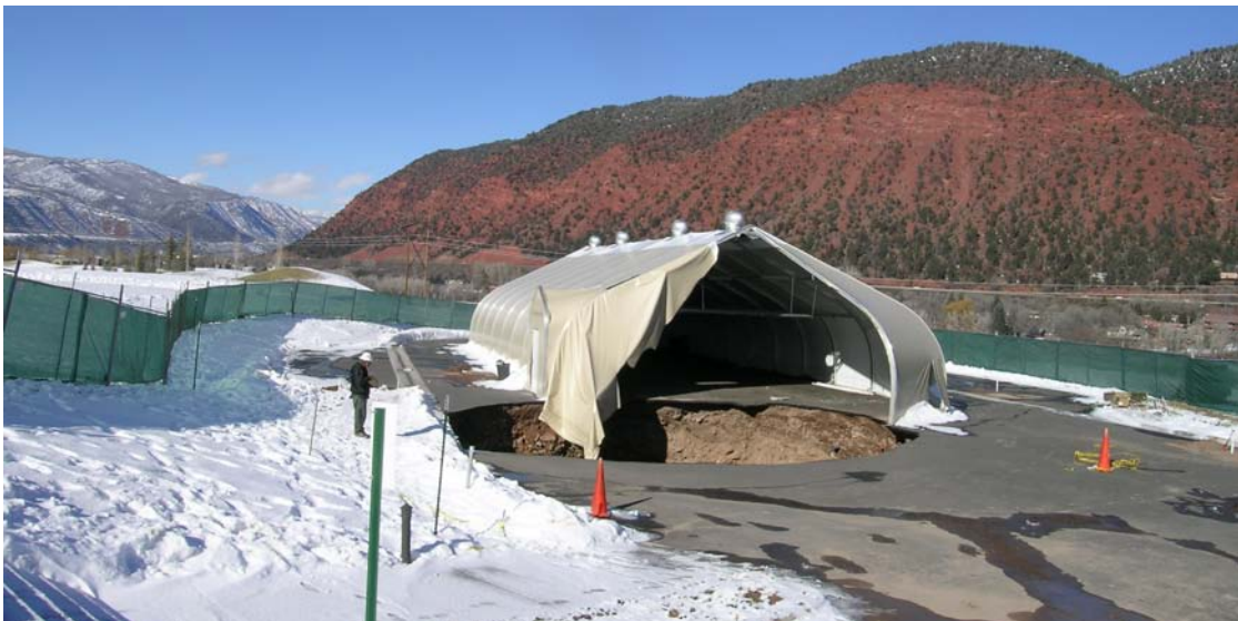
Figure 10. Large sinkhole opened in 2005 at golf course club grounds at Ironbridge Development. Two golf carts inside the structure were lost down the throat of the sinkhole. View is to the northwest, down the Roaring Fork River valley towards Glenwood Springs. Red cliffs are the Maroon Formation. For scale, note person in white hardhat standing in the snow.
