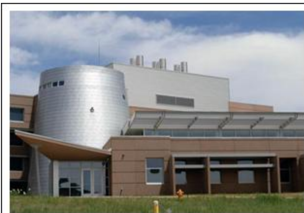
NREL Science & Technology Facility, Courtesy of NREL, Credit— Marjorie Schott
