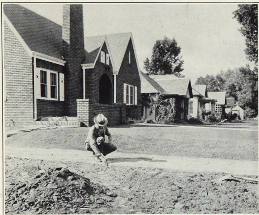
Figure 1.—A well-graded surface is most desirable for starting the new lawn; note the depth of excavation for filling in with good top soil.
