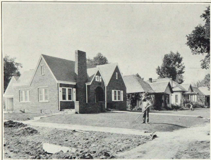
Figure 2.—Gradual drainage away from the house is preferable to flat lawn; note fineness of pulverization in seedbed.
