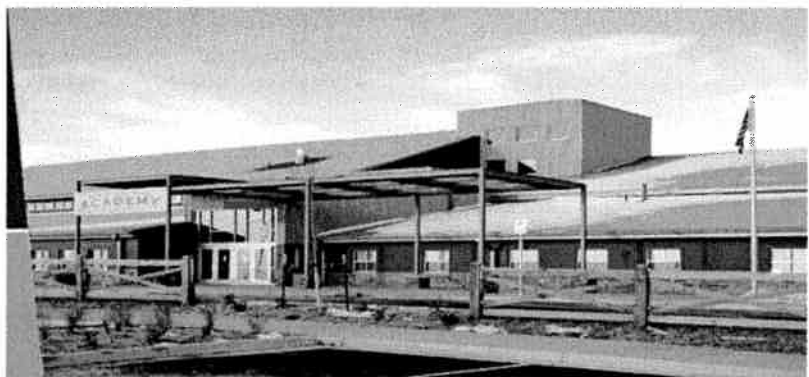
Banning Lewis Ranch Academy, K-8 Colorado Springs
