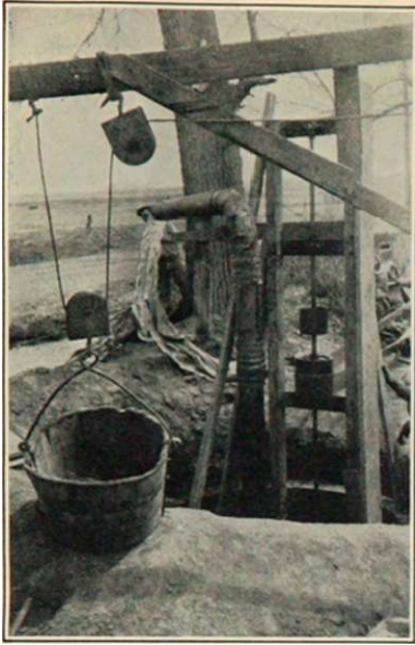
Fig. 4.—Sinking-pump equipment for large shallow wells in use.
