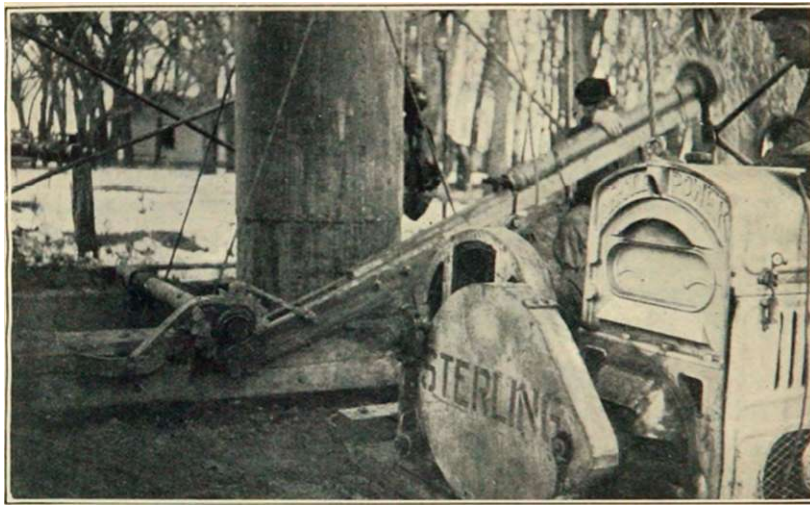
Fig. 19.—Jacking arrangement for forcing casing.
