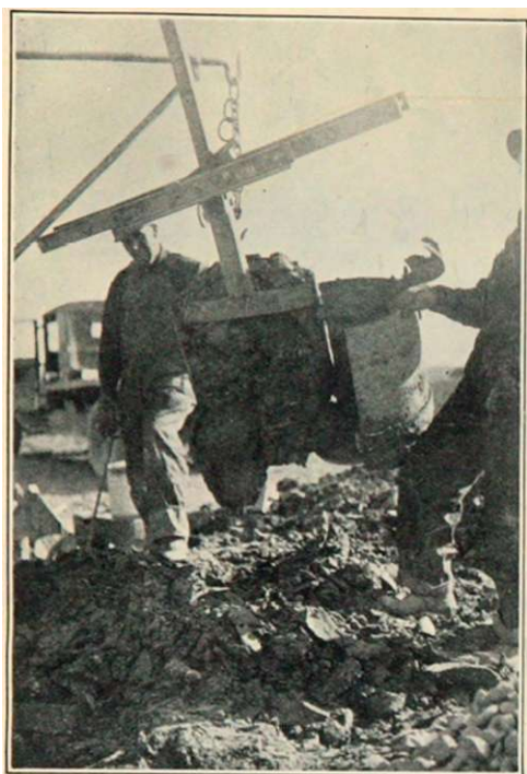
Fig. 9. —Engine-driven soil auger. Side opening bucket with reamer attached.
