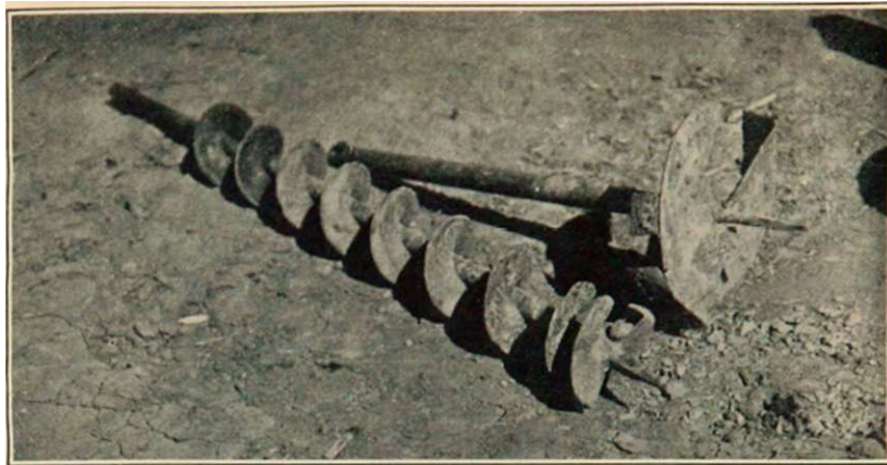
Fig. 8a.—Soil auger operated by hand.
