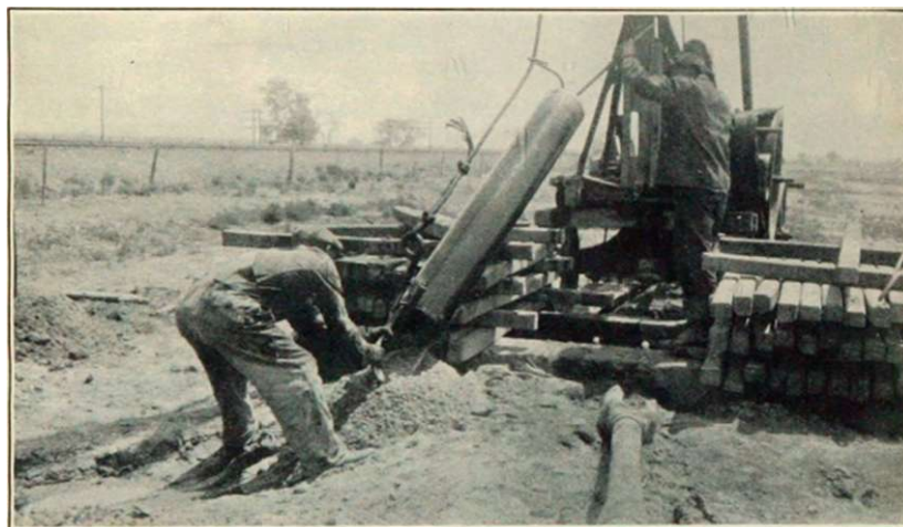
Fig. 12.—Dumping a churn bucket. Steel billets being used to load casing.
