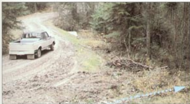
One of the most common road drainage problems is allowing ditch drainage to flow directly into a stream. Always route ditch drainage into a filter (SMZ, slash filter windrow, etc.) so sediment can be removed before water reaches the stream.
