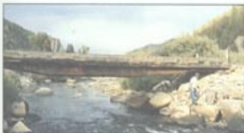
Railroad flatcars can provide a low cost alternative to conventional bridge construction.
