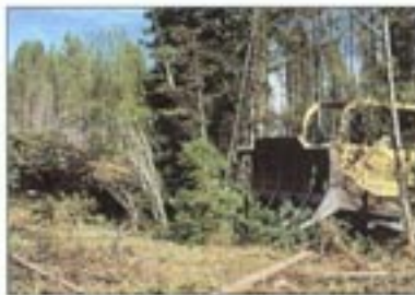
Work around existing small trees and low brush.
