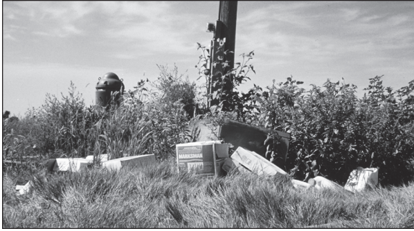
This wellhead is in serious need of a clean-up.
