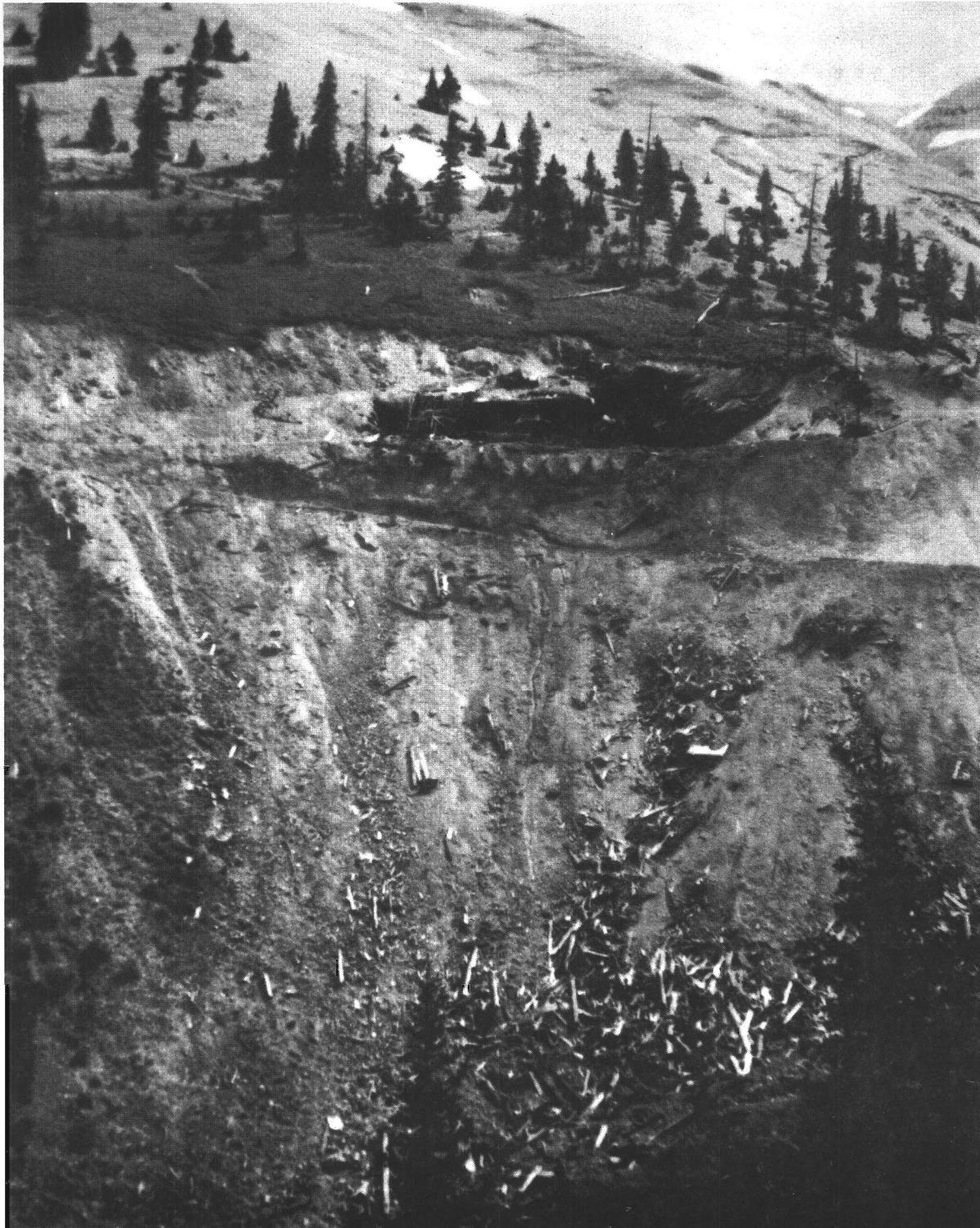
Figure 10. Location of the Gold King Mine boarding house, 1975. (R. Armstrong photo)
