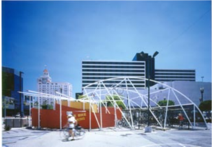
Figure 4-3. Long Beach Bikestation. This project in Long Beach, California is seen as a model for similar endeavors nationwide..
