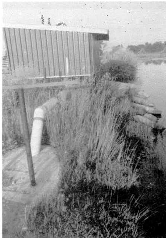
Well pump and house
