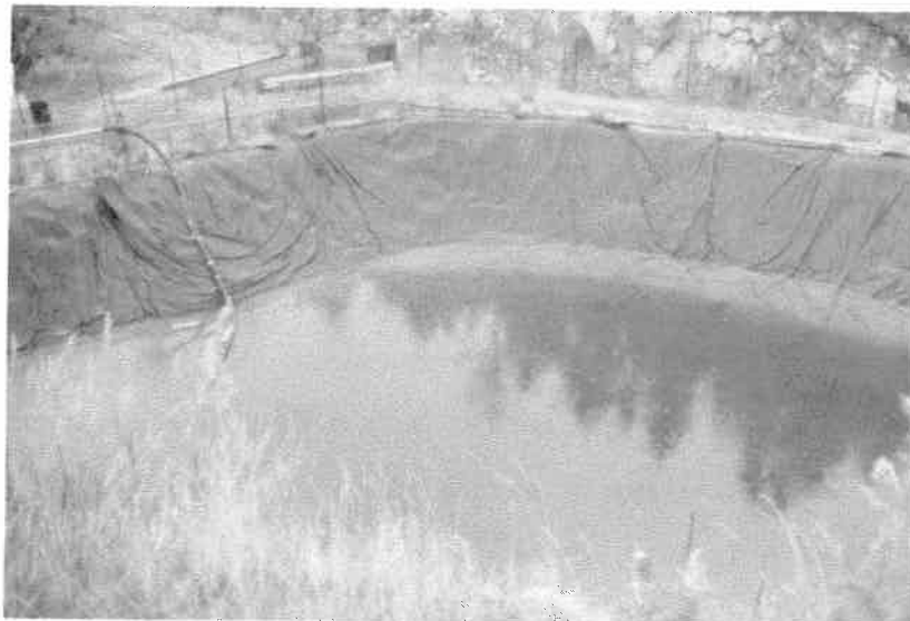
Plastic lined tailings pond
