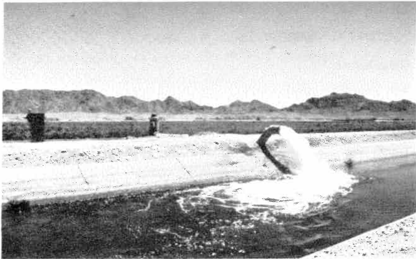
Pumping water into canal
