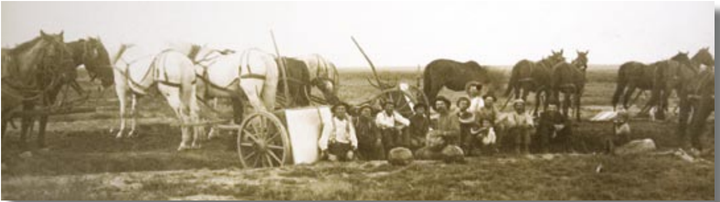
Workers take a break from digging a ditch near the Pleasant Valley School in Greeley. Most early settlers possessed no experience or equipment for building irrigation canals, and ended up using their own teams, plows, pick-axes and shovels.
