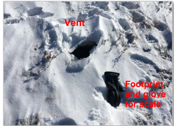
Figure 4-2 – Lewis Mine Fire Vent
