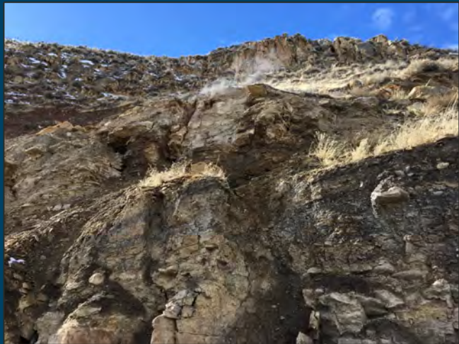
Vents in east-facing outcrop
