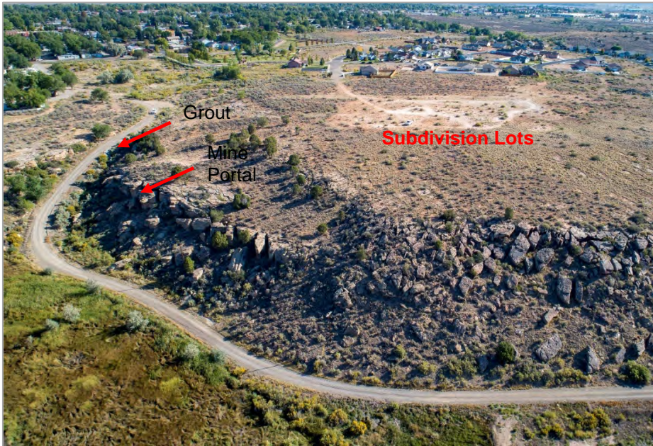
Figure 4-104 – McElmo Mine Fire Looking North
