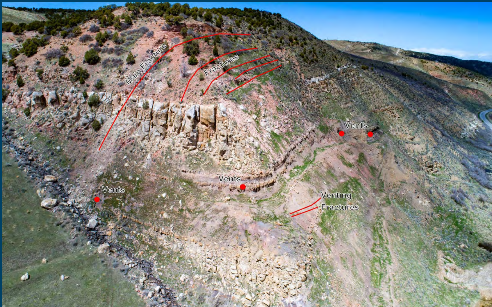
Axial Mine fire looking Northwest
