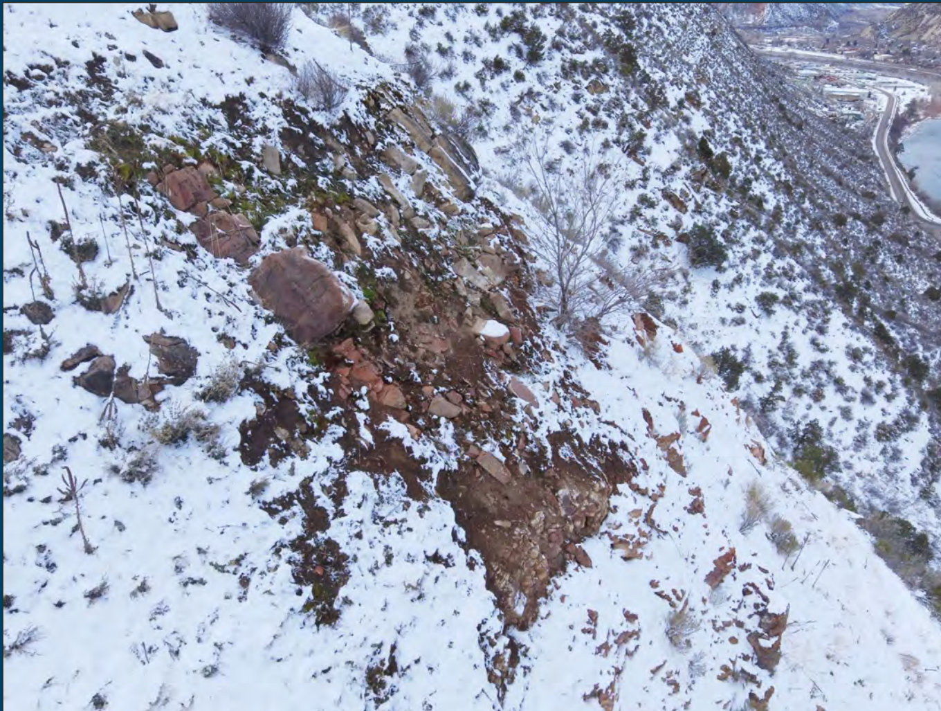
Fire expression looking West
