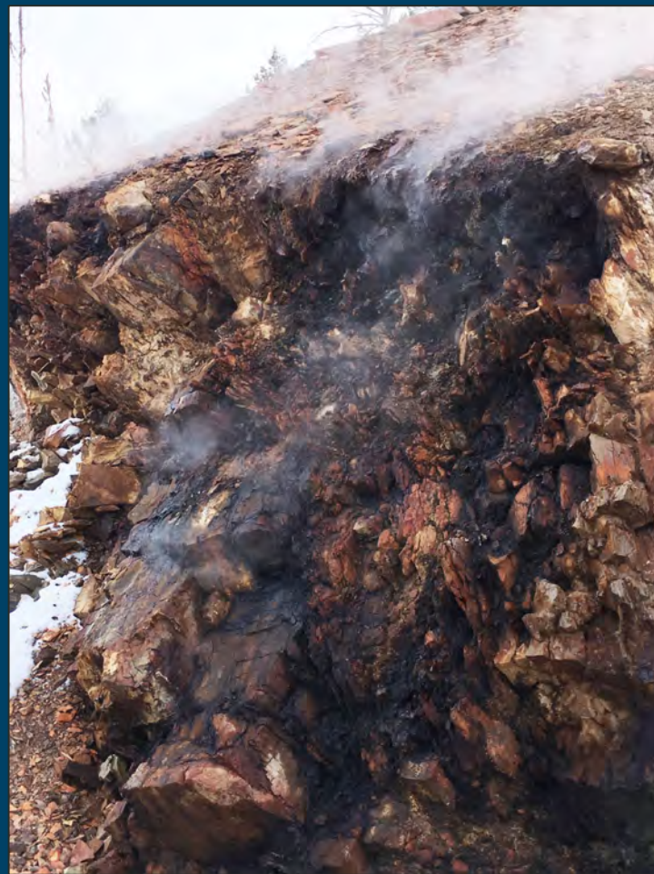
Upper road cut vents with creosote
