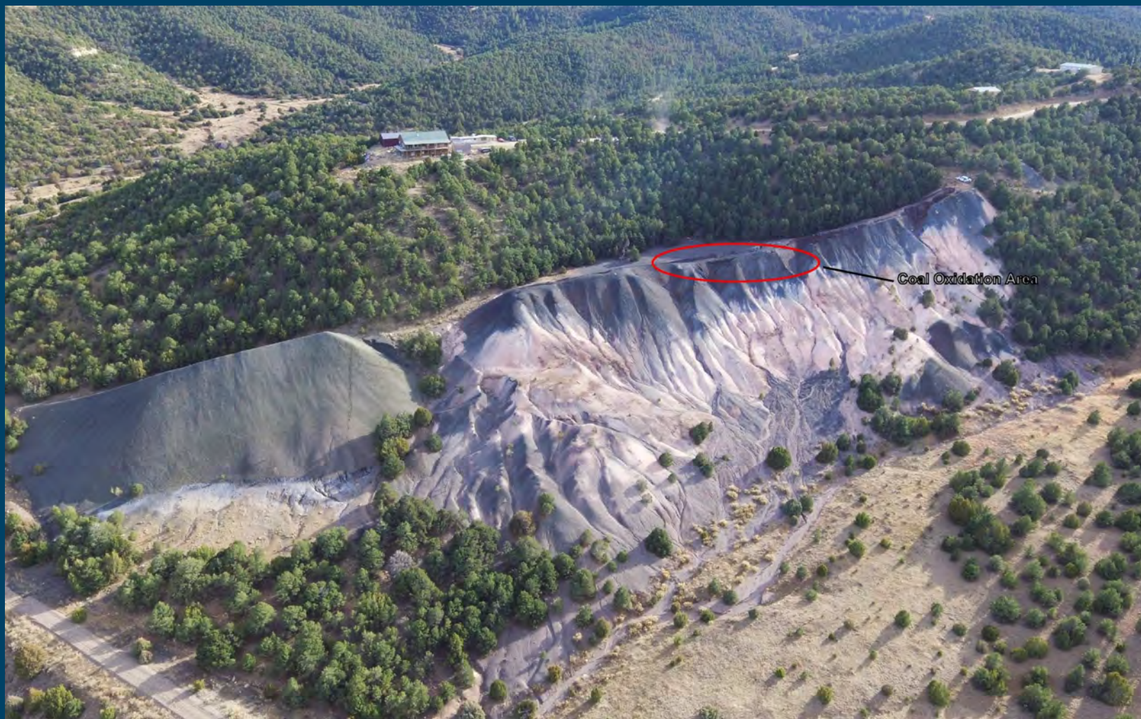
West Sopris coal refuse pile fire looking Southeast
