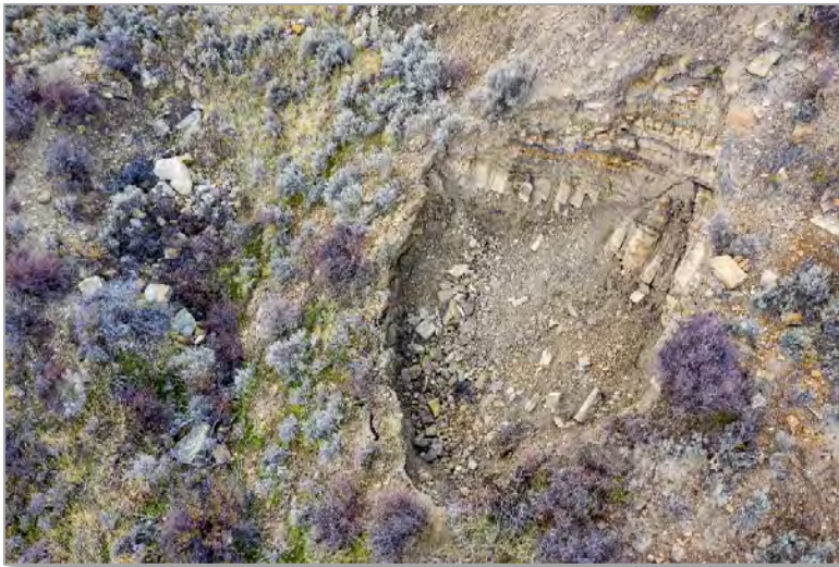
Figure 4-65 – Large Subsidence Feature
