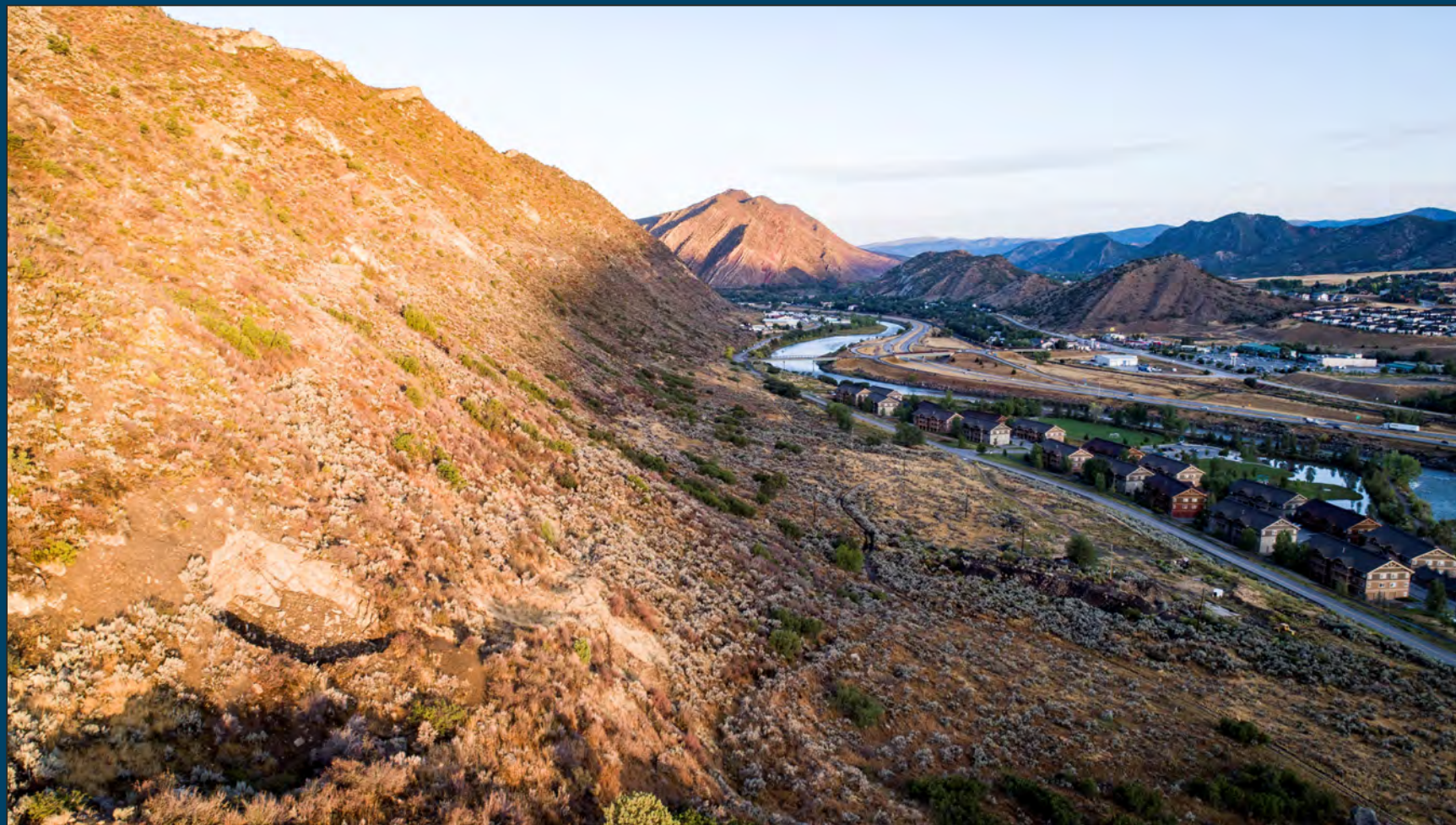
45 ft diameter subsidence feature looking West
