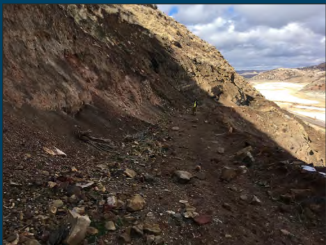
Looking North below vents
