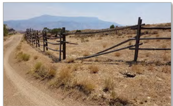
Figure 4-93 – Fence Damage and Subsidence
