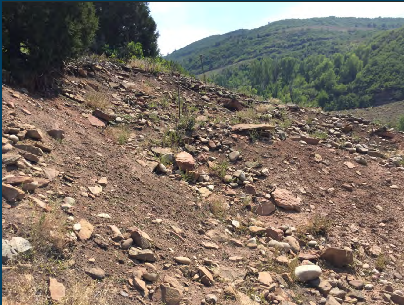
Subsidence area over adit with monitoring monuments
