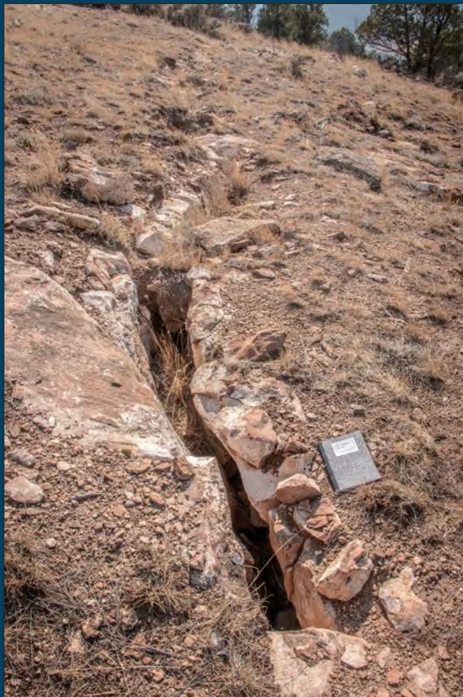
Large fracture, no venting
