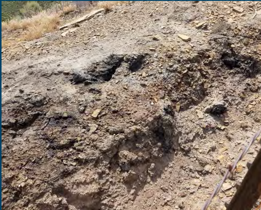
Venting South of smoking subsidence feature
