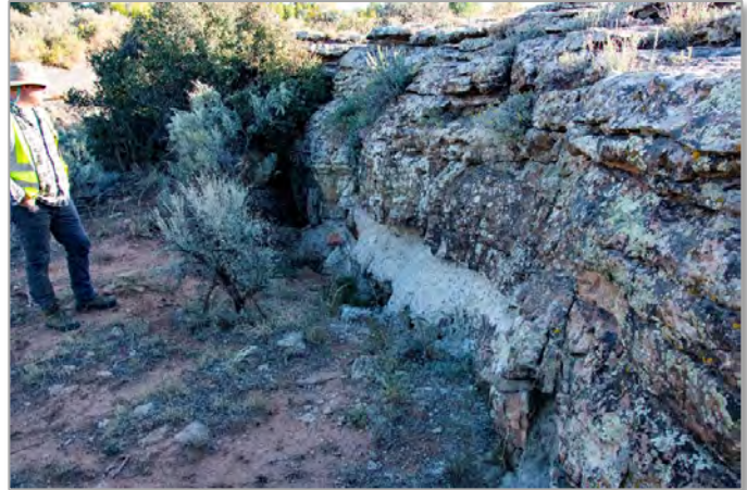
Figure 4-106 – Grout Seal in Sandstone Outcrop
