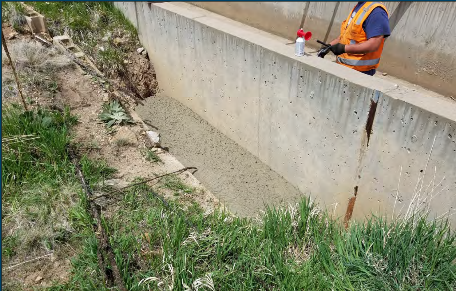
Flow fill of two voids under aqueduct May 7, 2018
