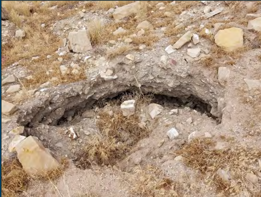
6 ft by 5 ft subsidence feature
