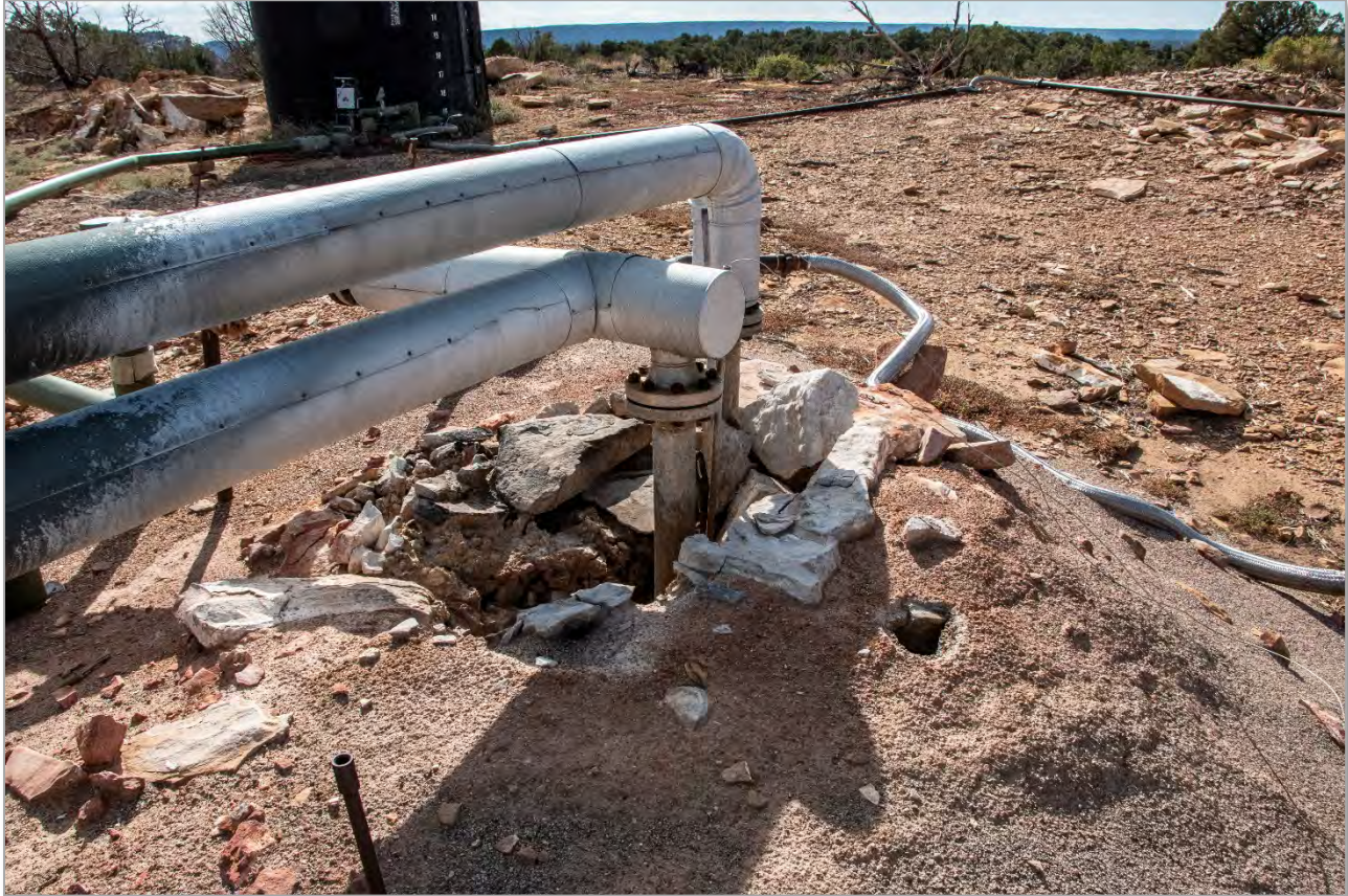
Figure 4-85 – Vent Around Vertical Pipes
