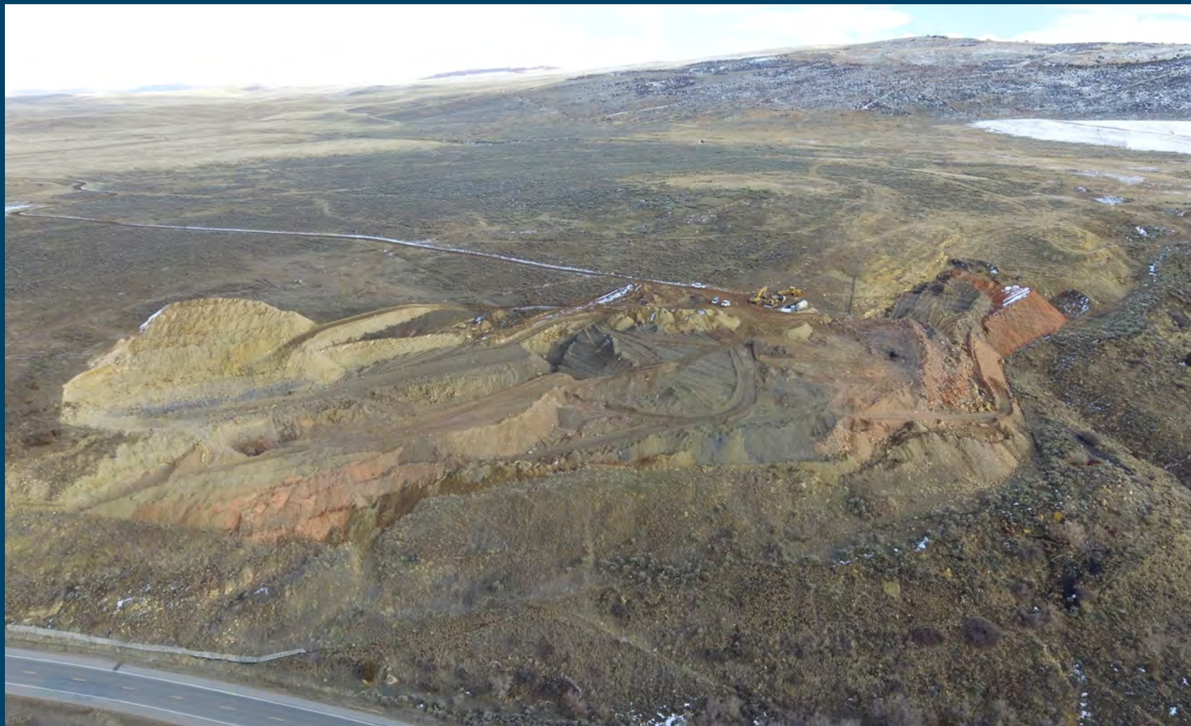
Abatement area looking East (February 13, 2018)
