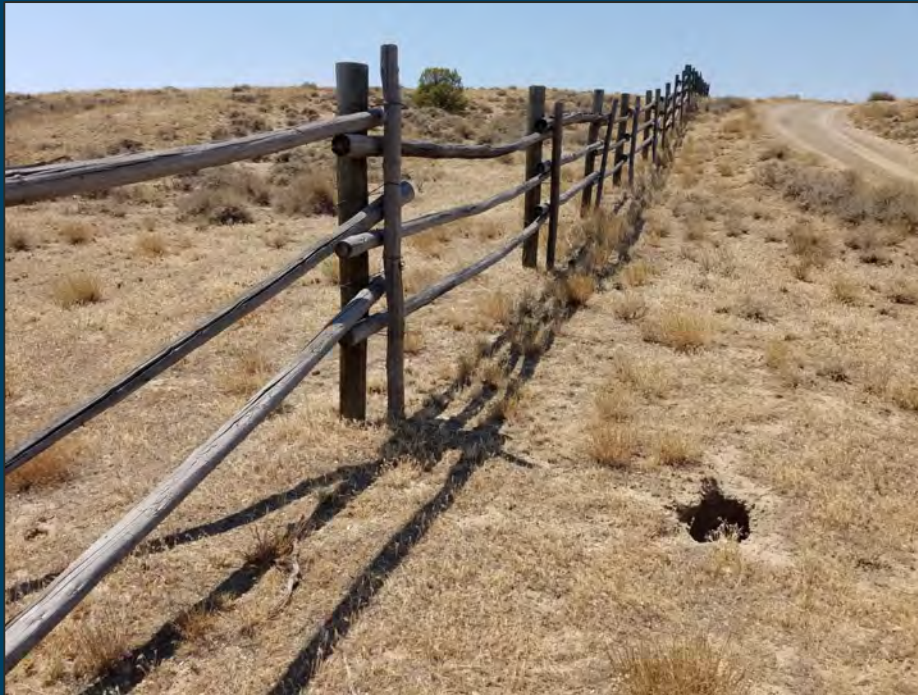
Broken fence and subsidence feature
