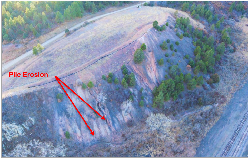
Figure 4-77 – Morley Coal Refuse Pile Looking West
