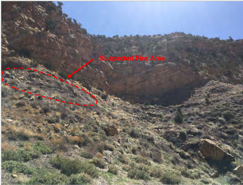
Figure 4-90 – Farmers Mutual Mine Fire Looking Southeast
