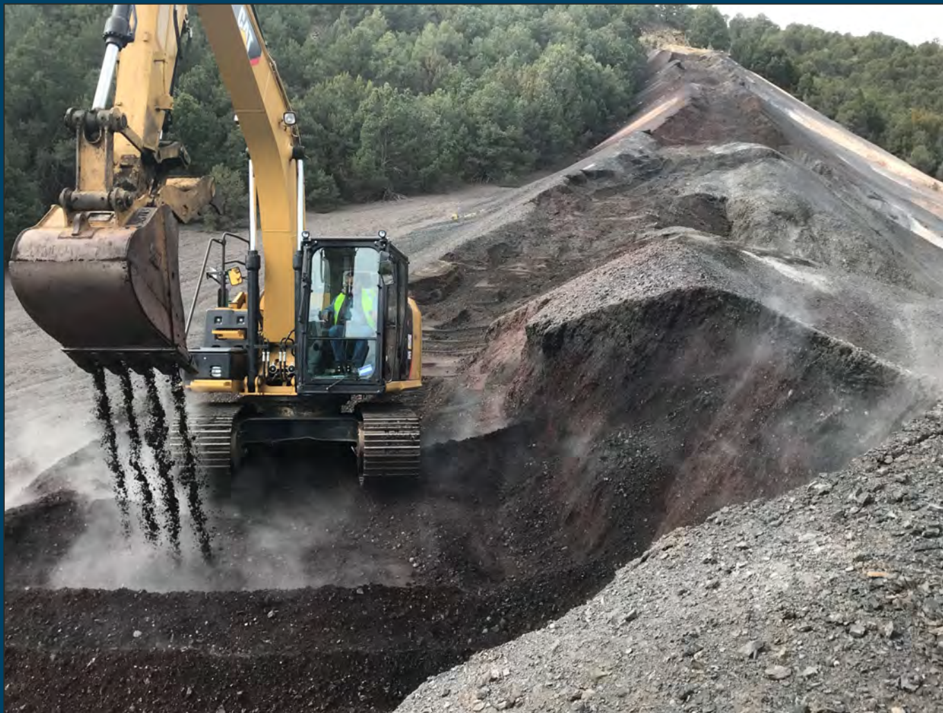
Excavating test pit
