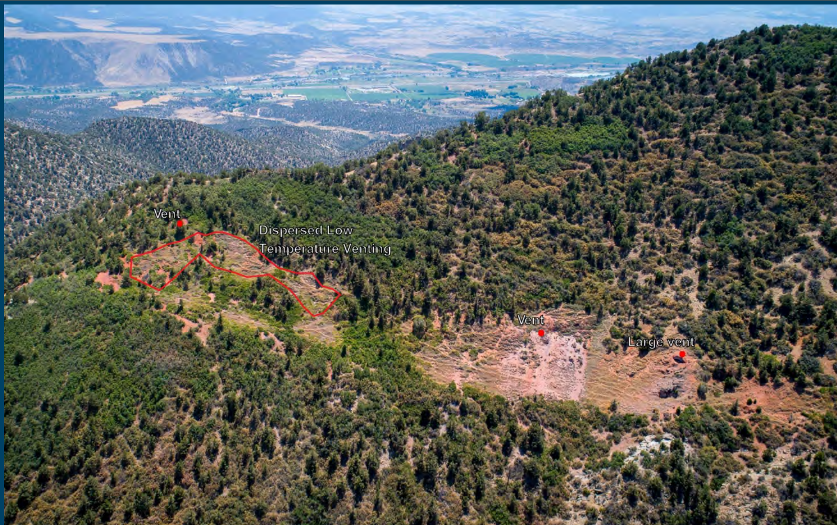
Morgan Mine fire looking South
