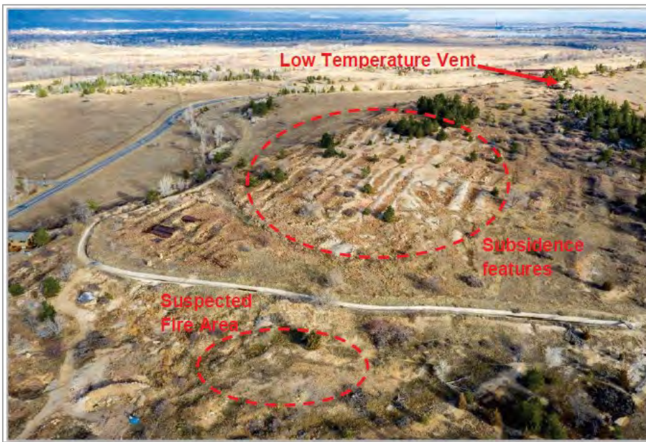
Figure 4-1 – Lewis Mine Fire Looking North
