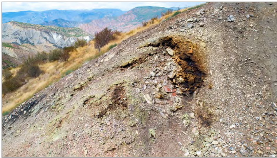
Figure 4-55 – Creosote and Sulfur Build-up at Upper Vents
