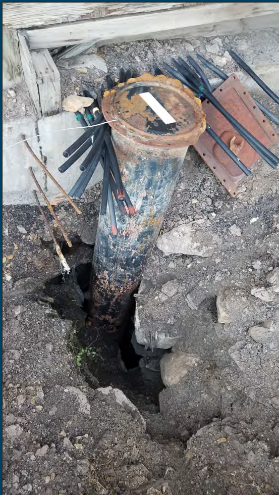
Vent pipe with opening into mine workings
