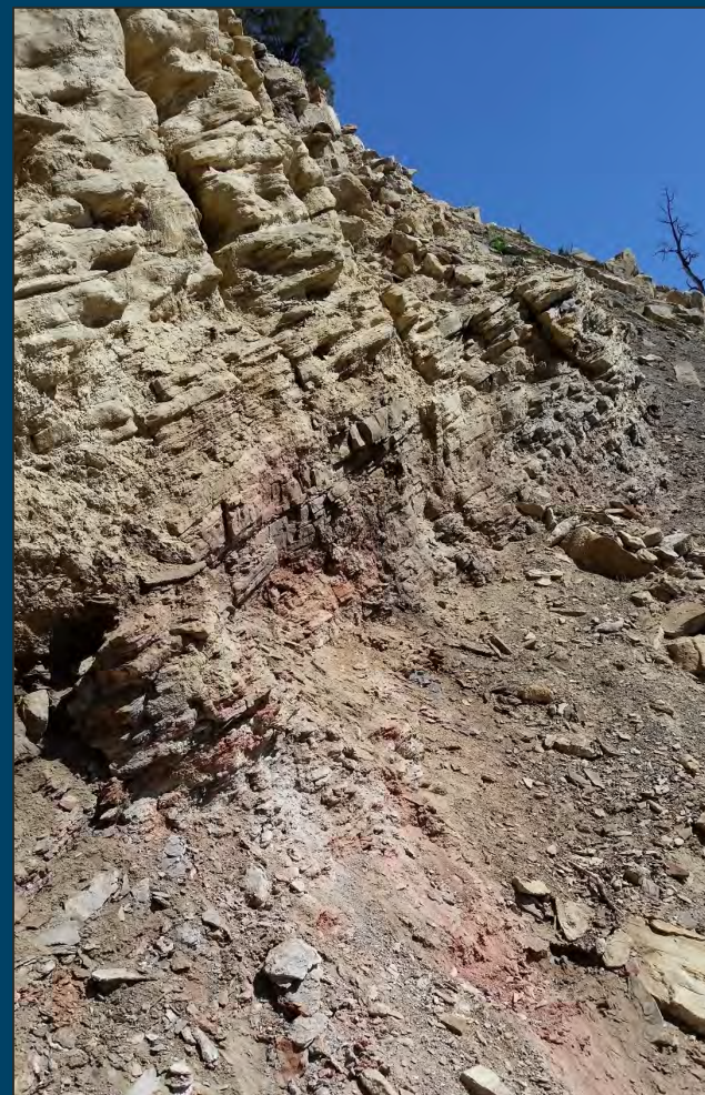
Vents along cliff base
