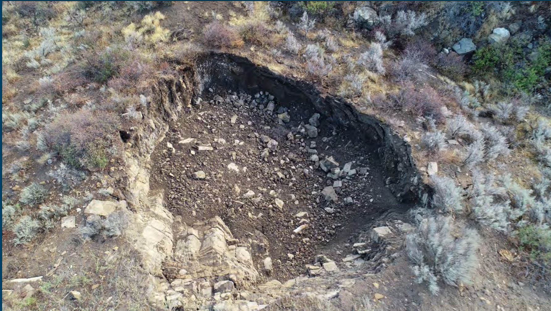
45ft diameter subsidence feature looking down
