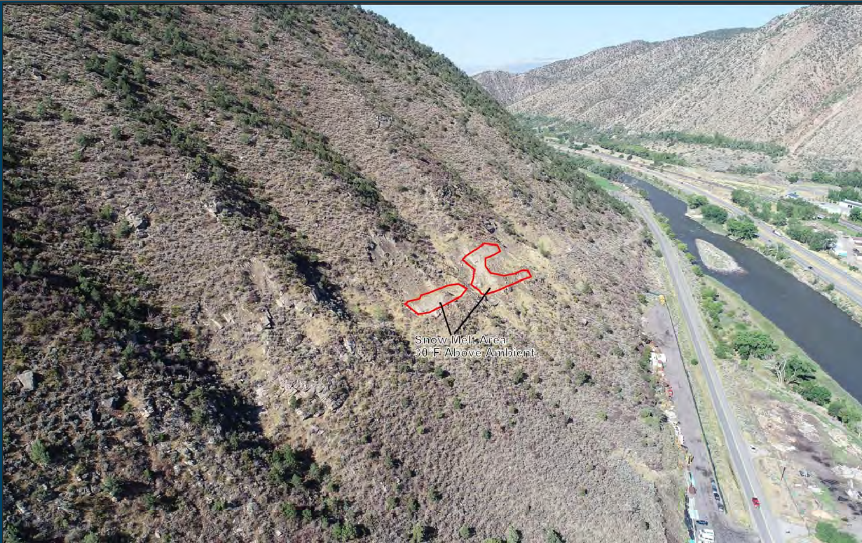
Coryell Mine fire looking West
