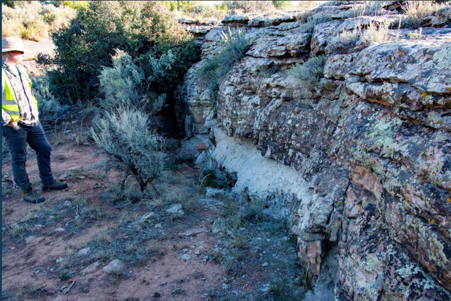
Older grout at sandstone outcrop
