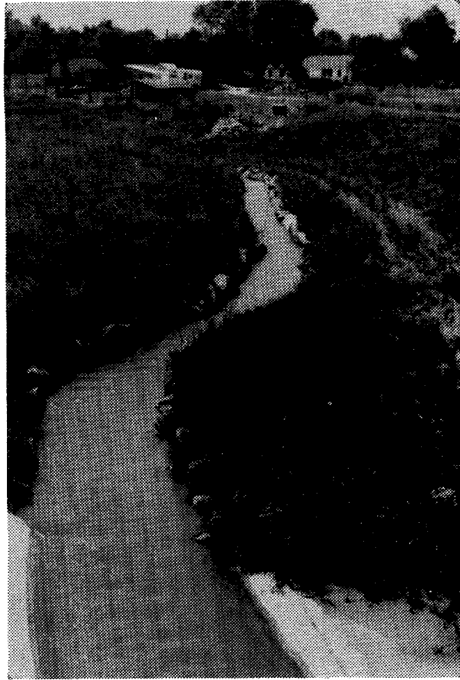
Figure 4.28. Low flow channel lined with rock for erosion control.
