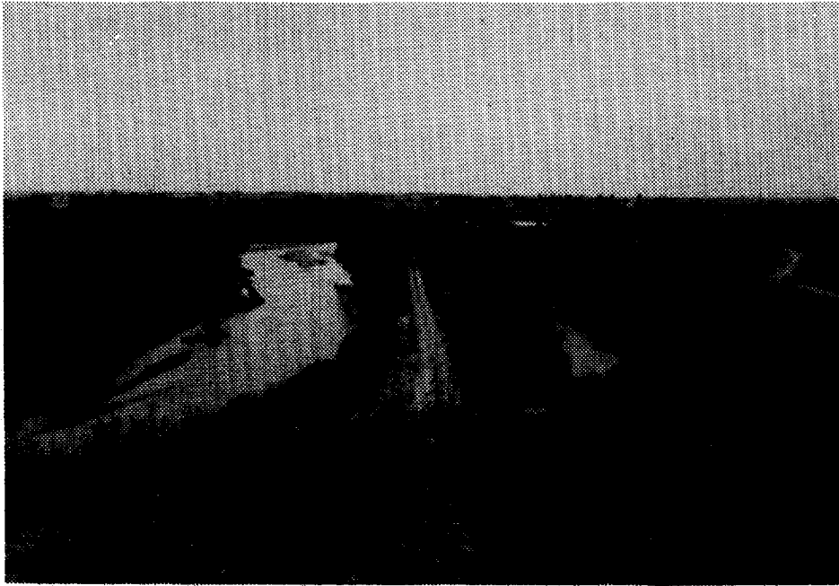
Figure 4.26. Flood control dike (at center with road) designed for 100 year flood level. Protection for sanitary landfill. St. Vrain River, Longmont, CO.
