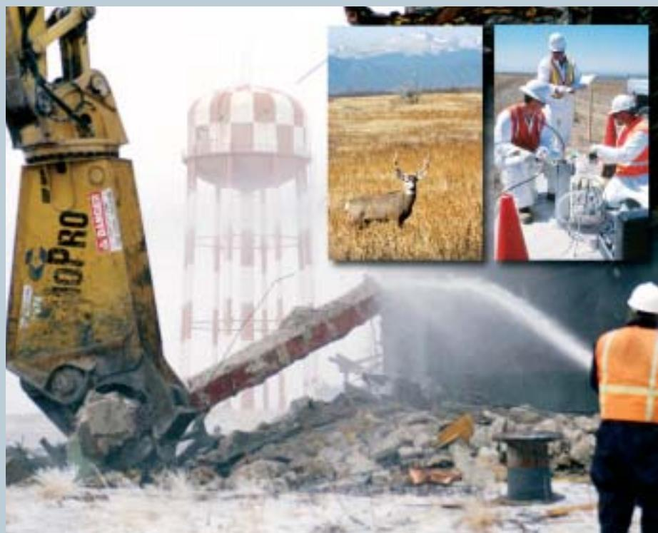
A worker sprays water to prevent dust emissions during demolition of the "north plants" at the Rocky Mountain Arsenal. Workers demolished more than 150 structures throughout the Arsenal's 17,000 acres. Monitoring groundwater quality is an important part of Superfund efforts to remove contamination and transform the site into a national wildlife refuge. Today, the U.S. Fish and Wildlife Service estimates there are more than 300 different species of wildlife found within the Arsenal boundaries.
