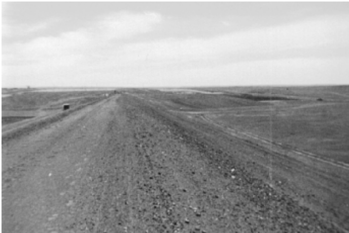
PHOTO 7.3-3—Well-graded straight crest of a newly completed dam.
