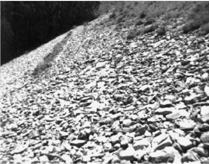
PHOTO 8.4-3—Example of well-placed riprap on the downstream slope.
