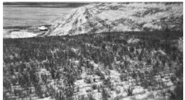
Photo 8.4-1—Early stage of growth for grass slope protection.
