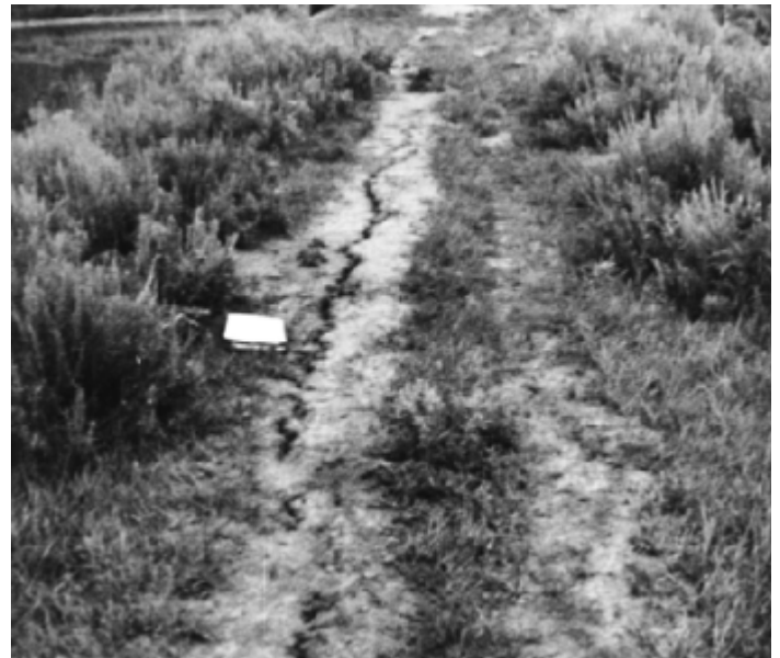
PHOTO 7.5-8—LONGITUDINAL DRYING CRACKS ON THE CREST OF A DAM. These cracks are caused by drying of the crest surface and are only 6-8 inches deep.
