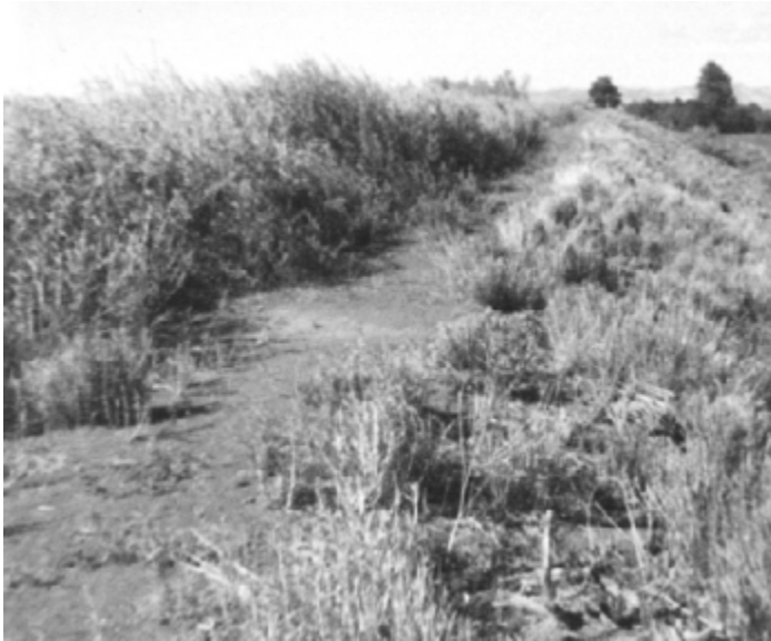
PHOTO 7.5-4—THE CREST OF A DAM PARTIALLY OVERGROWN AND OBSCURED DUE TO EXCESSIVE BRUSH GROWTH.
