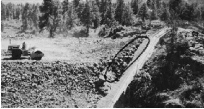
FIGURE 2.5-11—VIBRATORY ROLLER. Drums vibrate as roller moves.
