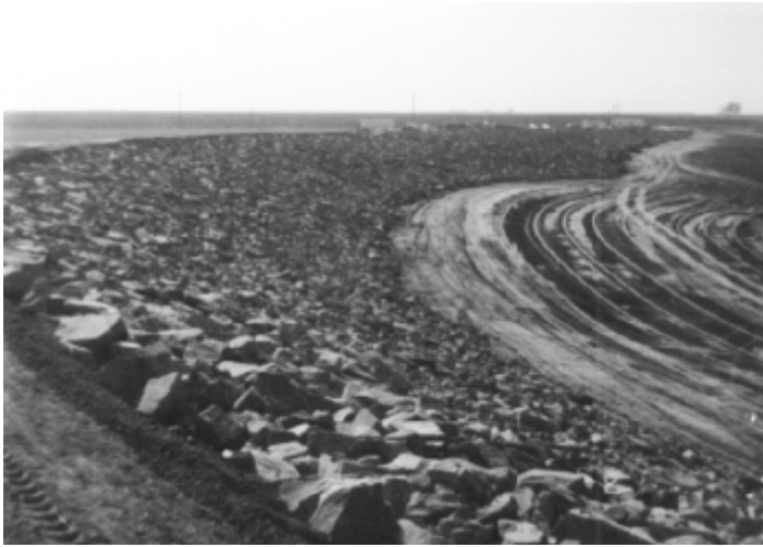
PHOTO 6.1—EXCELLENT UPSTREAM FACE. Note uniform surface or riprap protection.
