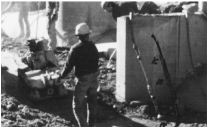
FIGURE 2.5-7—POGO STICK, SIMILAR TO TAMPING TOOL.—Is used in tight spots not accessible to larger equipment.
