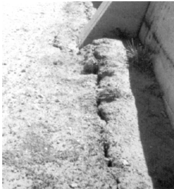
PHOTO 8.5-3—LONGITUDINAL CRACKING
