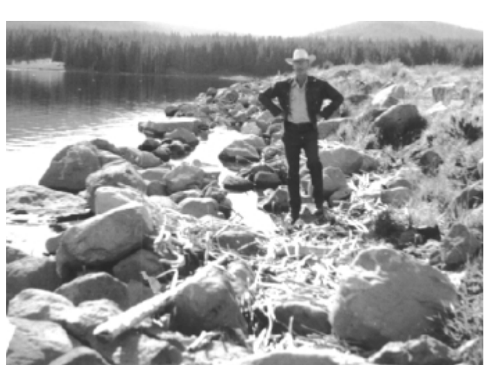
PHOTO 6.5-6—SLIDE AT UPSTREAM SLOPE. Note water line alignment
