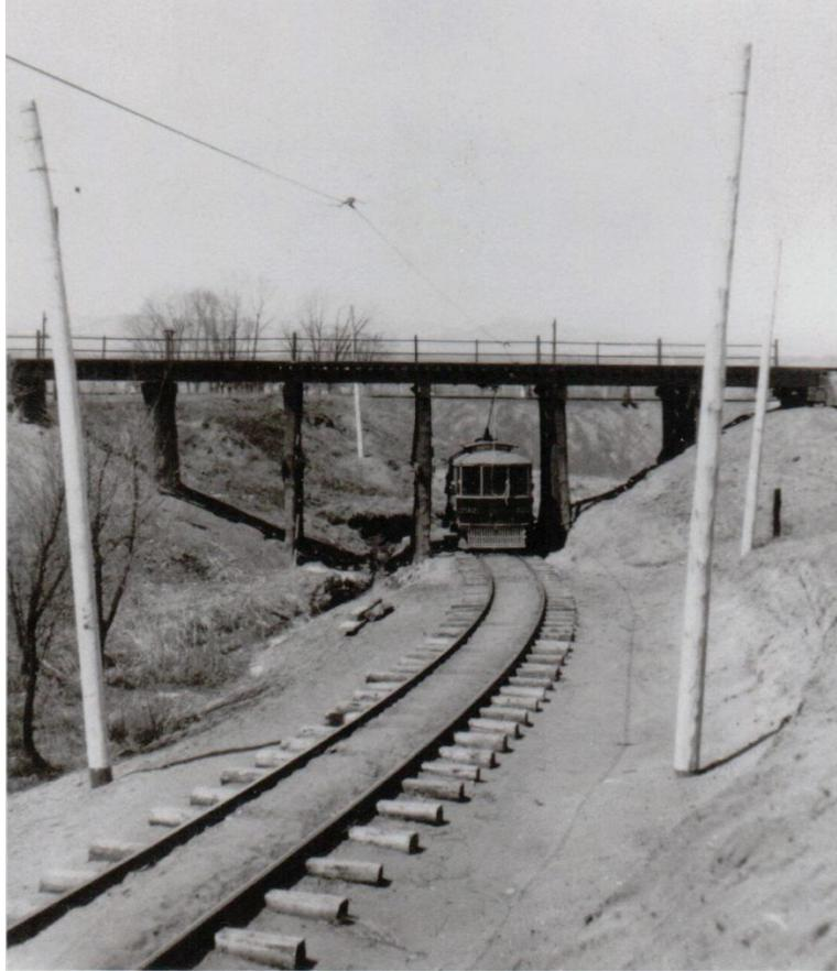
**Figure 164. D&SP streetcar in Slaughterhouse Gulch, c.1910. Note the poles carrying the electric lines installed at an angle outward to keep the electric lines taut.<sup>710</sup> (Image from the Collection of the Littleton Museum. May not be reproduced in any form without permission of the Littleton Museum.)**
