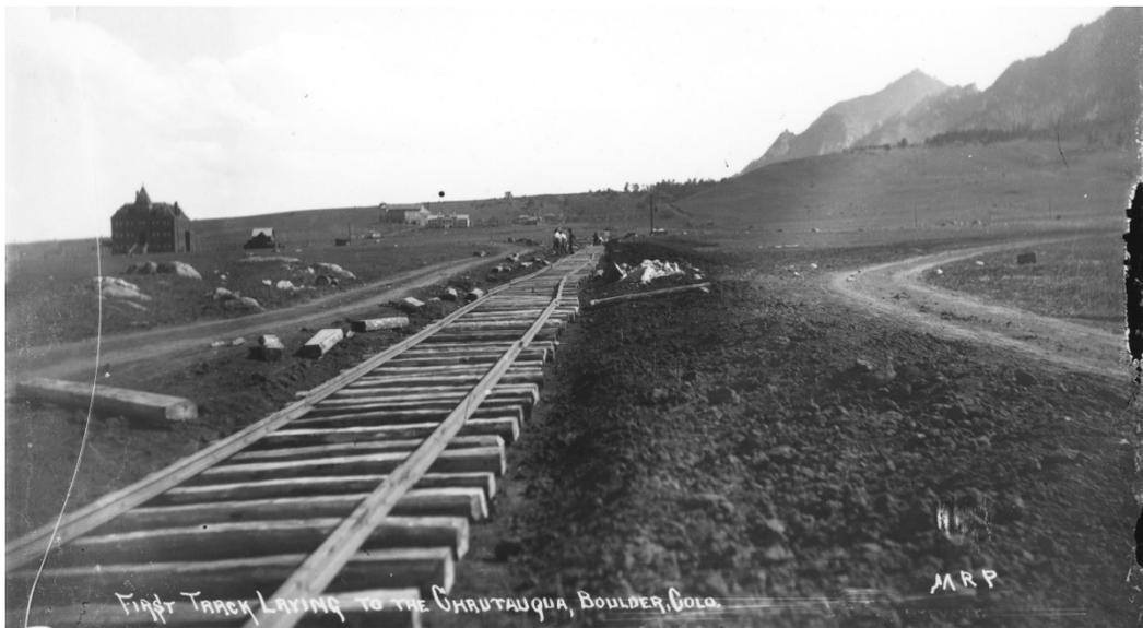
**Figure 22. Laying track on the BR&U route to Chautauqua Park in 1899.<sup>187</sup>**
