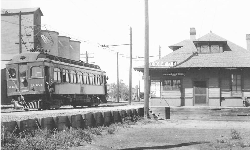
**Figure 114. D&I car outside of the Broomfield Depot, originally located at West 120<sup>th</sup> Avenue and the C&S tracks. Note the diamond-shaped pantograph atop the car.<sup>542</sup>**
