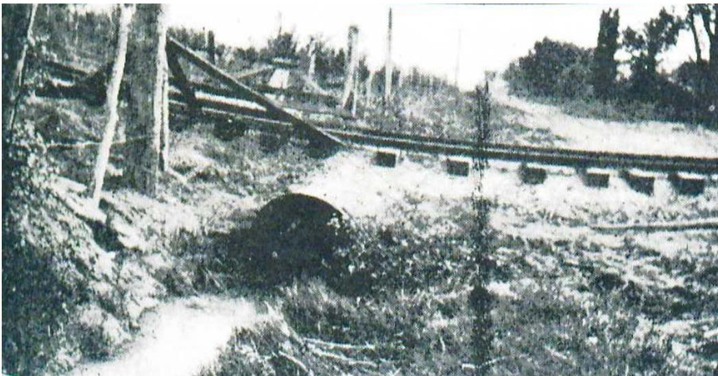
**Figure 148. A corrugated culvert on the GJ&GRV interurban line to Fruita.<sup>666</sup>**
