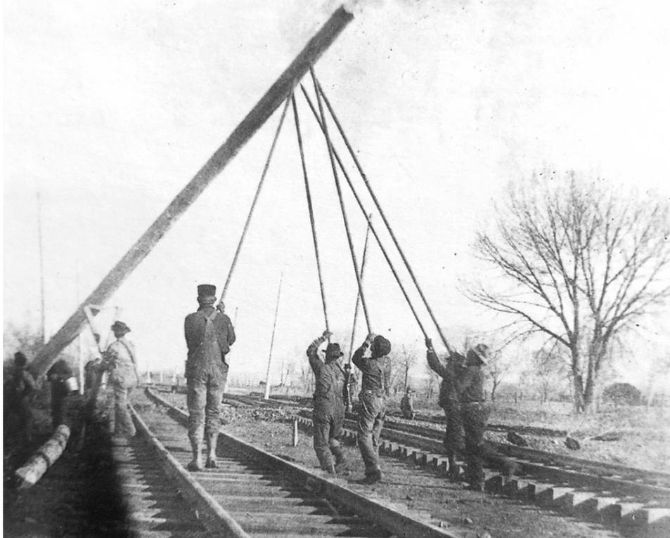
**Figure 107. Crews erecting poles to support the catenary wire on the route to Golden.<sup>515</sup> It was common practice during the first part of the twentieth century for the poles to be painted white.<sup>516</sup>**
