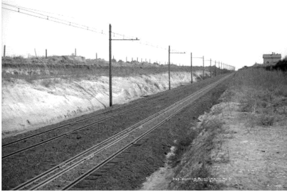
**Figure 197. Cut-and-fill embankment on the Denver & Interurban Railroad between Denver and Boulder, c.1920 (current condition unknown).<sup>773</sup>**
