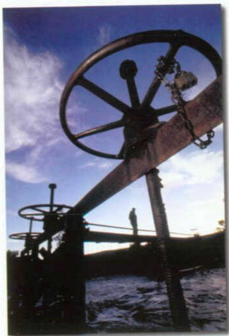
An irrigation headgate near Kremmling, Colorado controls the amount of water diverted from the Colorado River.
