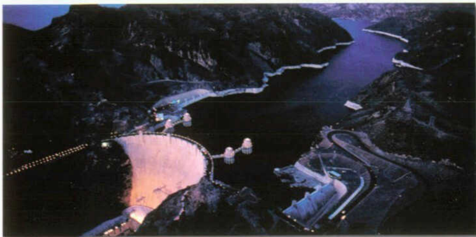
Construction of new dams is subject to federal approval. The controversial Two Forks Dam project in Colorado was vetoed by the Environmental Protection Agency (EPA) in the 1980s. When completed in 1935, Hoover Dam (above) on the Colorado River, which produces more than four billion kilowatt hours of electricity each year, was the largest dam in the world.
