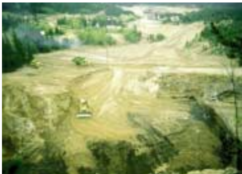
PLACING MATERIAL ON A COMPOSITE COVER
