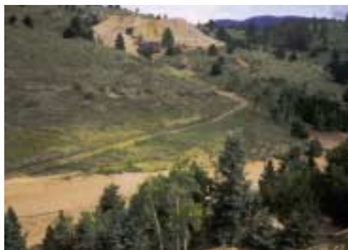
CONSOLIDATED WASTE ROCK SITE AFTER CAPPING AND REVEGETATION
