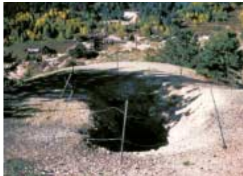
ABANDONED MINE SHAFT WITH INEFFECTIVE FENCE AND COLLAPSING WALLS
