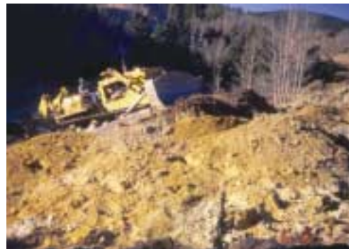
GRADING WASTE ROCK PRIOR TO CAPPING
