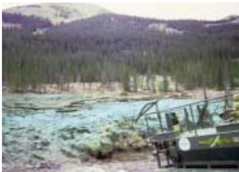
REGRADED MILL TAILINGS SITE AFTER MULCHING
