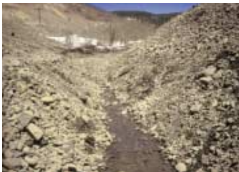
DIVERSION DITCH IN ROCKY AREA
