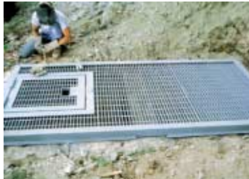
FABRICATING A STEEL GRATE WITH A LOCKING HATCH
