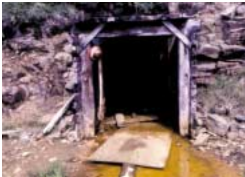
ACID MINE DRAINAGE CONTAINING HEAVY METALS
