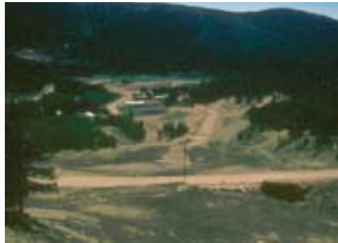
TAILINGS CAPPED, GRADED, AND VEGETATED
