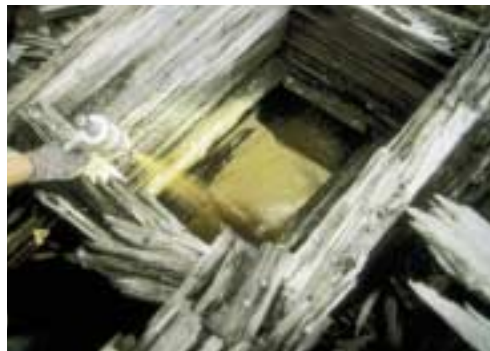
POLYURETHANE FOAM BEING INSTALLED IN A CRIBBED SHAFT
