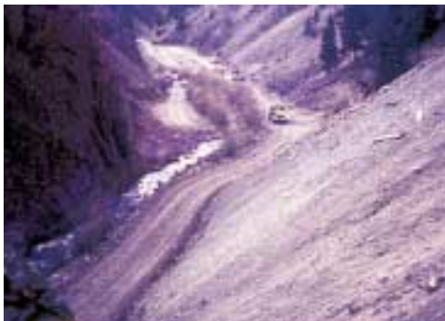
STREAM IN NEW CHANNEL SEPARATED FROM WASTE ROCK BY RELOCATED ROAD
