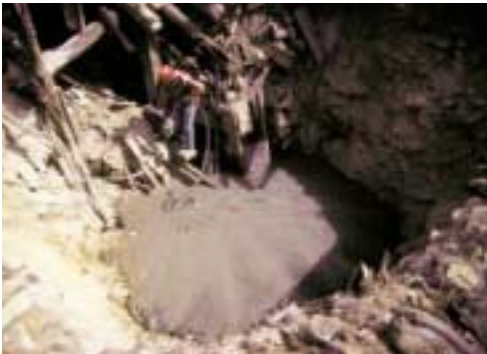
INSTALLING CONCRETE FOR A MONOLITHIC PLUG
