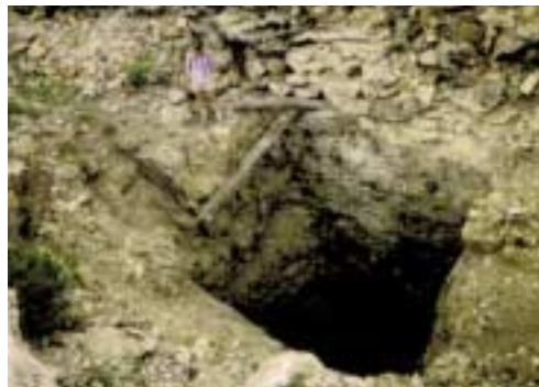
accessible openings into the rock or soil;
