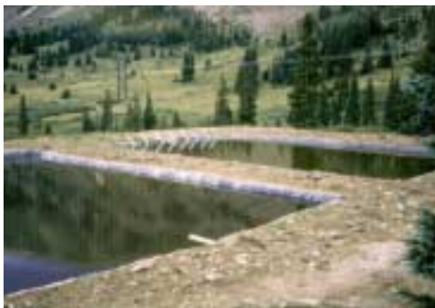
SULFATE-REDUCING WETLANDS WITH HDPE LINERS
