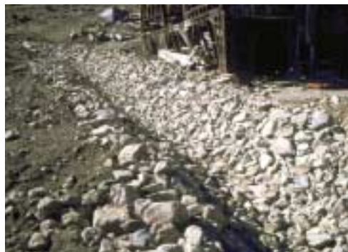
DIVERSION DITCH LINED WITH RIPRAP
