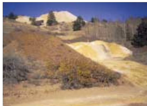
RELOCATED MINE WASTE PRIOR TO FINAL GRADING AND CAPPING
