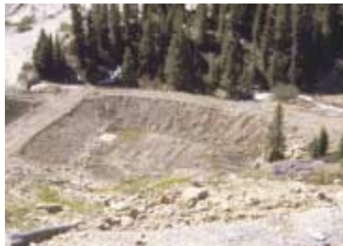
SETTLING POND AT A MILL TAILINGS SITE
