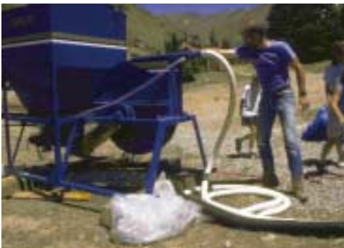
SMALL-SCALE PILOT LIME INJECTION SYSTEM
