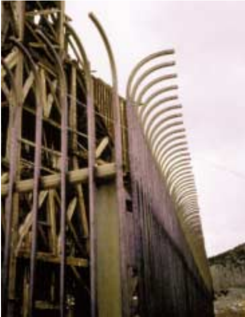
CUSTOM STEEL FENCE AROUND AN HISTORIC HEADFRAME AND SHAFT
