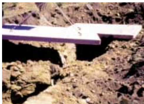
PLACING PRECAST CONCRETE PANELS OVER A STOPE
