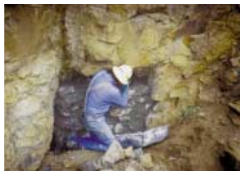
FINISHING CONSTRUCTION OF A NATIVE ROCK BULKHEAD AT AN ADIT
