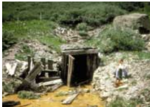
drainage from suspected mine openings (even if collapsed);
