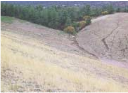
GULLIES IN A REGRADED SLOPE
