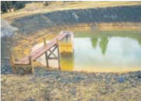
SETTLING POND BELOW A LIMESTONE INJECTION SYSTEM
