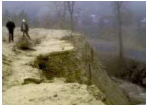
MILL TAILINGS BEING ERODED BY AN ADJACENT STREAM
