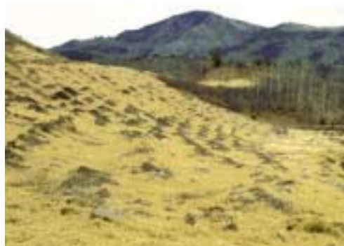
NEWLY-RECLAIMED SLOPE ROUGHENED TO HELP IN ESTABLISHING VEGETATION
