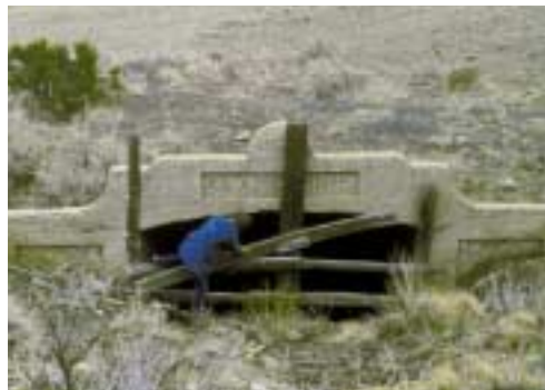
INEFFECTIVE BARRIER AT AN ABANDONED COAL MINE ALLOWING ACCESS TO THE WORKINGS
