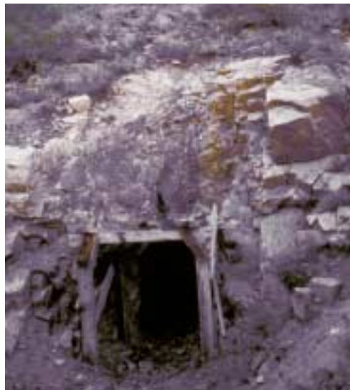
ADIT OPENING WITH TIMBERED ENTRY
