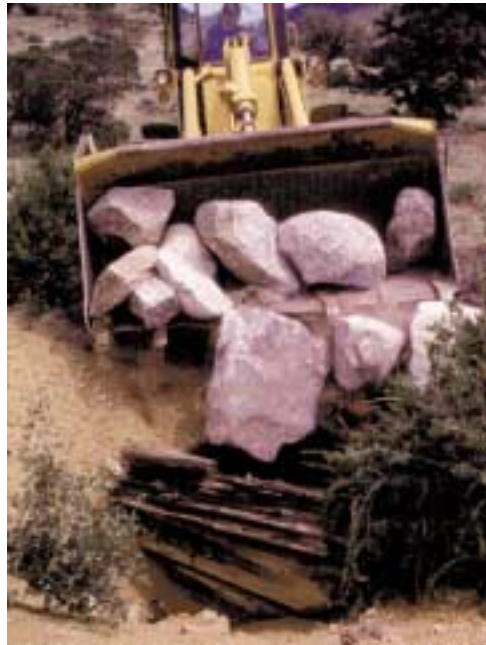
BACKFILLING A SHAFT USING RIPRAP
