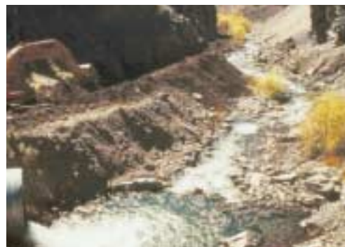
NEW STREAM CHANNEL UNDER CONSTRUCTION
