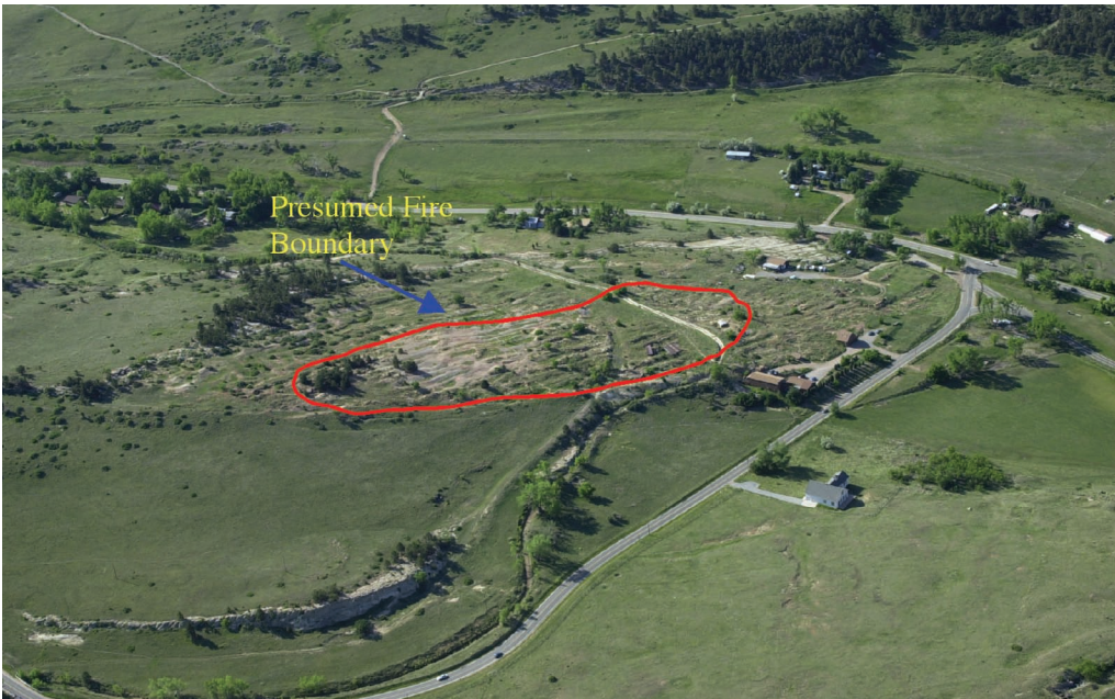
Lewis Number 1 and 2 Coal Mine Fire. View toward South.
