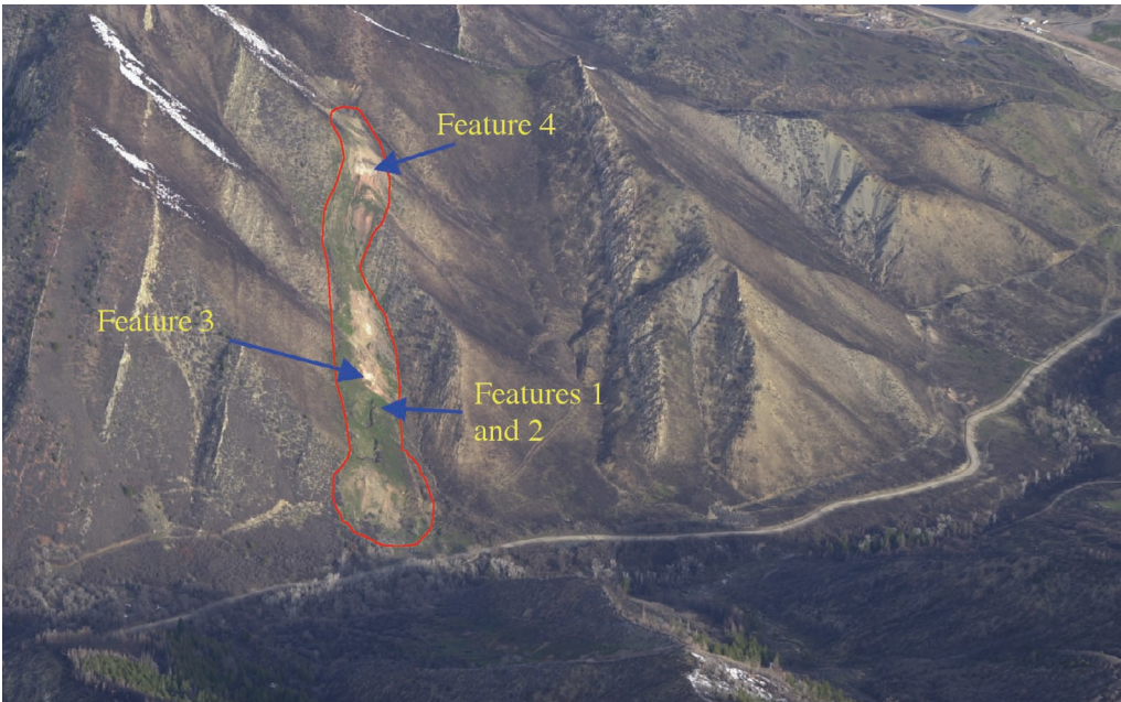
South Cañon Number 1 Mine Fire, West Burn Zone.
