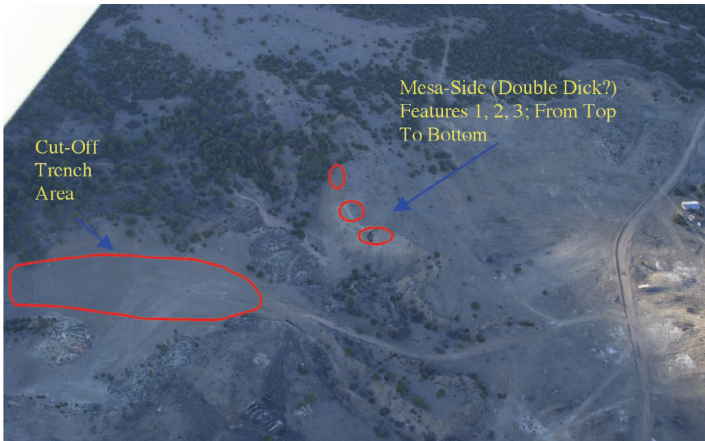
Double Dick Mine Fire Vicinity. Features 1, 2, 3; from top to bottom. View towards North.
