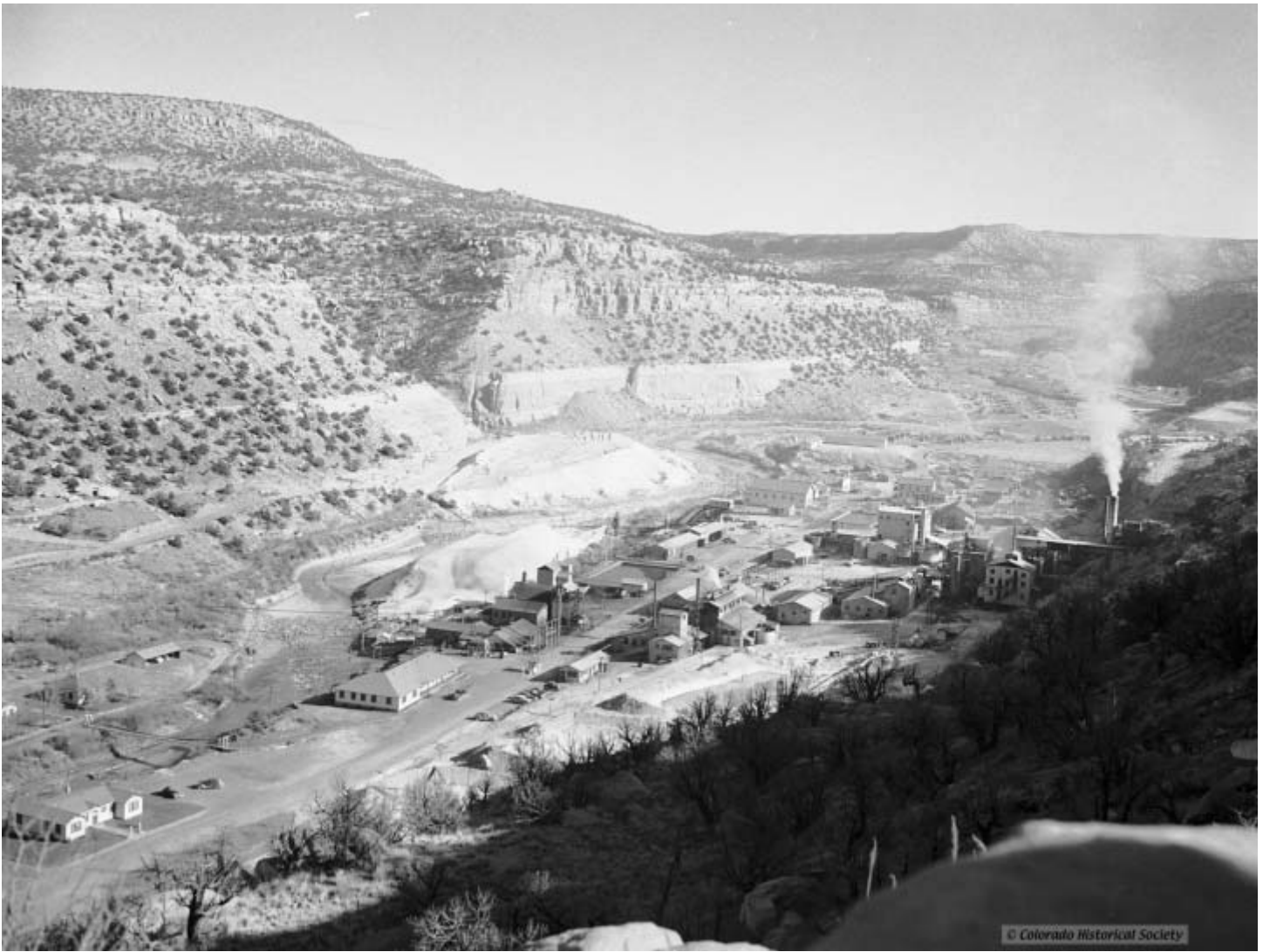
Figure 7. United States Vanadium Company plant, Uravan, in the late 1930s or early 1940s. Photograph courtesy of the Colorado Historical Society, CHSX 6203. (Photograph by Bob Zellars)
