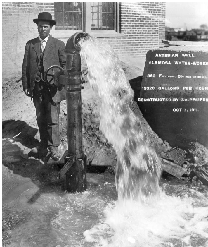
Artesian well at Alamosa Water works, 13,320 gallons per hour, constructed by J.A. Pfeifer, October 7, 1911
