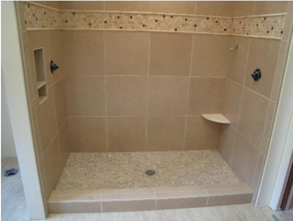
Tiled Shower Pan and Shower Walls
