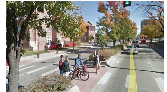
Image Showing a Crosswalk with a Median Safe-Haven
