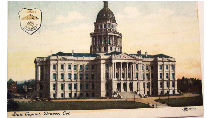
Image Showing Historic View without Parking
