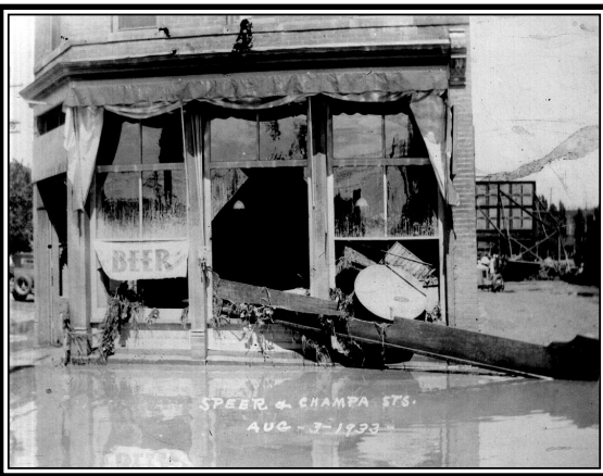
This demolished business at Speer and Champa Streets shows the power of the frightening flood. Photo courtesy of Denver Public Library.
