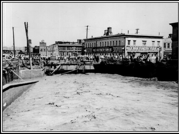
People flocked to the bridges to view the damage. The bridges themselves formed "dams" as trees and animals and other debris caught against them. This is the Blake Street Bridge. Photo courtesy of Denver Public Library.
