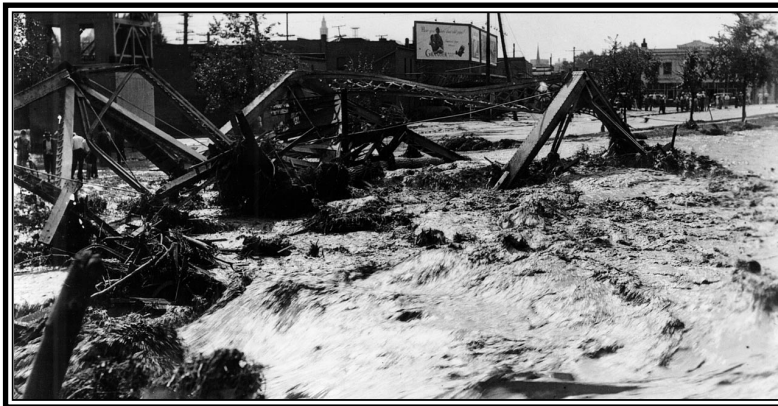
The Stout and Champa Street steel bridges floated downstream until they "fetched up" against the Curtis Street Concrete Bridge. Photo courtesy of Colorado Historical Society.
