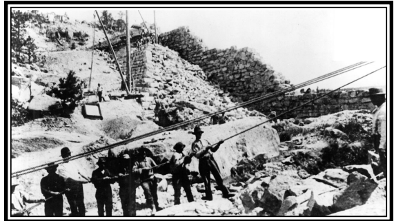
Some 335 men and 180 teams of horses worked 11 months building the dam and the Arapahoe ditch that ran down the canyon to smaller reservoirs and irrigation canals. Photo courtesy of Denver Public Library.
