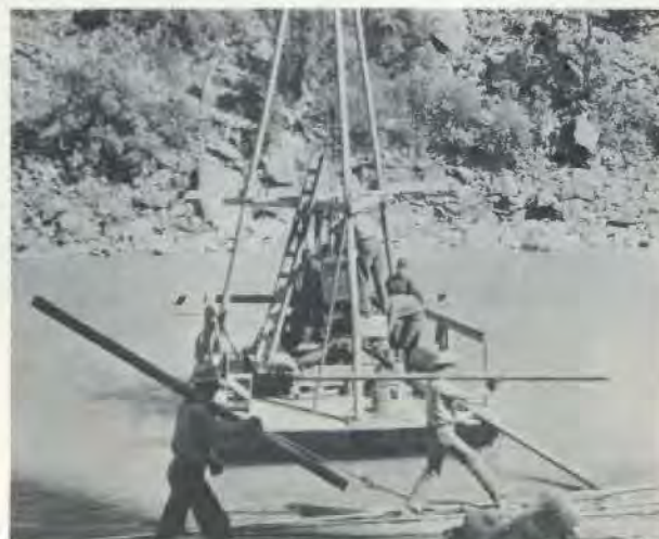
Work begins on Flaming Gorge Dam
