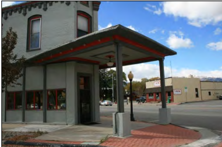
5CF.2858, Buena Vista, 111 E. Main Street, Calder Block, Wedge Building (1883)
