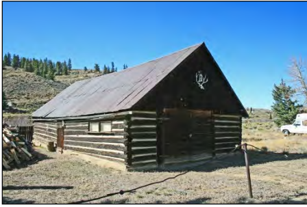
5CF.150, Granite, 43255 County Road 397 (north building), Granite Livery Stable and Blacksmith Shop (ca. 1860s-80s)
