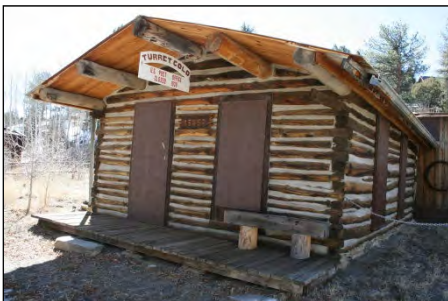
5CF.2904, Turret, 15257 Turret Avenue, Turret Post Office (Pre-1903)
