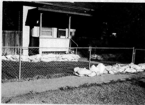
Sandbagged House on Custer Avenue
