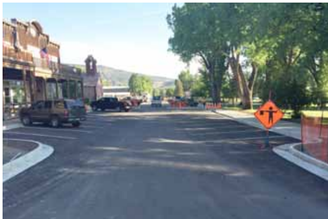
After. Paved streets, sidewalks and bulbouts helped make downtown more pedestrian friendly. Ridgway.
