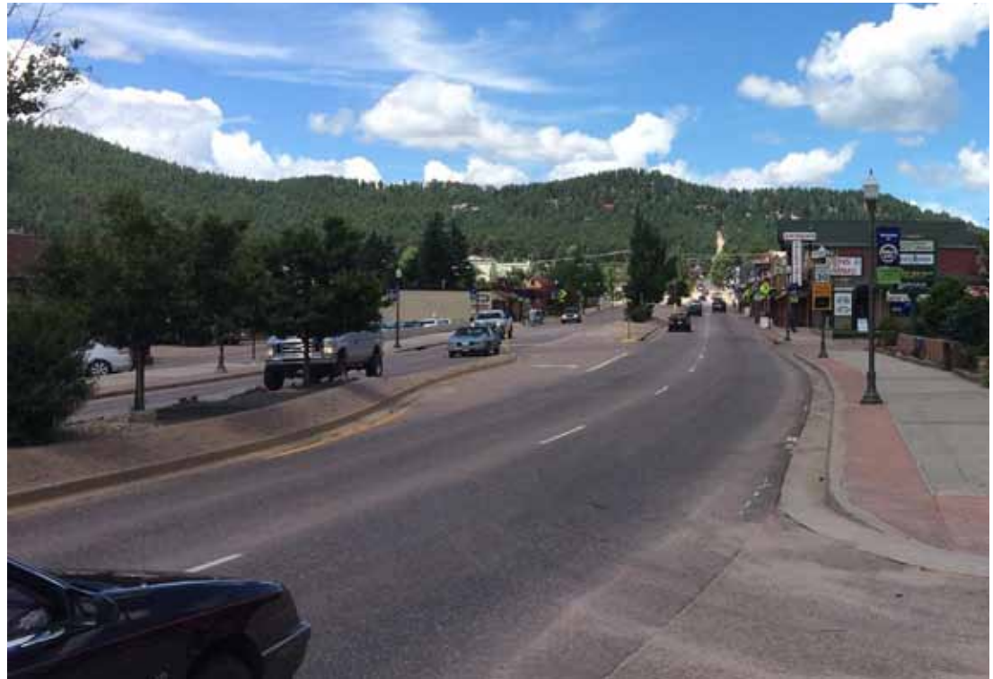
Raised medians reduce the risk of collisions, help slow down traffic and enhance pedestrian safety. Woodland Park.
