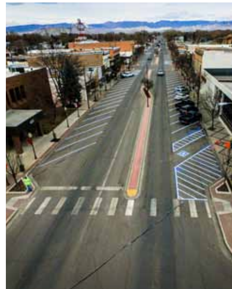
E. Main Street after introduction of diagonal parking. Montrose.
