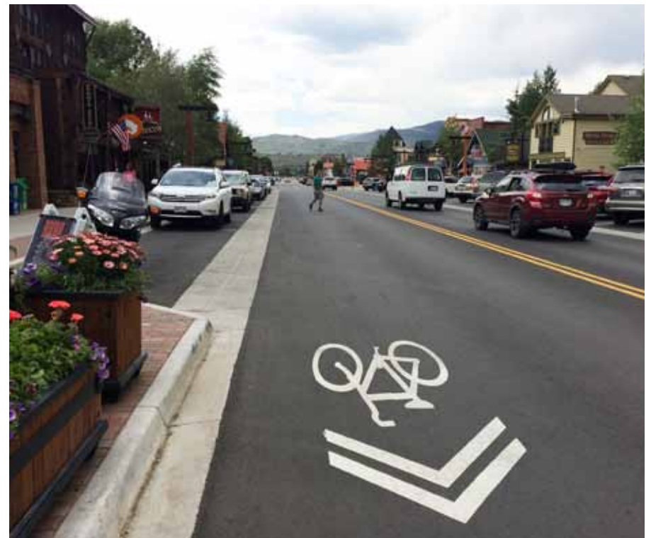
“Sharrows” provide notice to motorists that bicyclists may share the lane with moving vehicles. Frisco.
