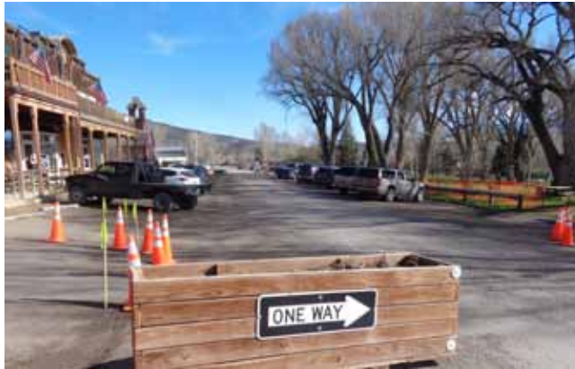
Before. Dirt roads were common in Ridgway's downtown before construction. Ridgway.
