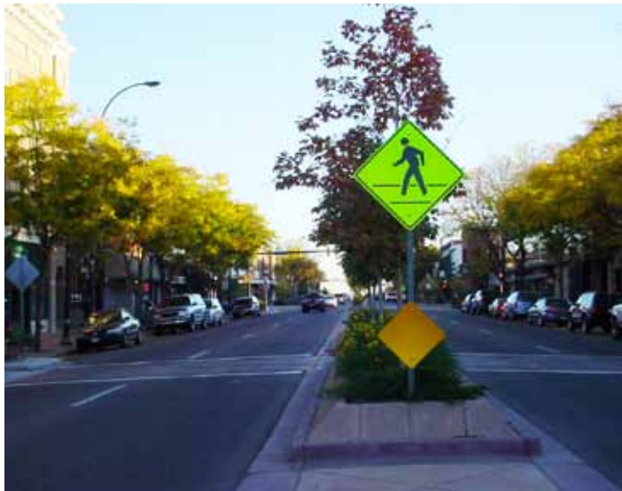
Pedestrian refuge islands help people cross four or more lanes of traffic. Longmont.
