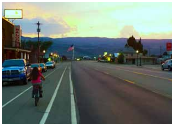
The road diet reduced the total number of lanes to three and added bicycle facilities. Kremmling.
