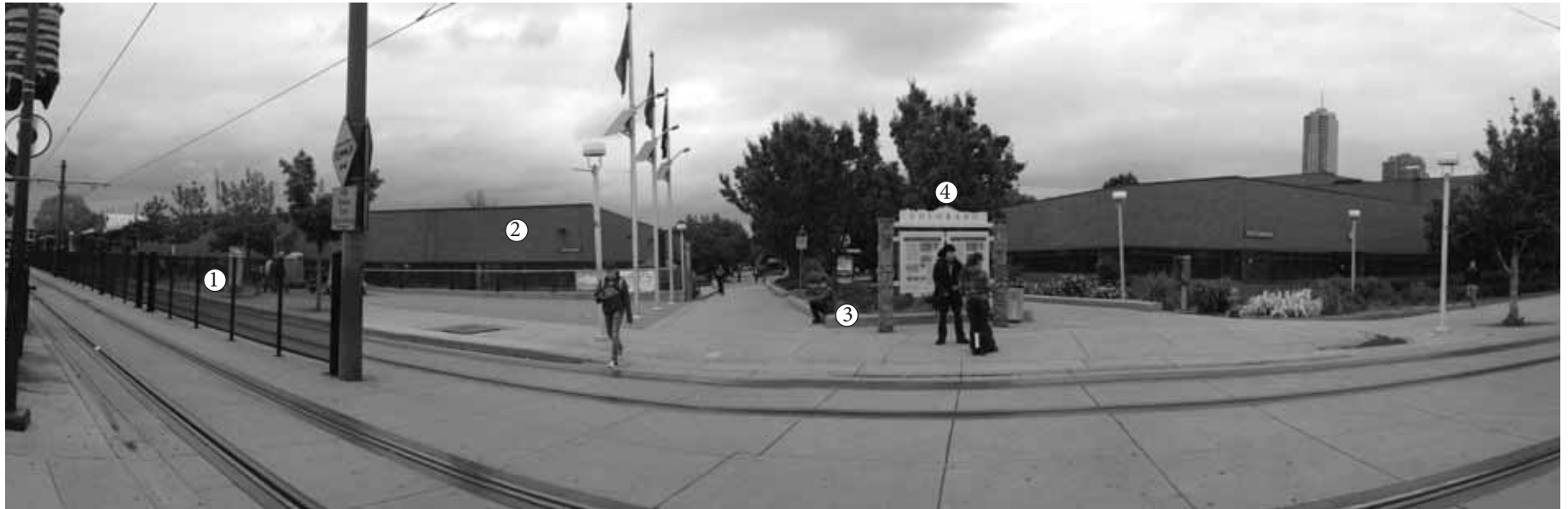
Existing Conditions at 10th Street and Colfax Avenue looking north
