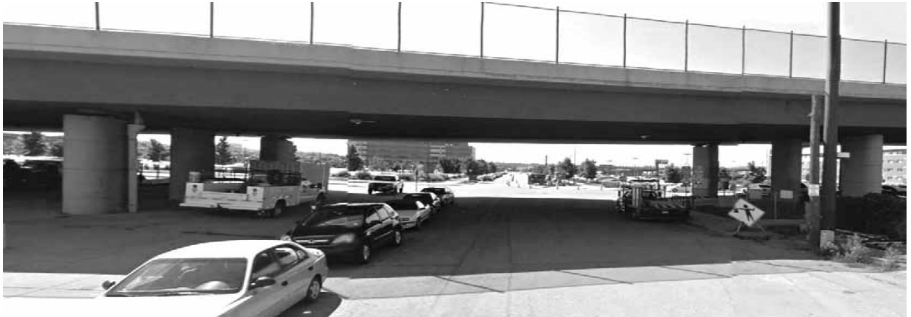
View beneath the Auraria Parkway Bridge at 5th Street
