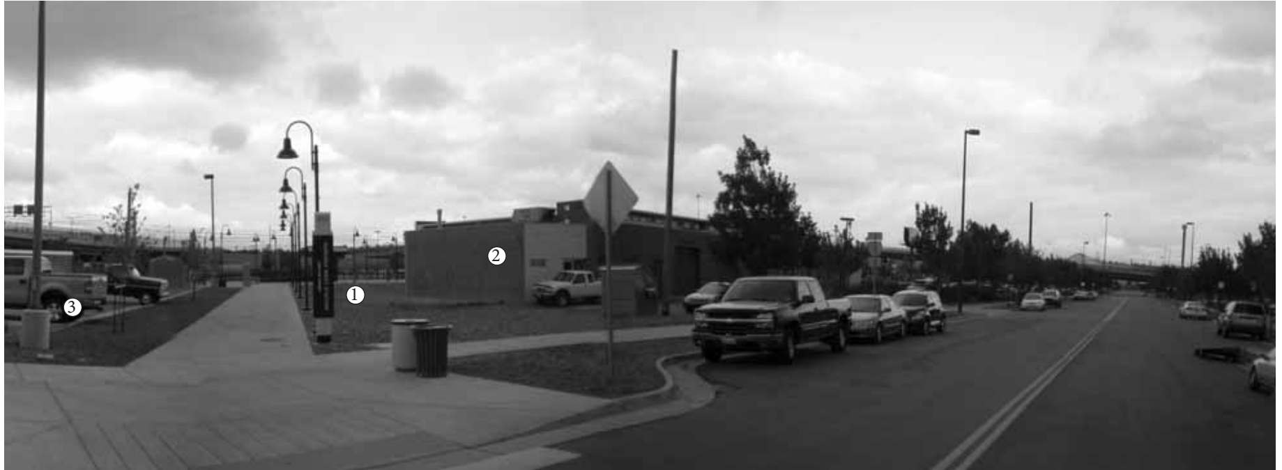
Existing Conditions at 5th Street and Lawrence looking towards Auraria West Station
