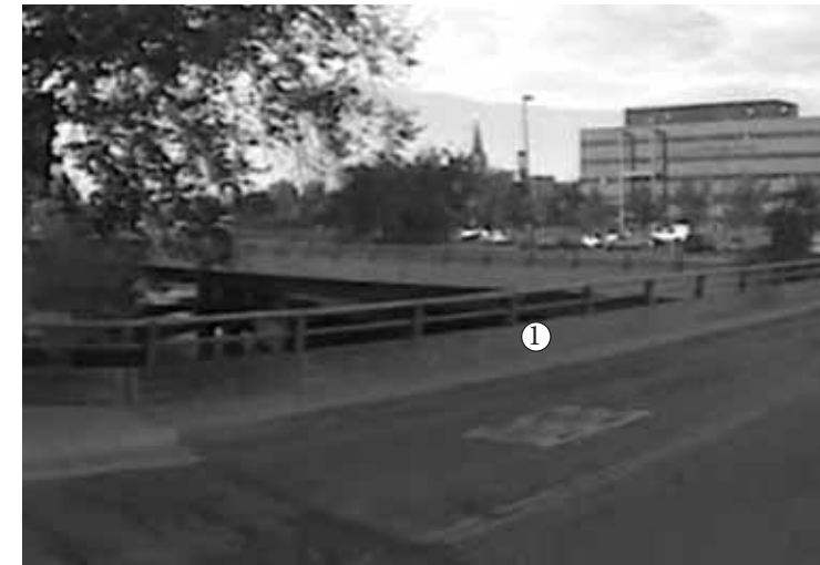
Existing Conditions on Larimer at Cherry Creek looking northwest
