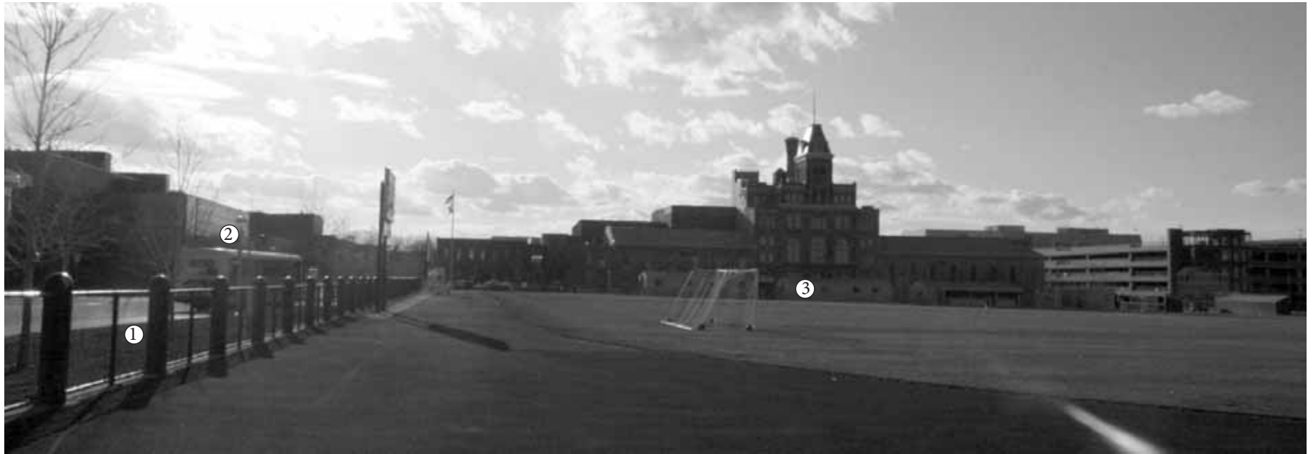
Existing Conditions at the Southeast Corner of the Tivoli Field
