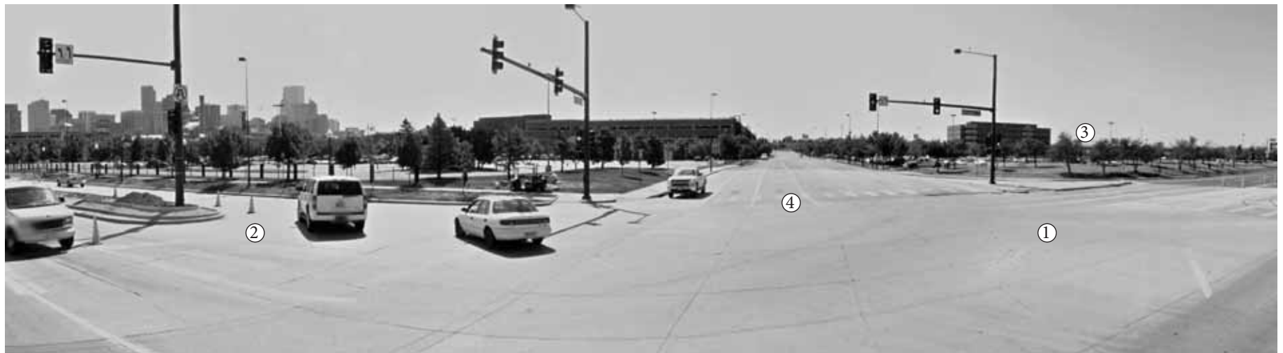
Existing Conditions at 7th Street and Auraria Parkway looking southeast
