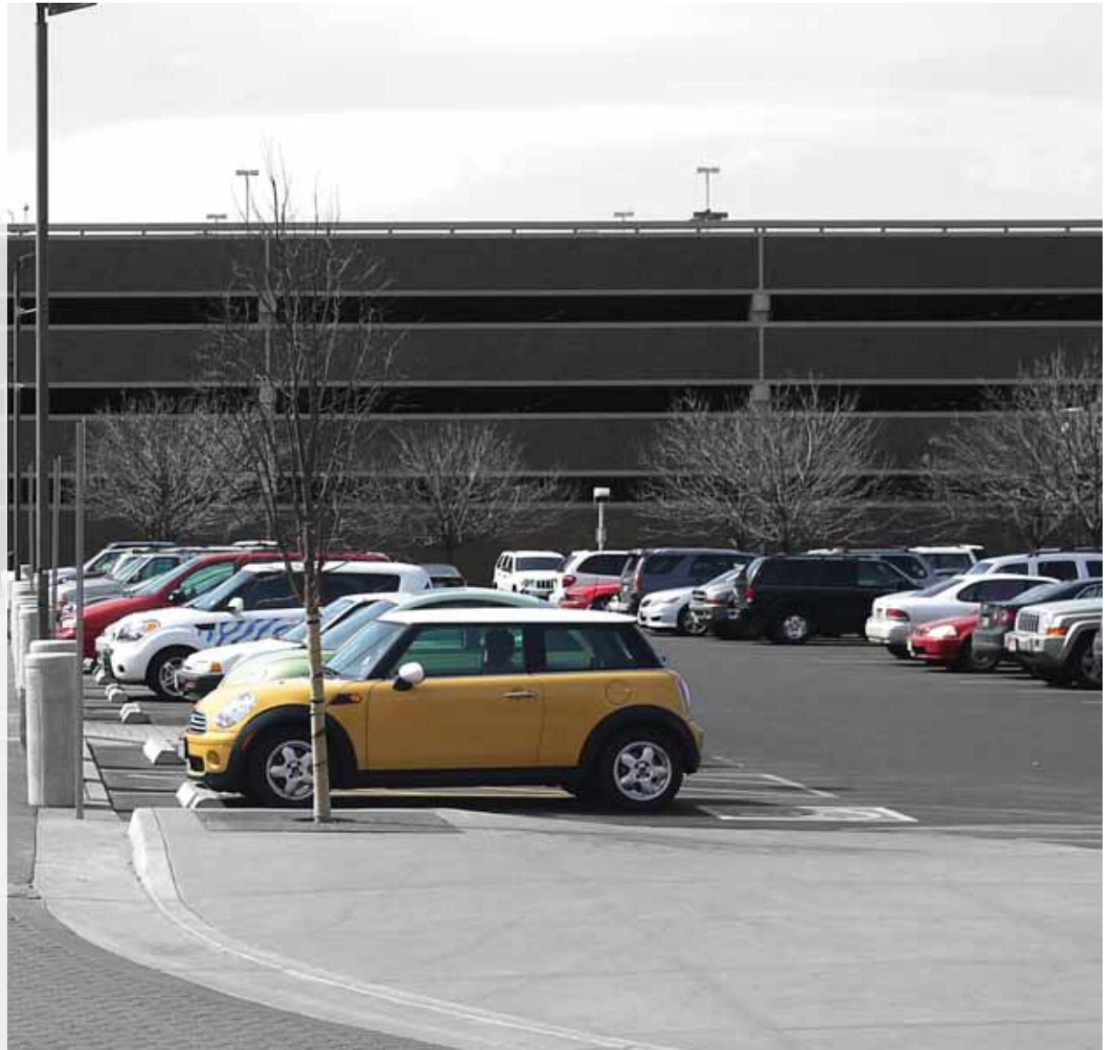
Long-range Parking Planning must Address Opportunities for Integrated Parking Structures and Reduction of Parking Demand
