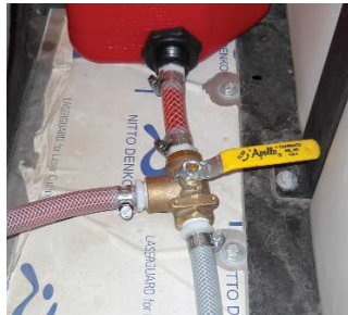
Valve position for antifreeze
