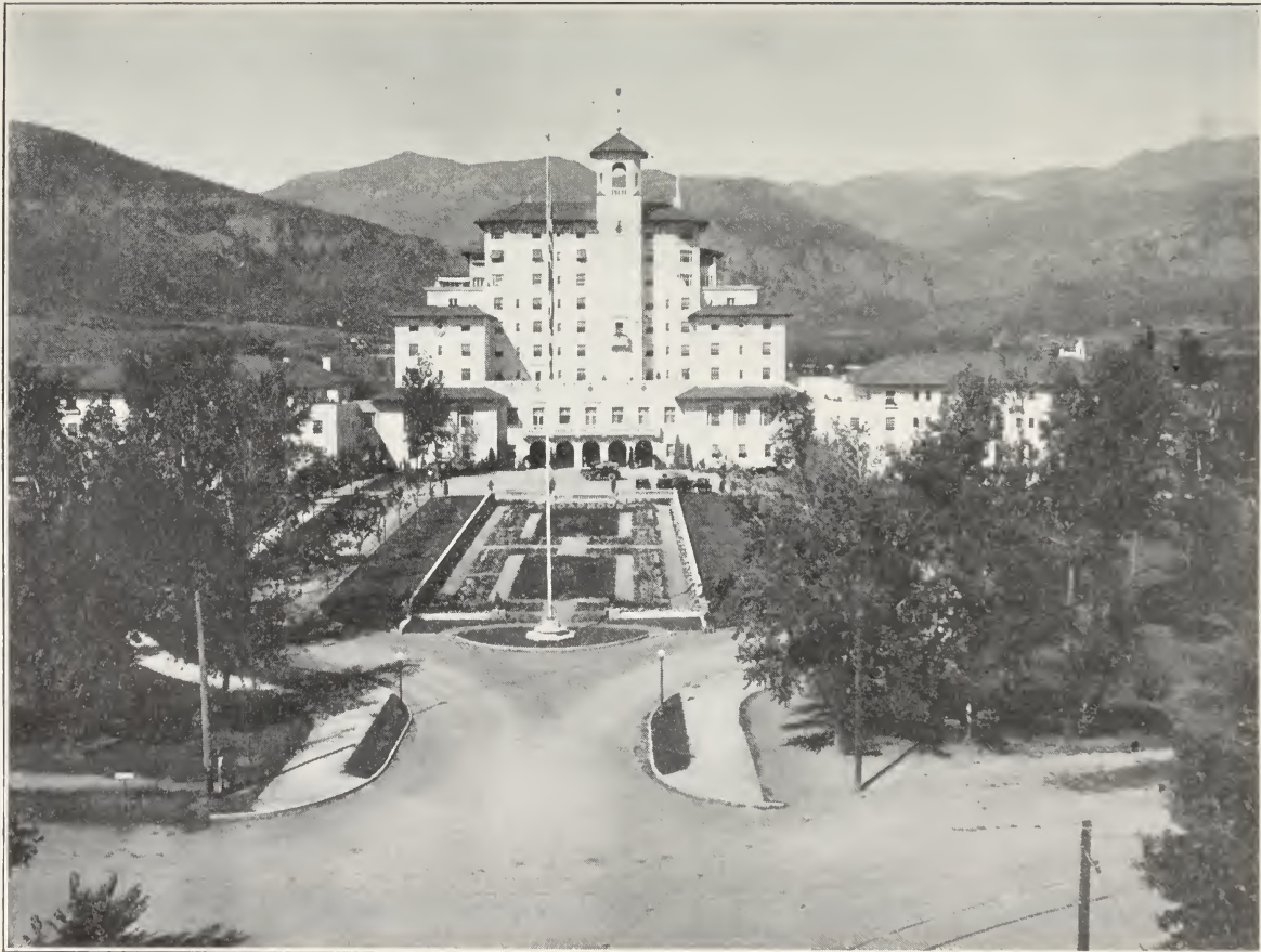
THE BROADMOOR HOTEL, COLORADO SPRINGS
