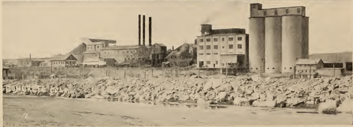
1. VALMONT POWER STATION, PUBLIC SERVICE COMPANY OF COLORADO 2. PLANT OF THE UNITED STATES PORTLAND CEMENT COMPANY AT CONCRETE, COLORADO
