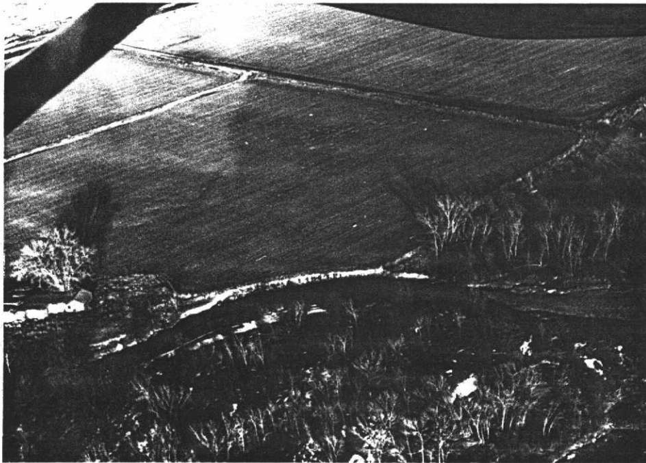
Left bank failure by erosion. Result will be a major channel realignment and flooding of Ironstone canal.
