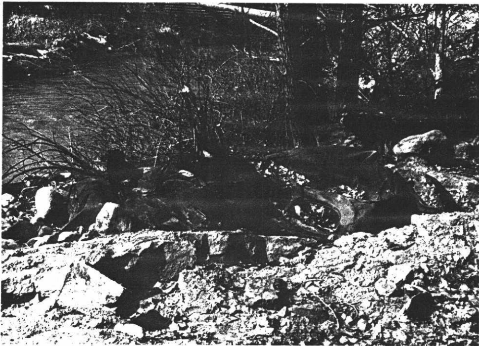
Upstream of County Road B. Three types of rip-rap materials - Sandstone, car body and volcanic rock.
