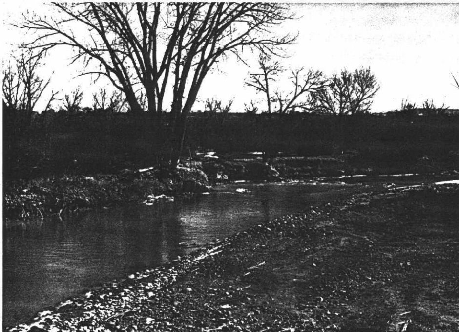
Sand bar causing bank and roadway abutment erosion.
