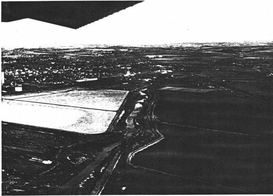
Uncompahgre River confluence with the Gunnison River - Levee repair on left bank looking upstream.
