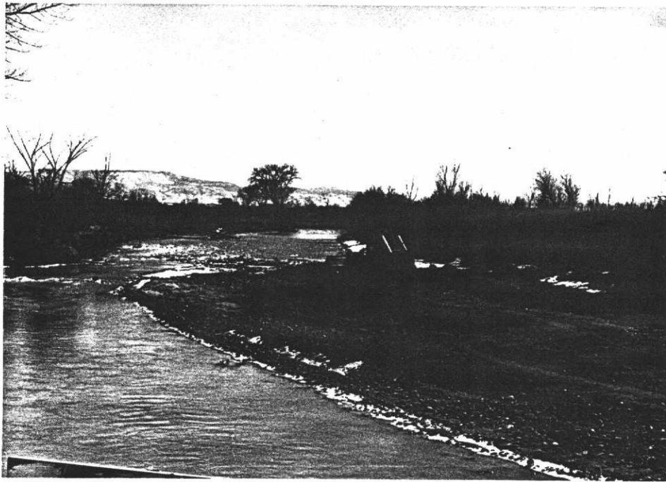
Removal of sand bar with rubber tire equipment.
