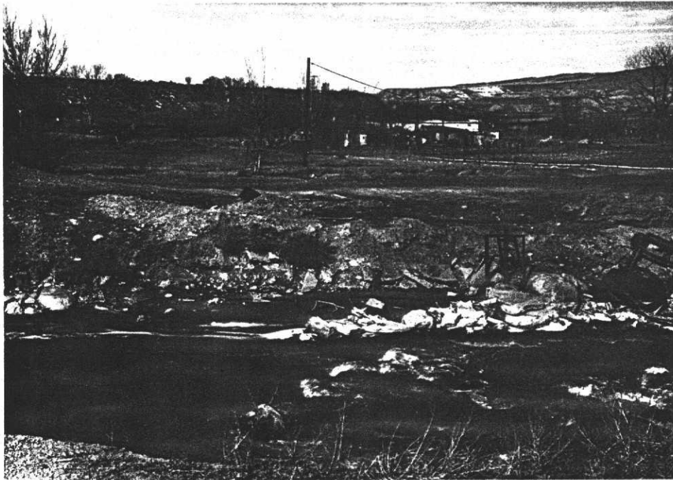
Irrigation diversion structure washed out.
