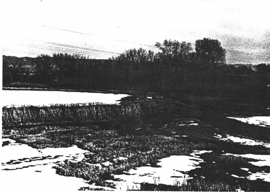
Dike of Lake No. 2 in Chipeta State Park severely eroded.
