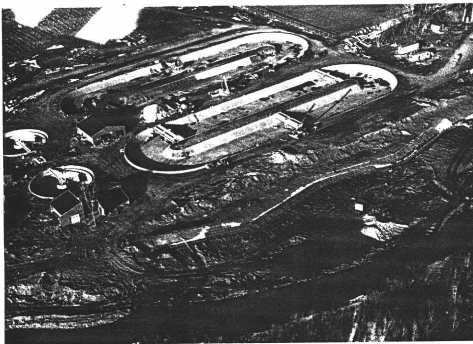
Left bank stabilization required for erosion protection.
