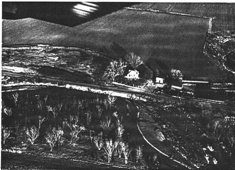
County Road 1600 repair. Channel alignment work required.
