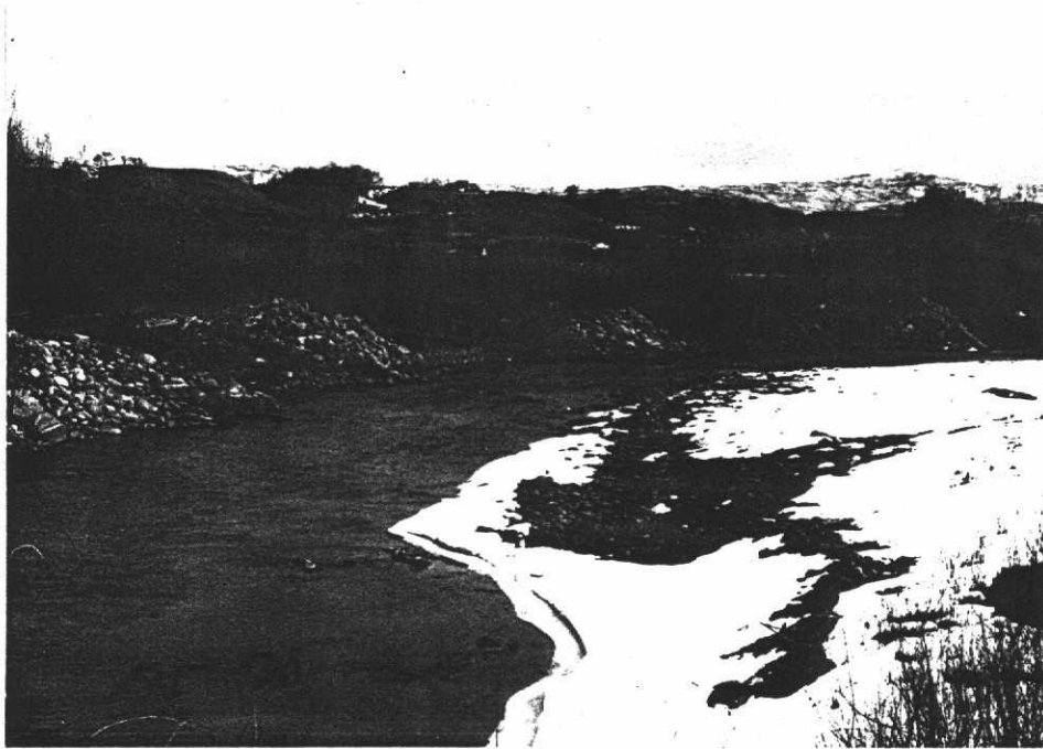
Right bank stabilization. Rock jetties placed in 100 foot intervals.
