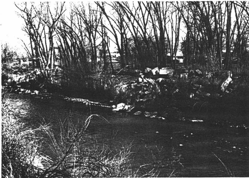
Rock jetties placed at 100 foot intervals in the 1930's.
