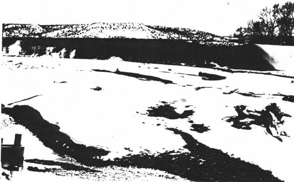
75 feet of Mesa land was eroded in 1983. The embankment is 40 feet high.
