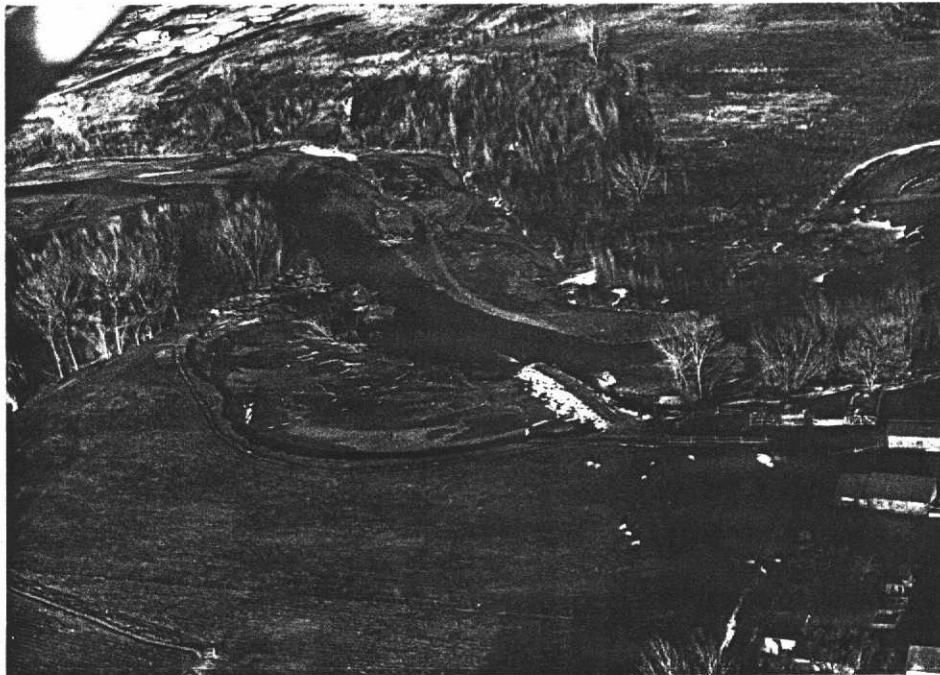
A rock jetty constructed to place channel in pre-flood alignment.
