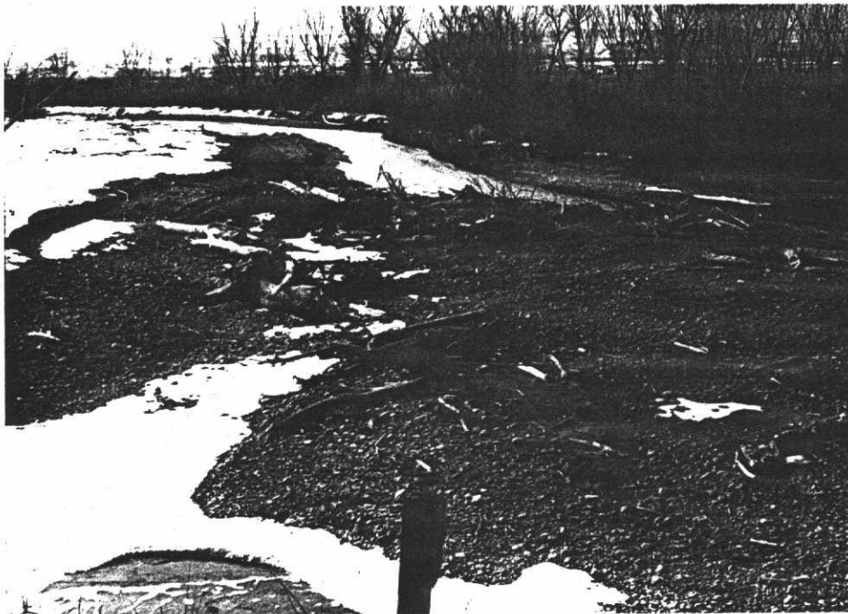
4 - 6 feet of sediment build-up completely clogging channel. Cobble size \frac{1}{2} " to 6".
