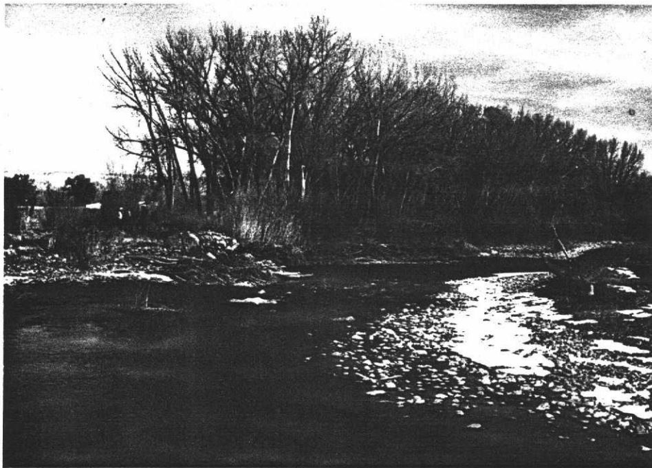
Upstream end of CC Camp project. Channel is eroding around the project.
