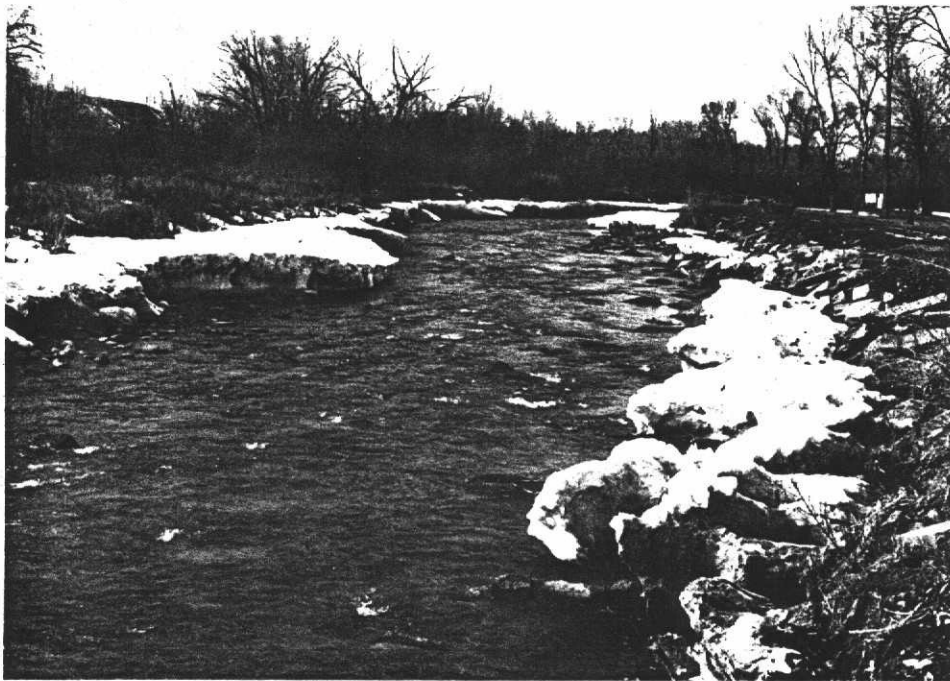
Channel stabilization by rip-rapping.
