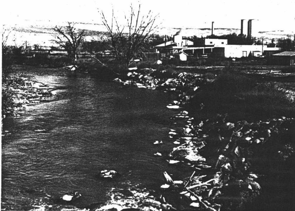
Right bank erosion - emergency repair during flood.
