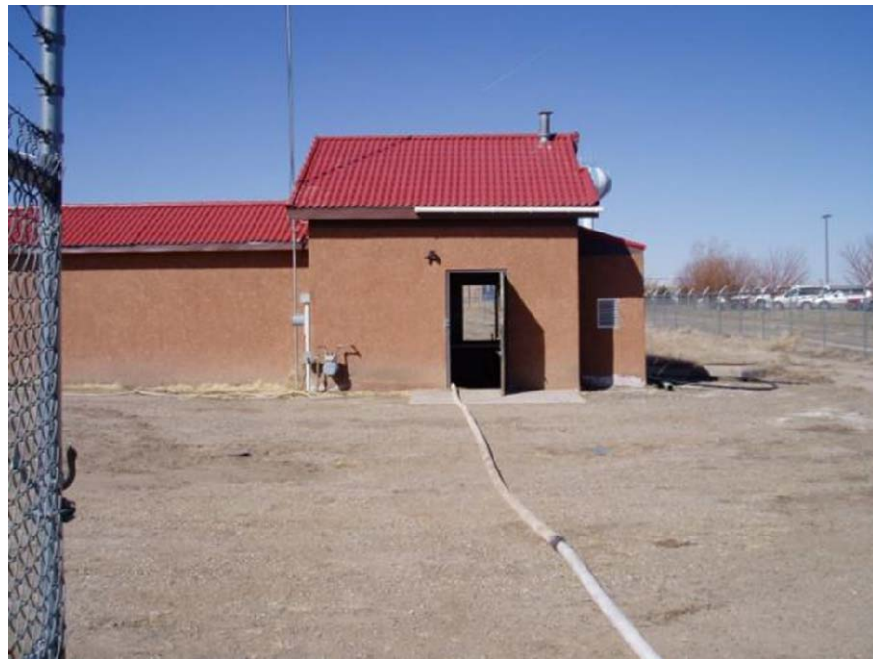
Photo 18: Crews used a mobile chlorination unit to disinfect the Weber Reservoir.
