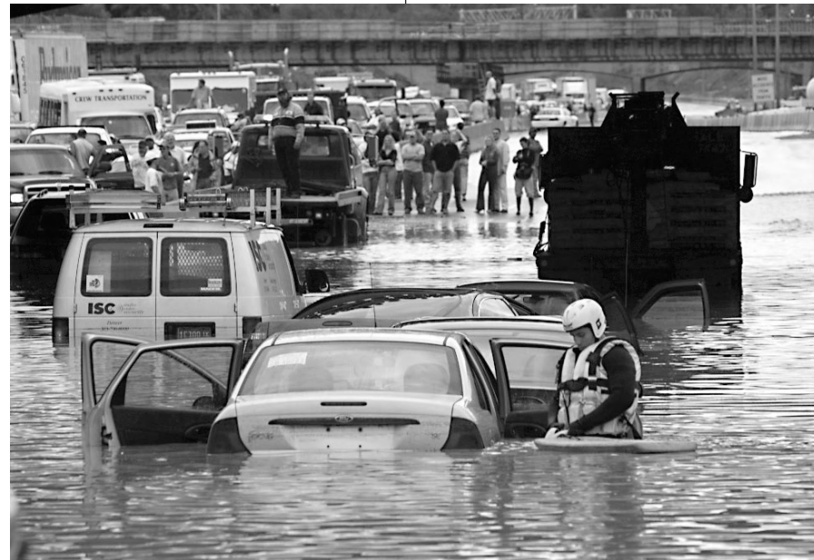
Drainage problems were frequent in the Narrows section of I-25 (Lake Logan, Sept. 13, 2002) prior to the completion of the new drainage system. Opposite: T-REX used a massive boring machine to drill the new drainage tunnel, replacing an inadequate drainage pipeline.
