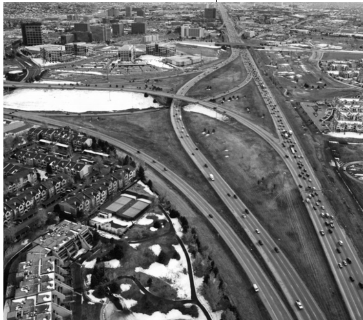
The I-25/I-225 interchange looking south in 2001, prior to the beginning of construction, with the left merge and exit ramp to northbound I-225.
