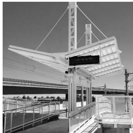
Nine Mile Light Rail Station Gull Wing style canopy.
