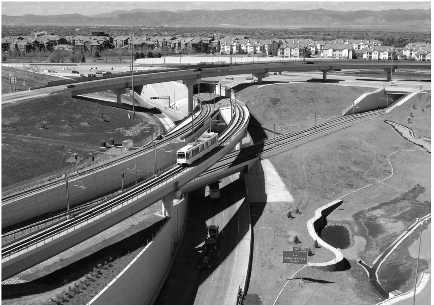
Light rail testing on the rebuilt I-25/I-225 interchange in 2006.
