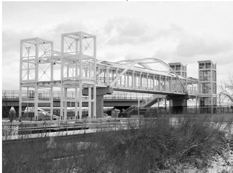
The Dayton Station is located adjacent to a sensitive wetlands area.
