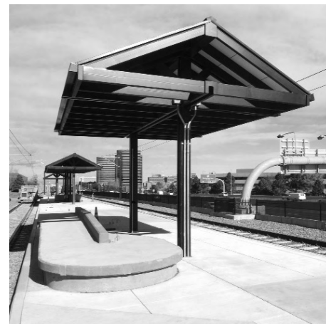
Orchard Light Rail Station Village style canopy.
