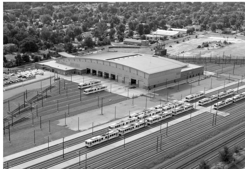
The Elati Light Rail Maintenance Facility was constructed along RTD's Southwest Corridor in Englewood at the former site of the General Iron Works.
