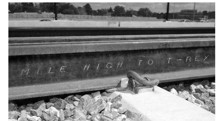
The steel used to manufacture the tracks was recycled from the former Mile High Stadium. Each section of rail along the project is inscribed with "Mile High to T-REX."
