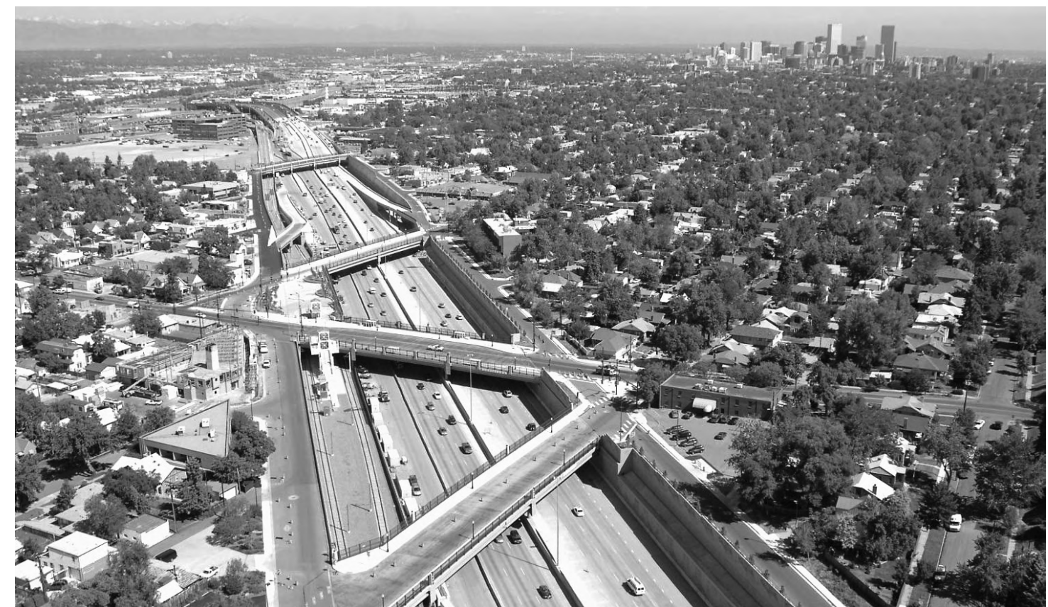
Most of the bridges in the Narrows were more than 50 years old prior to the construction of T-REX. All of the bridges in that area were reconstructed.
