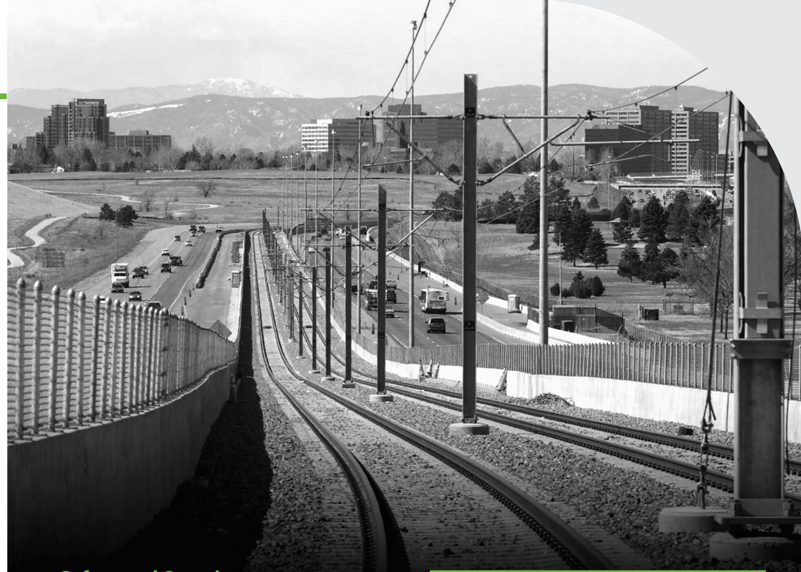
The light rail runs down the median on I-225, while staying on the west side of the highway along I-25.
