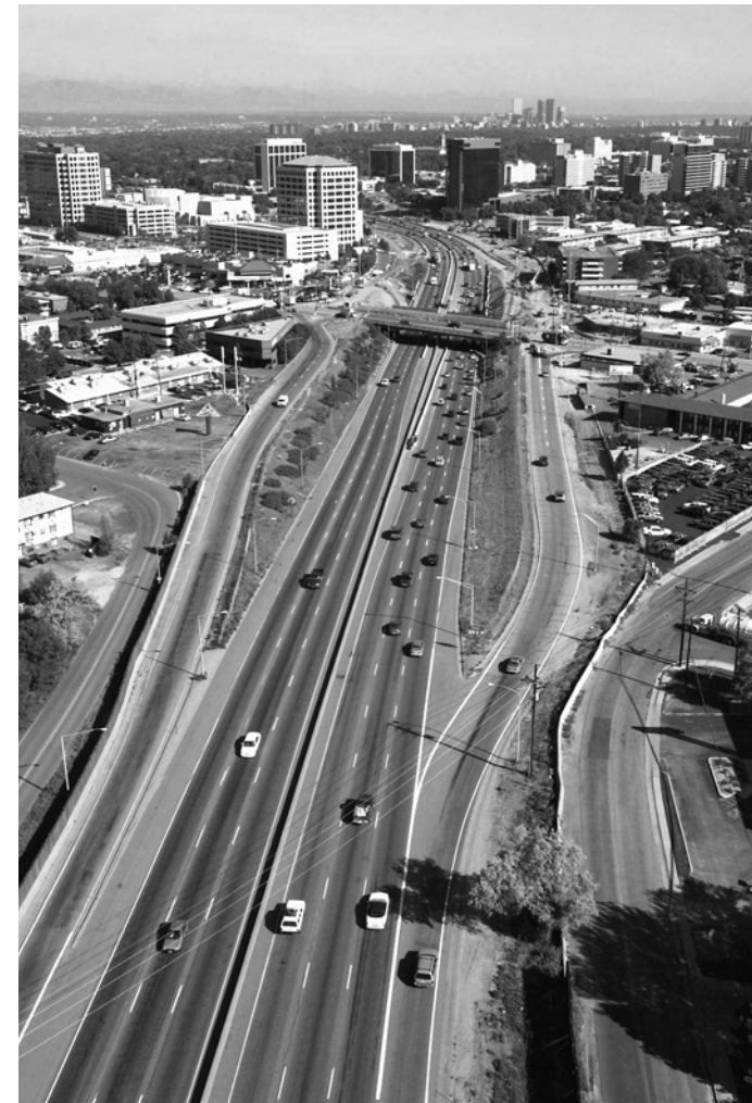
I-25 at Evans looking north in 2001, before the start of construction.
