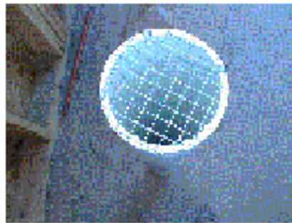
¼ inch rodent screen on discharge
