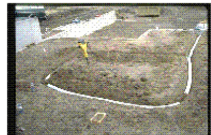
Photo of pipe being laid in trench
