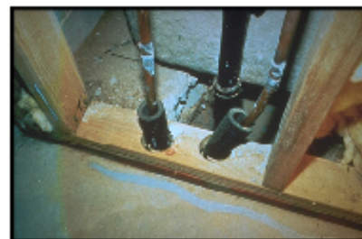
Plumbing penetrations through plates
