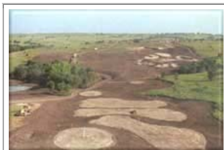
The construction of Colbert Hills Golf Course near Manhattan, Kansas.
