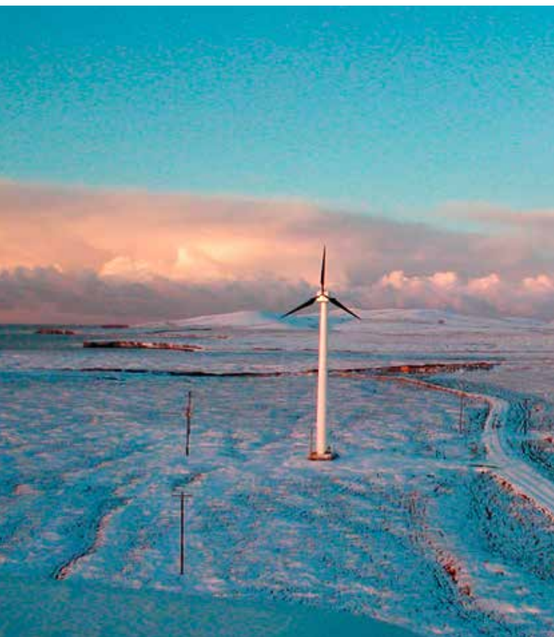
Figure 7.4. Snow and other winter weather conditions can negatively affect wind turbine operations (NorthWind 100 turbine in Toksook Bay, Alaska. Photo: National Renewable Energy Laboratory).
