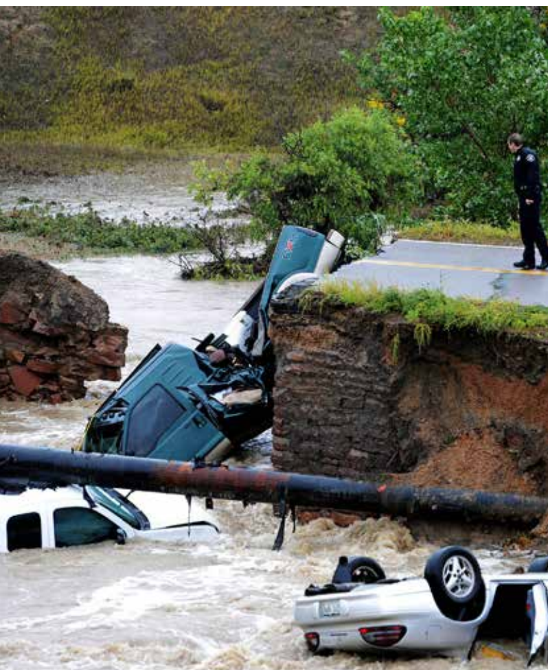
Figure 8.3. Cars plunged into Rock Creek when Dillon Road collapsed near Broomfield during the September 2013 Front Range floods (Photo: Cliff Grassmick, Boulder Daily Camera).
