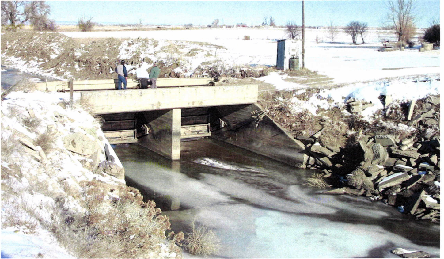
Photo 3 - Lake Lee Dam - Downstream
