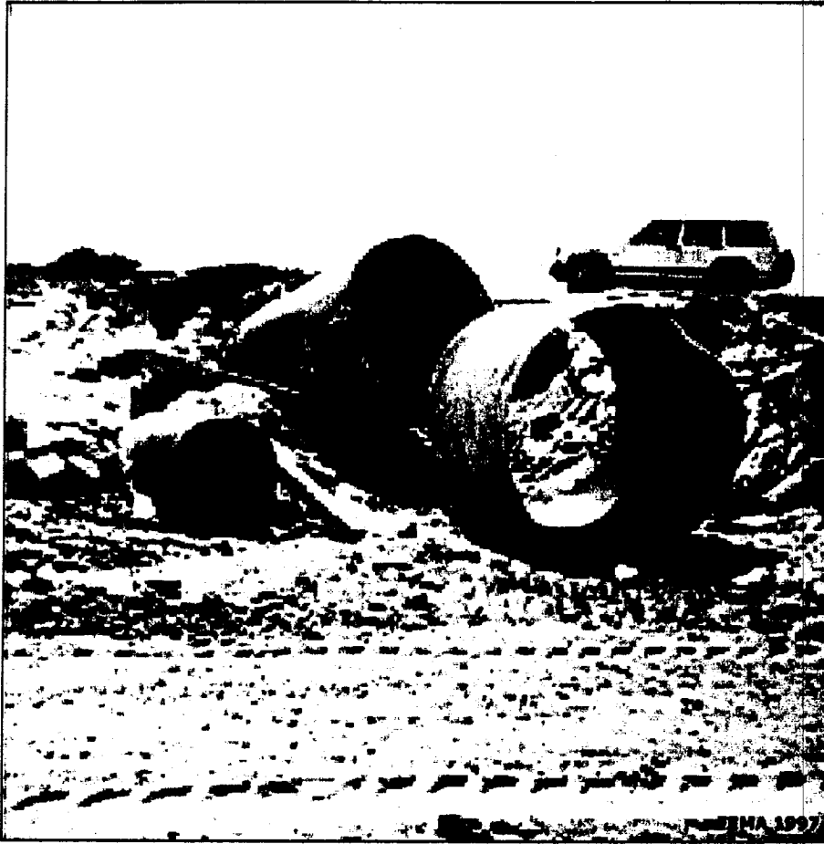
Figure 4.5-6 Damaged Culvert Under County Road L in Western Kiowa County
