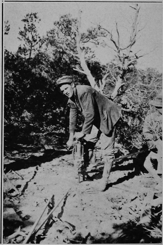
Fig. 40. Prospecting for ore in Long Park by means of a jackhammer.
