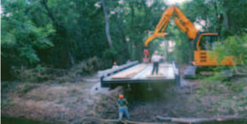
Figure 4-16. Example of a modular bridge with running planks. Photo: Big R Bridge
