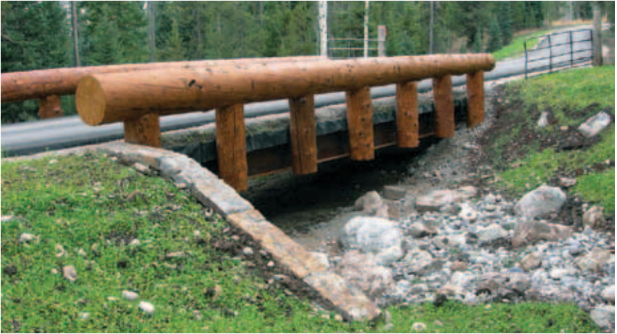
Figure 4-12. Modular bridge with log railing. Photo: Big R Bridge
