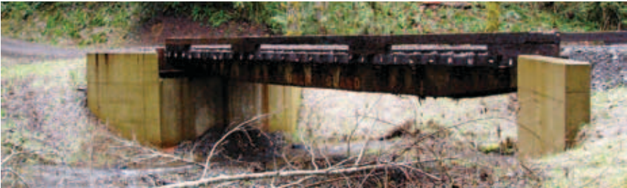
Figure 4-17. Example of a railroad car bridge with concrete abutments.
