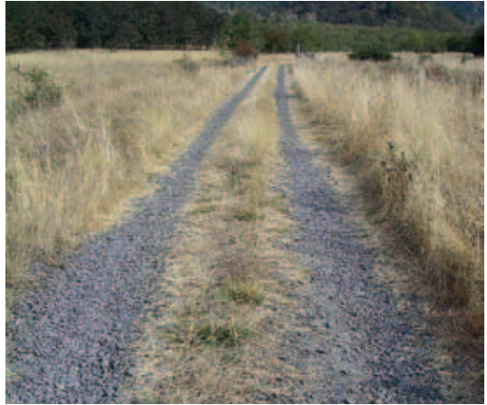
Figure 1-16. Example of low-usage road illustrating fire hazard and vegetation issues.
