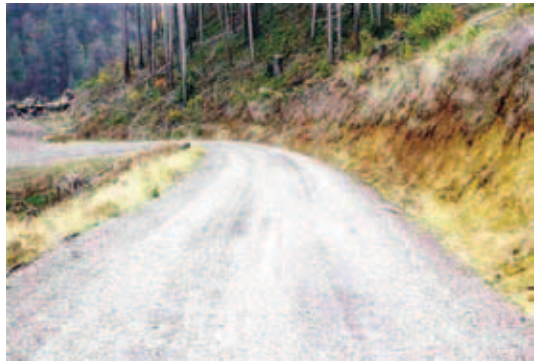
Figure 5-17. Example of road segment with proper water diversion and dissipation methods.
