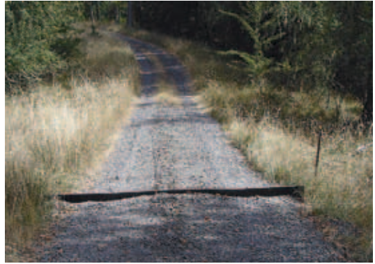
Figure 3-18. Example of an in-place rubber waterbar.
