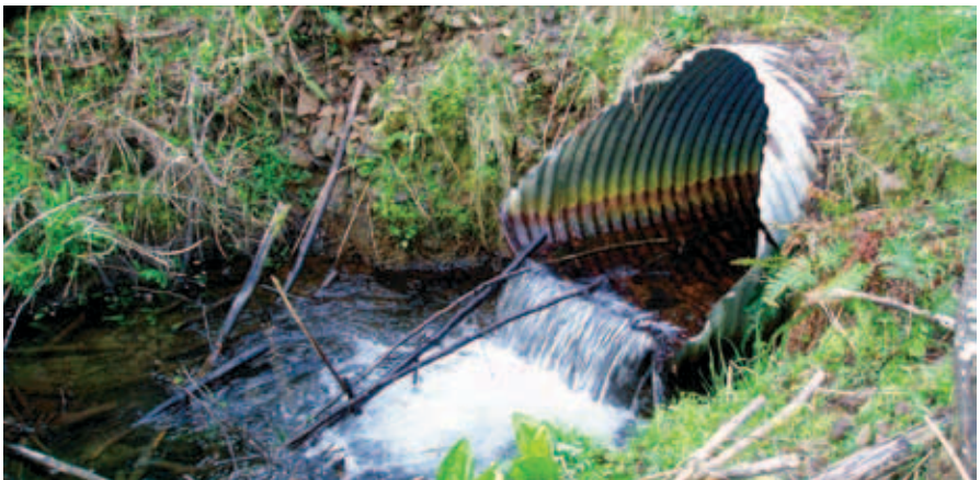
Figure 5-45. Stream crossing with reasonable jump height and stream velocity.
