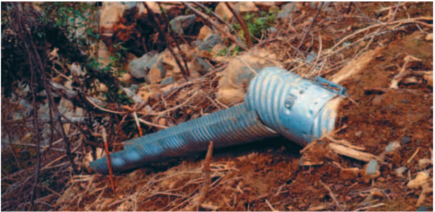
Figure 3-10. Example of a culvert half-round dissipater.
