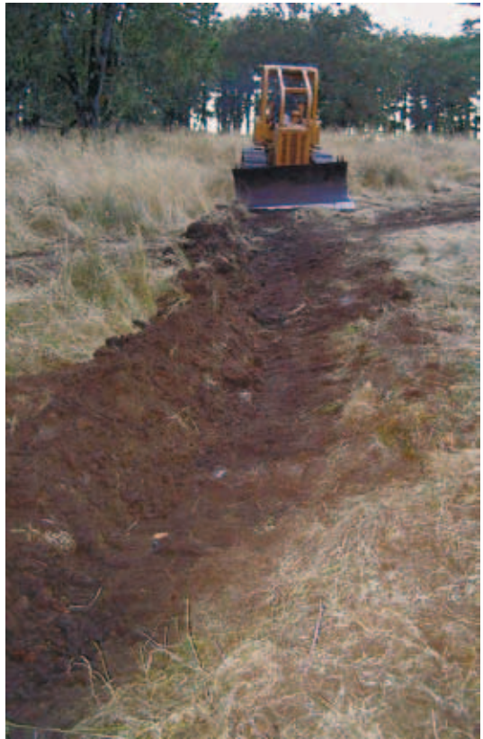
Figure 5-32. Example of waterbar being constructed on a low-use unimproved surface road.
