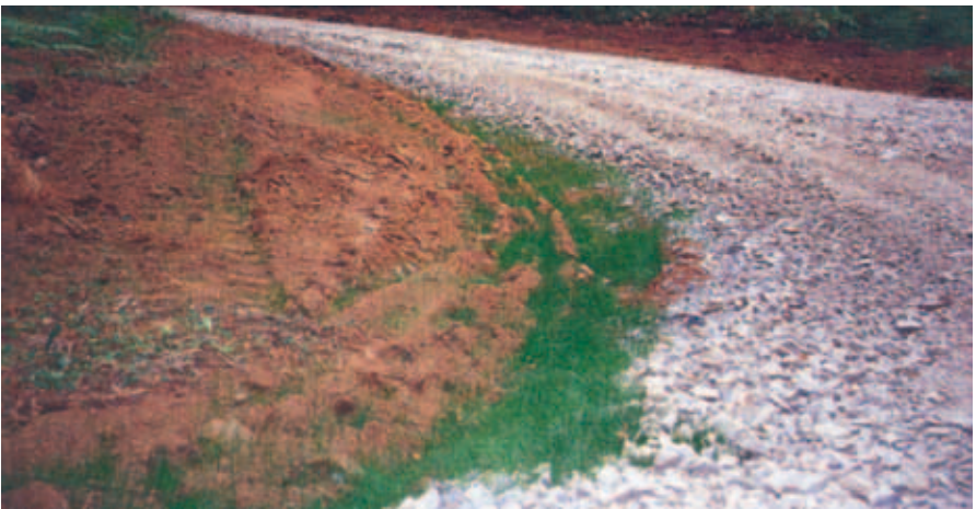
Figure 3-13. A properly functioning vegetated ditch.
