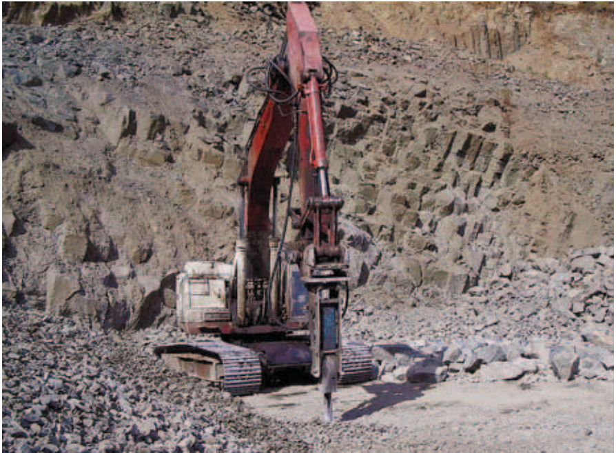
Figure 6-31. An excavator with a hydraulic rock breaker.
