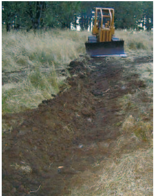
Figures 3-23 and 3-24. Bulldozer installing waterbars on unimproved surfaces.
