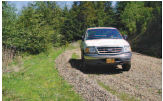
Figure 5-49. An improved road with aggregate berm.
