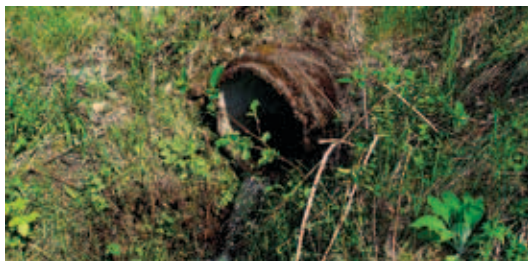
Figure 5-55. Concrete culvert; low priority.
