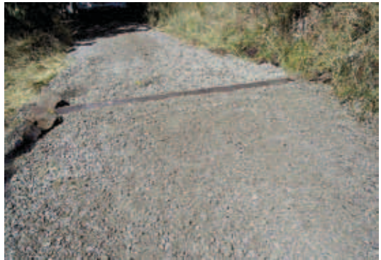
Figure 5-33. An example of how to make a conventional waterbar a bit more user friendly.
