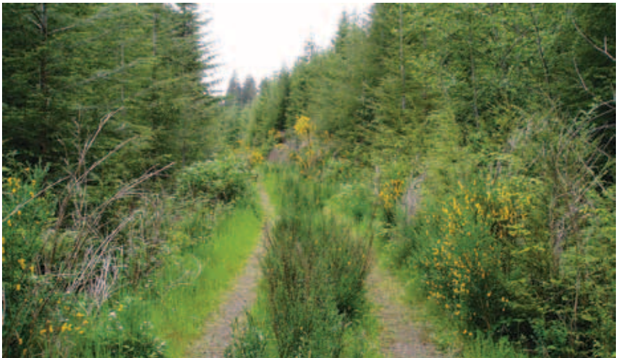
Figure 5-30. Brush and vegetation on the road can become a maintenance issue.
