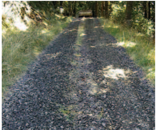
Figure 1-17. Example of a low-usage road after spot-rocking and track-spreading.
