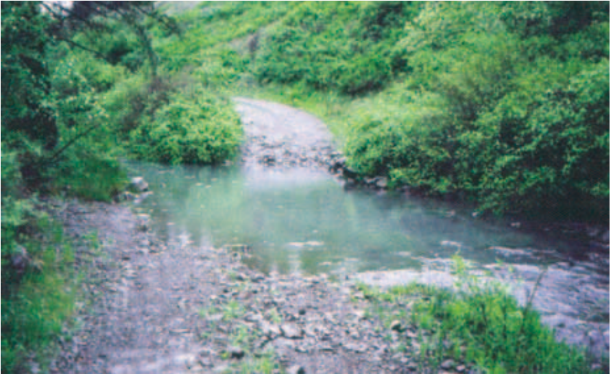
Figure 4-8. Example of a low-traffic ford crossing.
