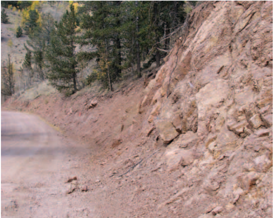
Figure 5-27. Cut-slope erosion example 2. Photo: R.M. Edwards
