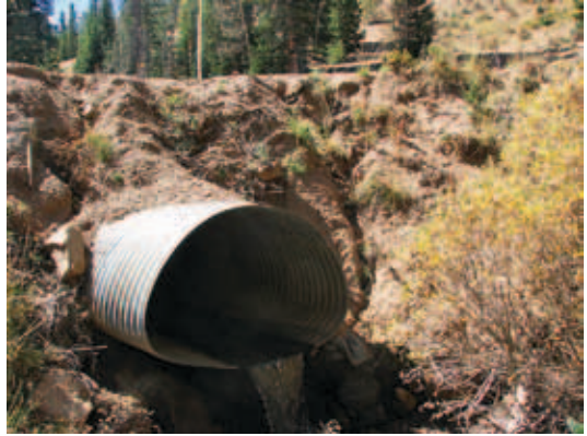
Figure 4-6. Culvert example 3. Photo: R.M. Edwards
