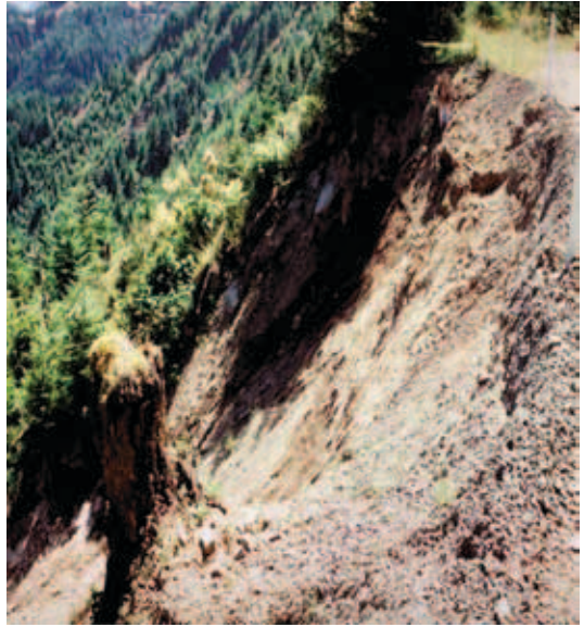
Figure 5-15. Example of slope failure.
