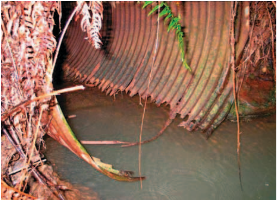
Figure 5-37. Rusted culvert.
