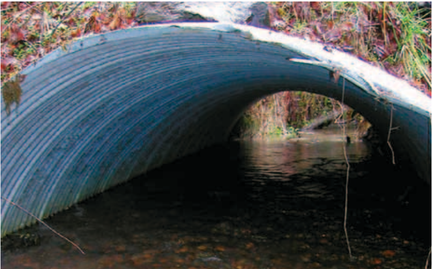
Figure 4-13. Bottomless arch culvert.
