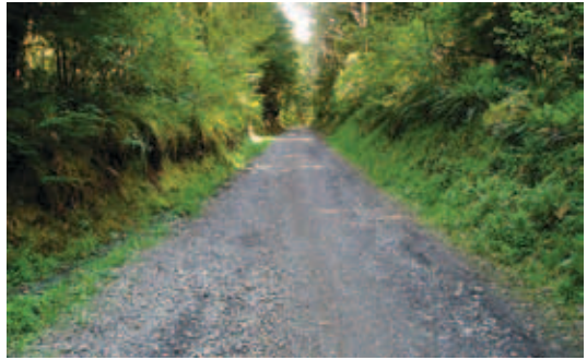
Figure 5-31. Example of an improved, through-cut road that may require waterbars.
