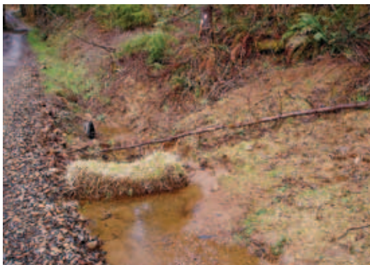
Figure 6-24. Use of hay bales for capturing sediment.
