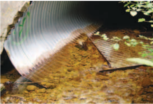
Figure 4-9. Example of an arch culvert with baffles.
