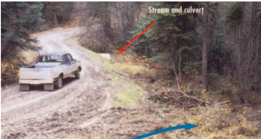
Figure 6-20. Routing ditch drainage through a filtering of undisturbed vegetation so sediment can be removed before water reaches the stream.
