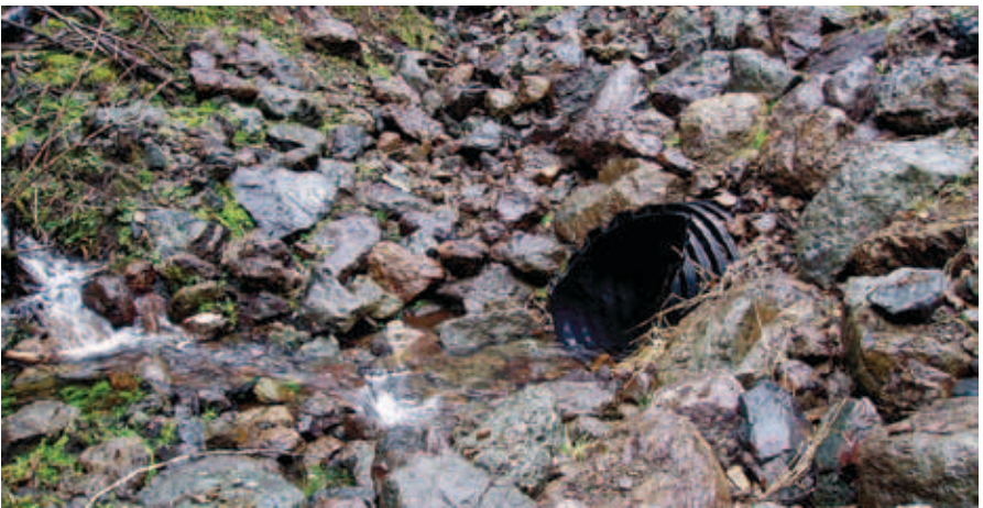
Figure 4-20. Culvert with armoring.
