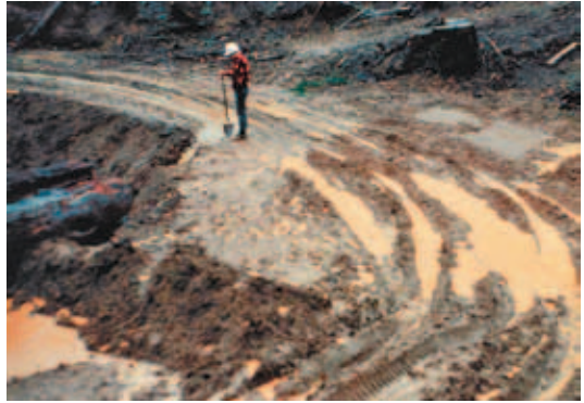
Figure 6-17. Wet-weather hauling on an unimproved surface road.
