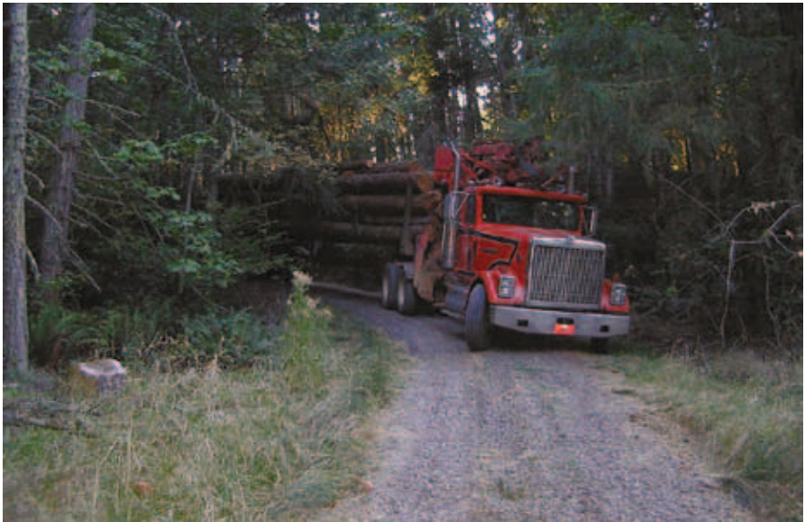
Figure 5-20. A poorly designed forest road in terms of clearance.
