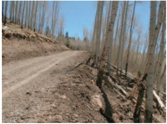
Figure 1-5. Example of an outsloped road.
