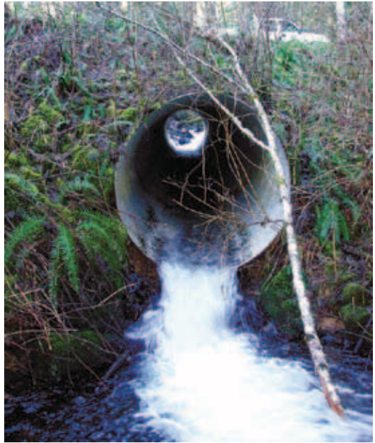
Figure 5-44. Stream crossing with excessive jump height and stream velocity.
