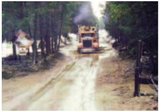
Figure 6-18. Wet-weather hauling on an improved surface road.
