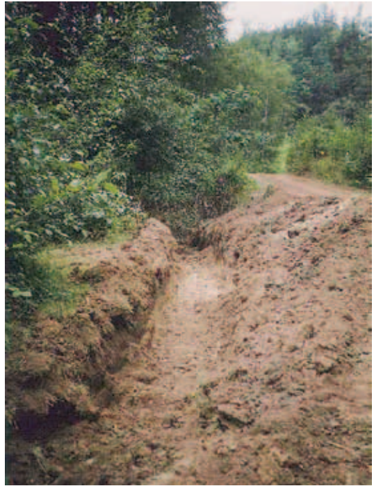
Figure 1-9. A soil trench barring entrance on unimproved road surface.
