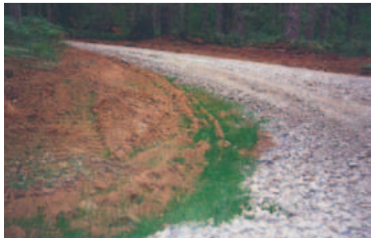
Figure 1-10. Improved road surface with off-site aggregates.
