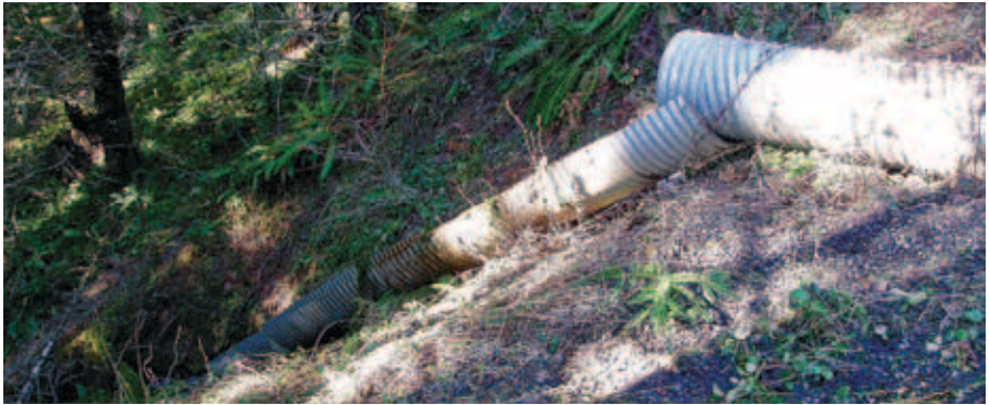
Figure 5-41. Prevention of downslope erosion utilizing steel half-round pipe.
