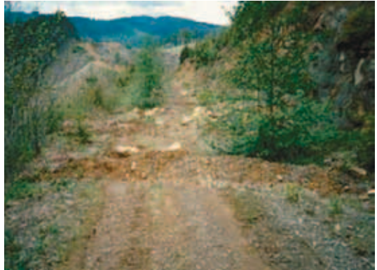
Figure 3-14. Example of an unimproved road with a waterbar.
