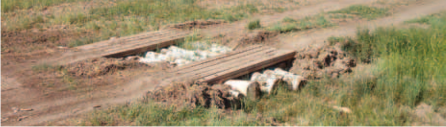
Figure 4-14. Example of low-tech solution for a temporary crossing using logs and lumber. Photo: Kelly Rogers
