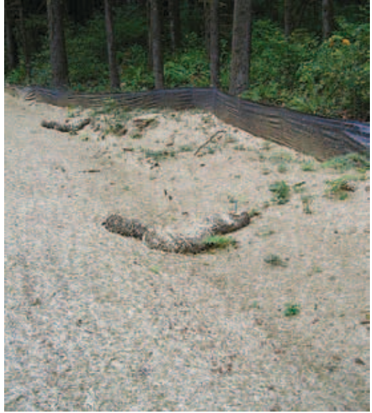
Figure 6-21. Use of slope-armoring as a filtering system.
