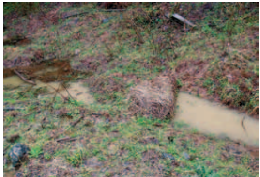
Figure 5-47. Illustration of permanent road structures as part of the sediment filtering system.
