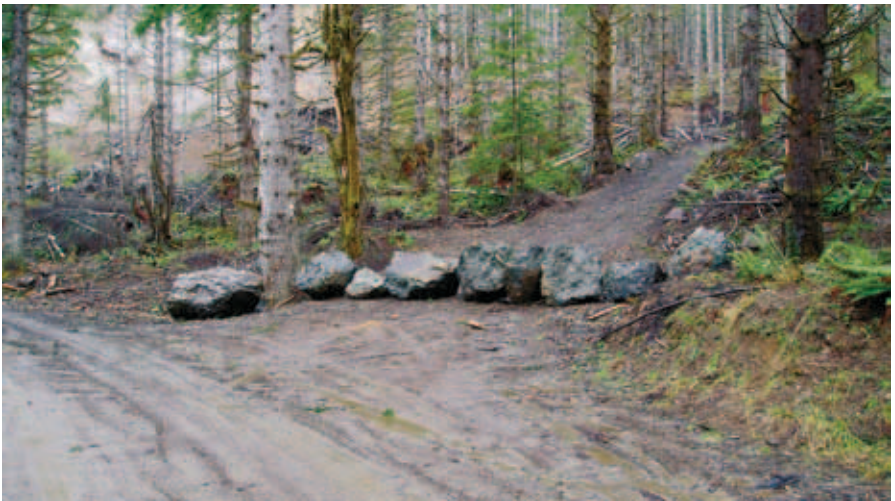
Figure 5-16. Temporary road closure.
