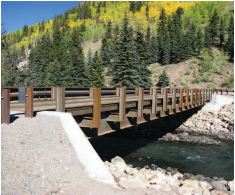
Photo: Big R Bridge
