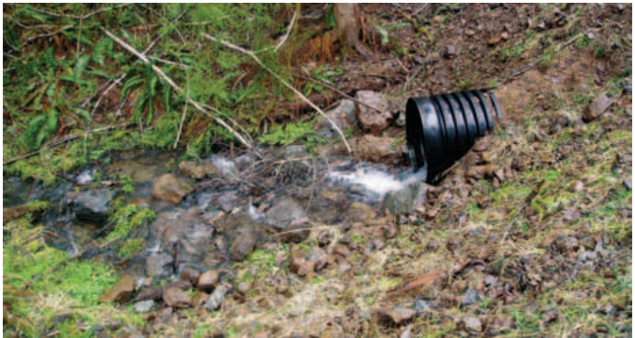
Figure 3-2. Example of a drainage culvert.
