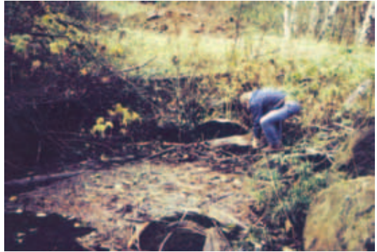
Figure 5-3. Preferred inspection method: inspect end of culvert prior to wet weather or heavy use.
