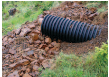
Figure 5-43. Prevention of downslope erosion with rip-rap.
