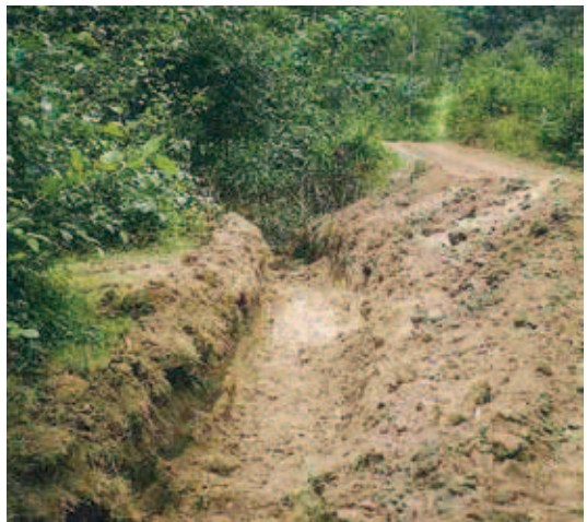
Figure 6-28. A road closure using deep ditches.
