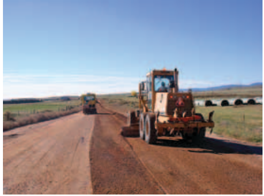
Figure 5-53. Preparation of road surface prior to dust-suppressant application.
