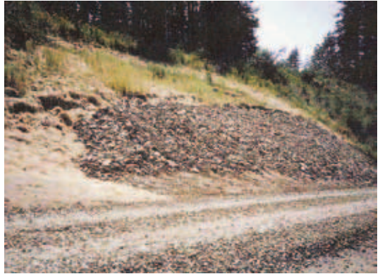
Figure 5-28. Example of cut-bank armoring.
