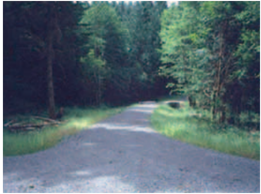
Figure 5-19. A well-designed forest road with adequate clearance.
