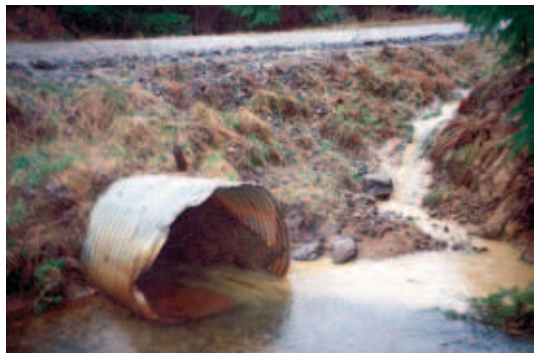
Figure 6-15. Example of ditch-relief structure sediment delivery.
