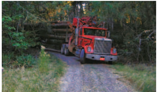
Figure 1-20. A horizontal curve with insufficient width for off-tracking with log trucks.
