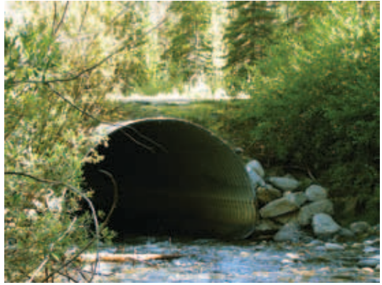
Figure 4-4. Culvert example 1. Photo: R.M. Edwards
