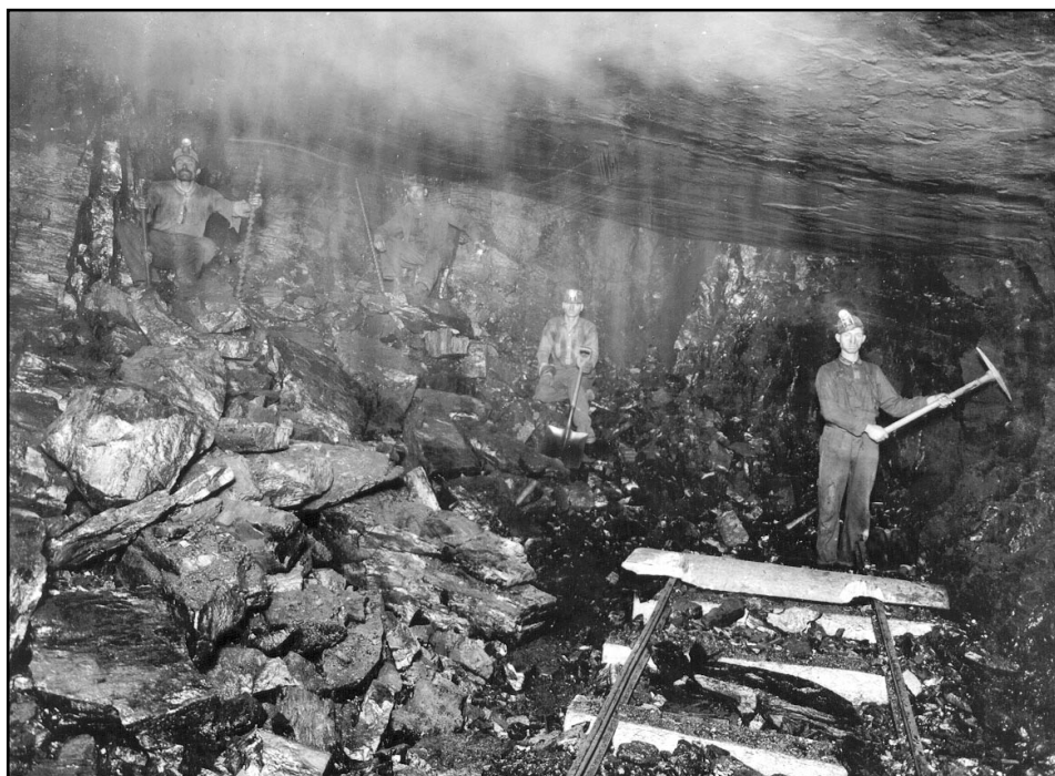
Figure 8. Pickers and Diggers after blasting coal in mine around early 1900s. Smoke on roof is from the blast. Mine name is unknown. (Photo courtesy of the Colorado Historical Society)
