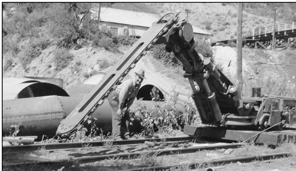
Figure 11. 1937—First hydraulic cutting machine, Sullivan 7AU with approximately a 9 ft blade. Man in photo is Wallace Bowie. (Photo courtesy of Robert Bowie).
