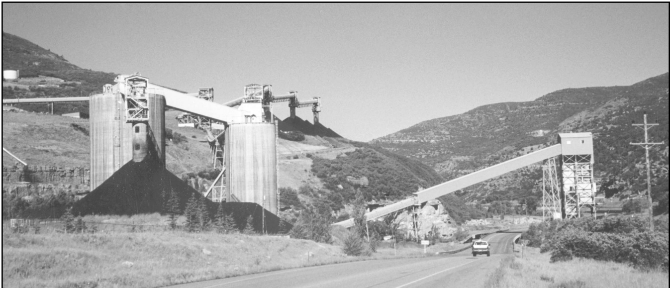
Figure 13. View from Highway 133 of the Union Pacific rail load-out (on right), storage silos and stack tubes (on left) of the West Elk Mine, Somerset Coal Field
